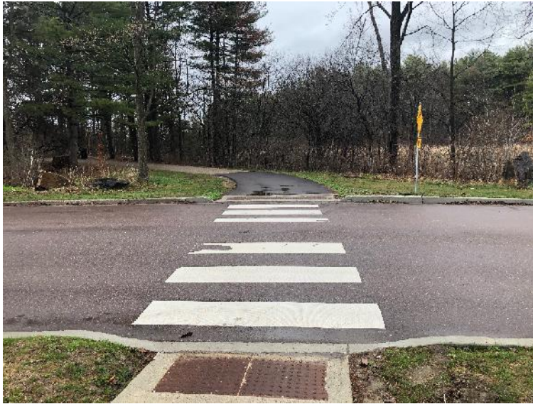
Entrance to Greenway from Austin Dr. looking north
