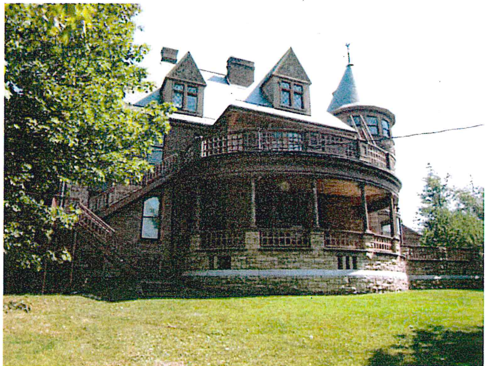
West Elevation, from the north
