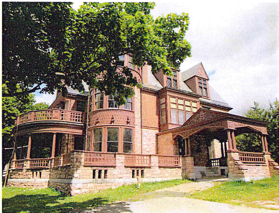
View from the Southwest
