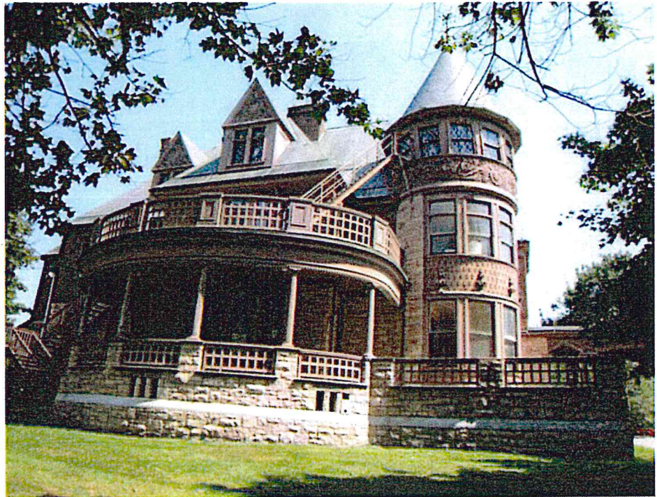
West Elevation, from the south
