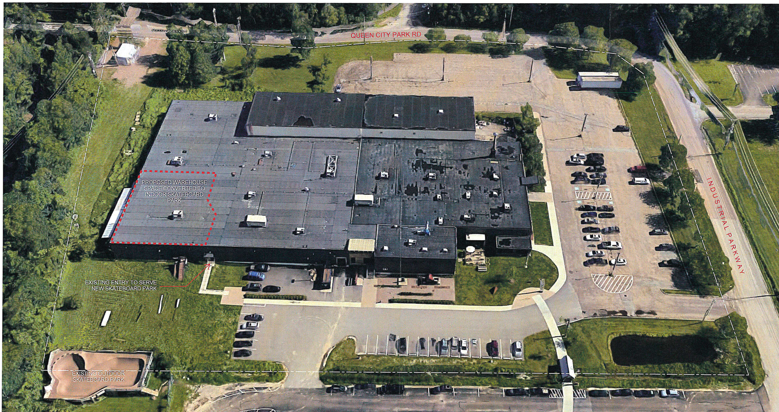
152 INDUSTRIAL PARKWAY AERIAL PHOTO FROM NORTH (THERE ARE NO PROPOSED CHANGES TO THE EXTERIOR)
