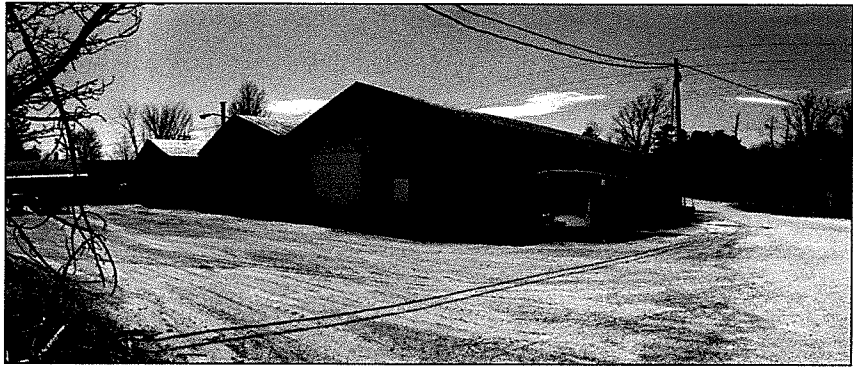
VIEW: EAST FACADE FROM BRIGGS STREET (Buildings 7&8)
