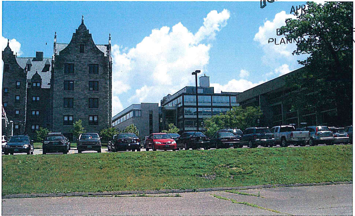
5. View just east of the project area looking toward Converse Hall (left), Given Hall (center) and Rowell Hall (right).
