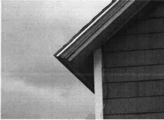
89. The molded cornice appears to be historic.
