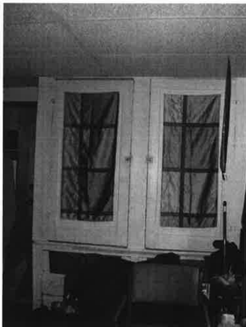
22. The front units on both floors retain historic kitchen cabinets; note modern ceiling tiles.
