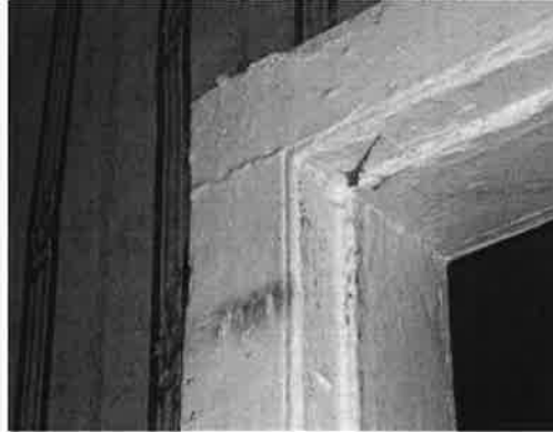
72. & 73. Typical views of window (left) and interior door trim (right). Note the many layers of paint.
