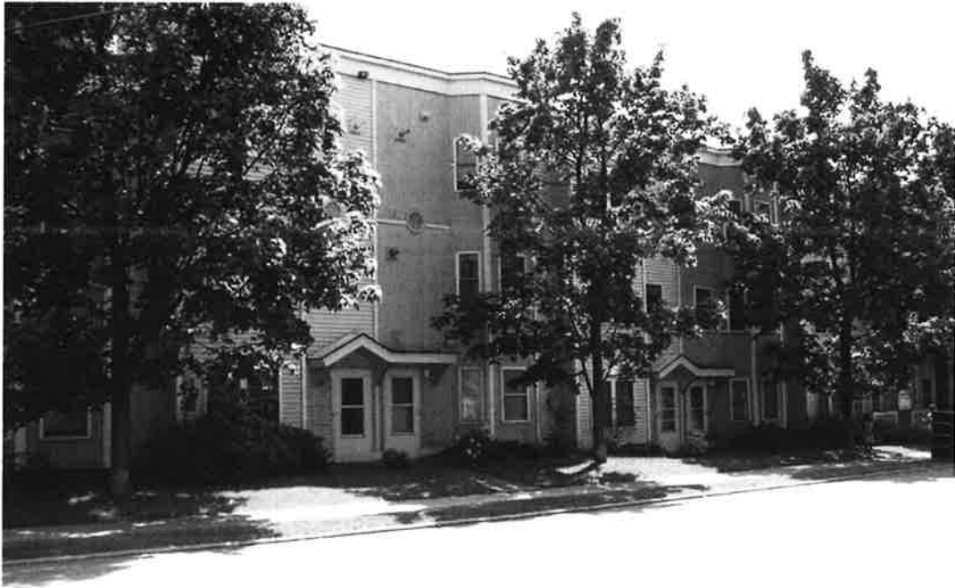
5. Context view looking southwest from 114 Archibald Street toward large, modern, 3-story apartment house.
