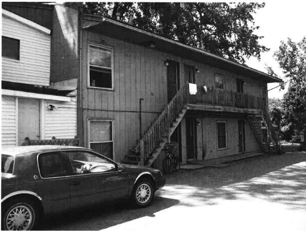
14. View of modern rear addition looking northwest.
