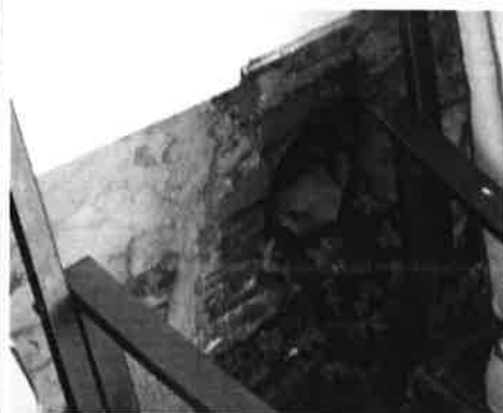
45. (Right) former clean-out remains in the foundation for a chimney on the north elevation that has been removed.
