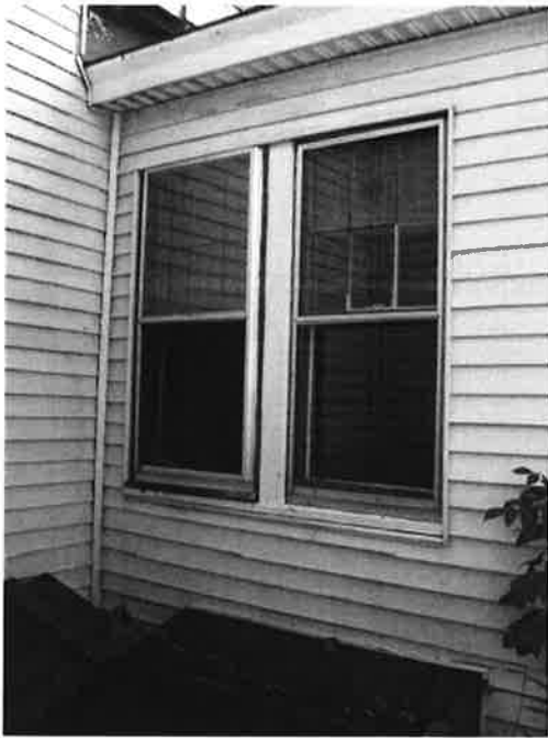
13. Two historic six-over-one windows on the east elevation.
