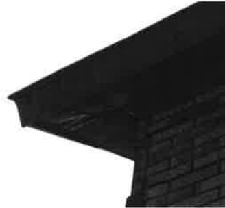
48. & 49. Details of the replacement box cornice on both the rear ell and main block.
