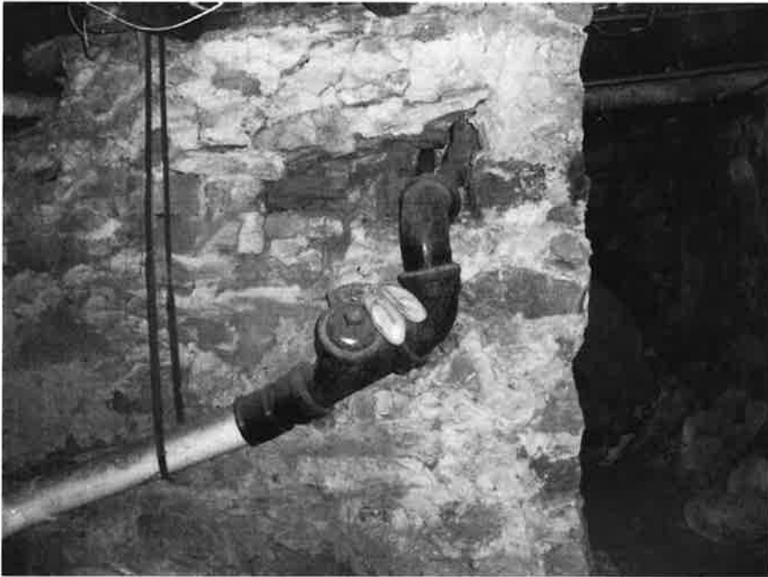
99. The stone foundation in the basement.
