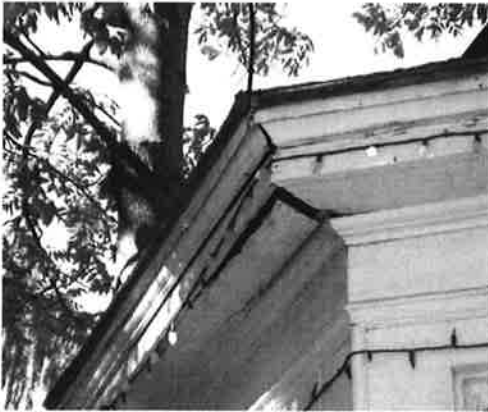
53. (Left) The bay window cornice is in poor condition in many areas such as above.
