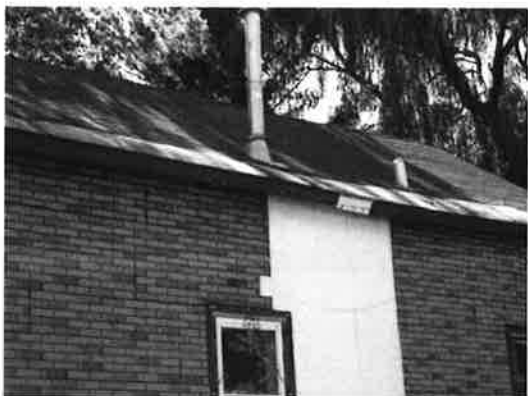
44. (Left) North roof slope has a significant sag.
