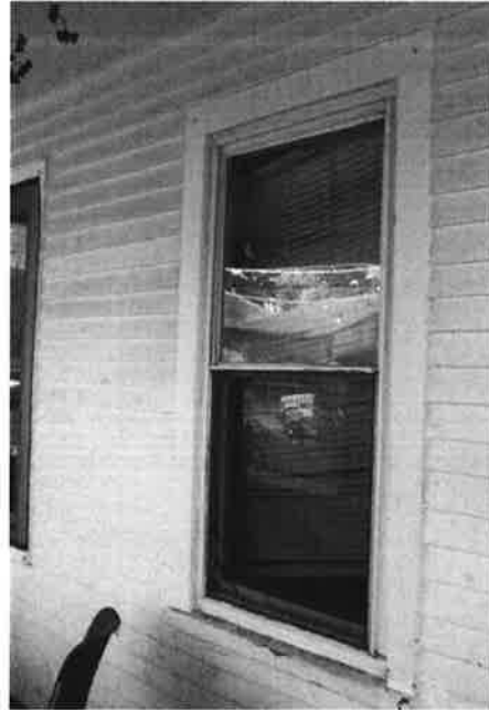
56. Vinyl windows and wood clapboards at front porch.
