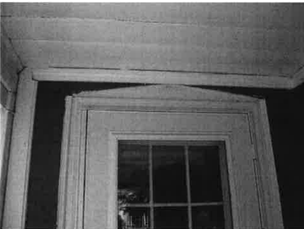
92. Remnants of older door trim including a peaked lintel remain in a modified opening with a new door.
