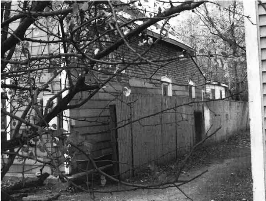
86. North elevation showing asphalt siding under asbestos siding. Peaked window lintels may be historic.
