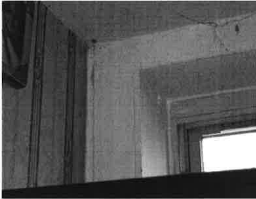
72. & 73. Typical views of window (left) and interior door trim (right). Note the many layers of paint.
