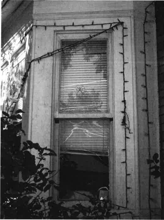
52. The bay window front elevation looking west.
