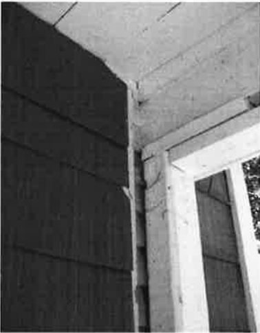
90. & 91. Front porch ceiling and frieze band appears old; other elements including posts are new.
