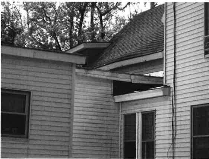
12. Detail of east elevation; note bowed roof at eaves and variety of adjacent roof slopes.
