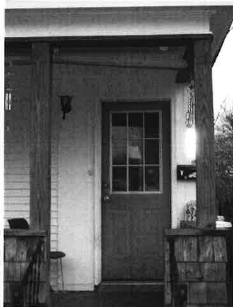
40. & 41. View of porch with detail of front entry showing historic porch cornice, clapboards and remains of an early door surround. Also note replacement flat trim at raking cornice of main block above, replacement porch posts and entry door within a partially infilled historic door opening.
