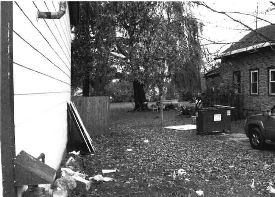
36. View of site between the white shed and 39 Bright Street, showing the depth of the parcel.
