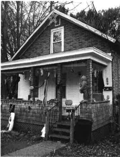
40. & 41. View of porch with detail of front entry showing historic porch cornice, clapboards and remains of an early door surround. Also note replacement flat trim at raking cornice of main block above, replacement porch posts and entry door within a partially infilled historic door opening.
