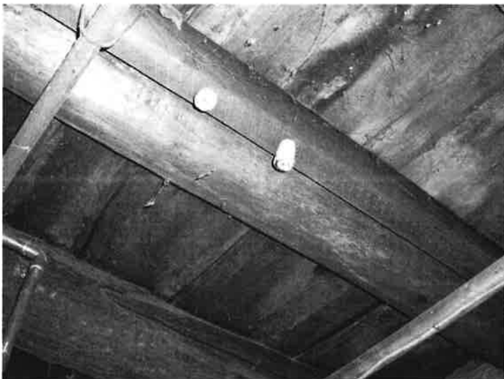
63. Framing in the basement reveals original joists with later sistered lumber.
