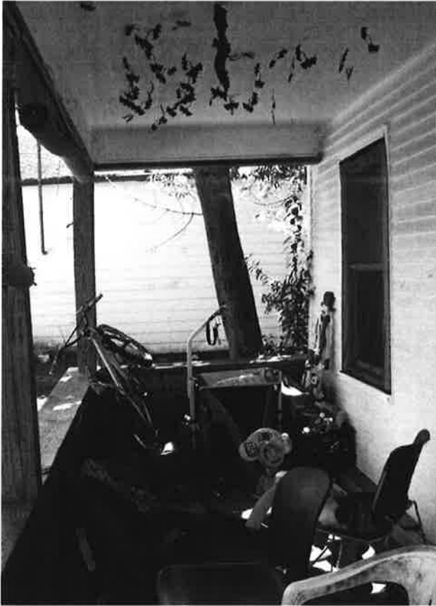
55. Front porch looking south.
