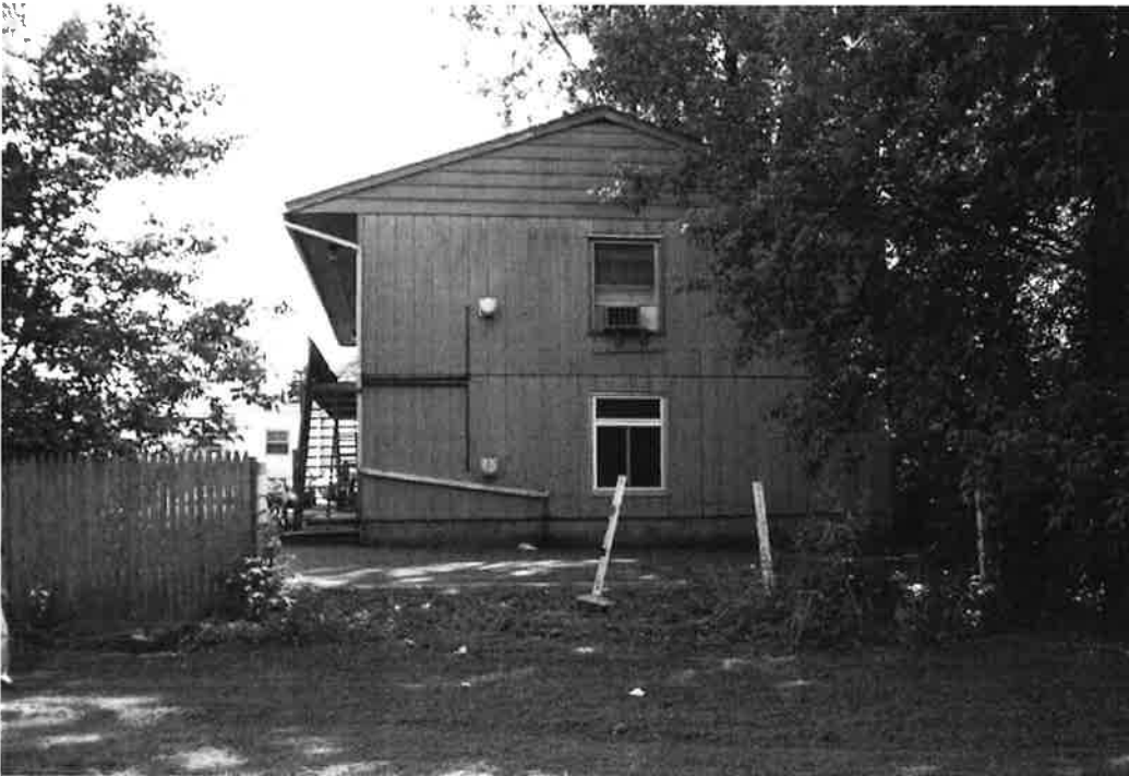
16. Rear (north) elevation of the modern rear addition.
