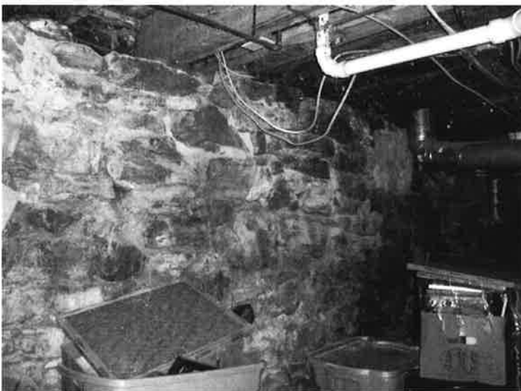
64. The stone and concrete basement foundation.
