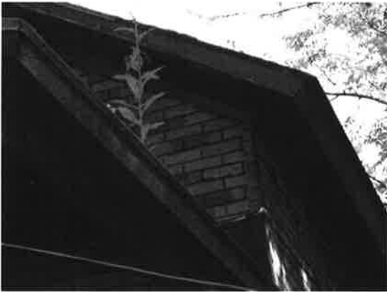
48. & 49. Details of the replacement box cornice on both the rear ell and main block.
