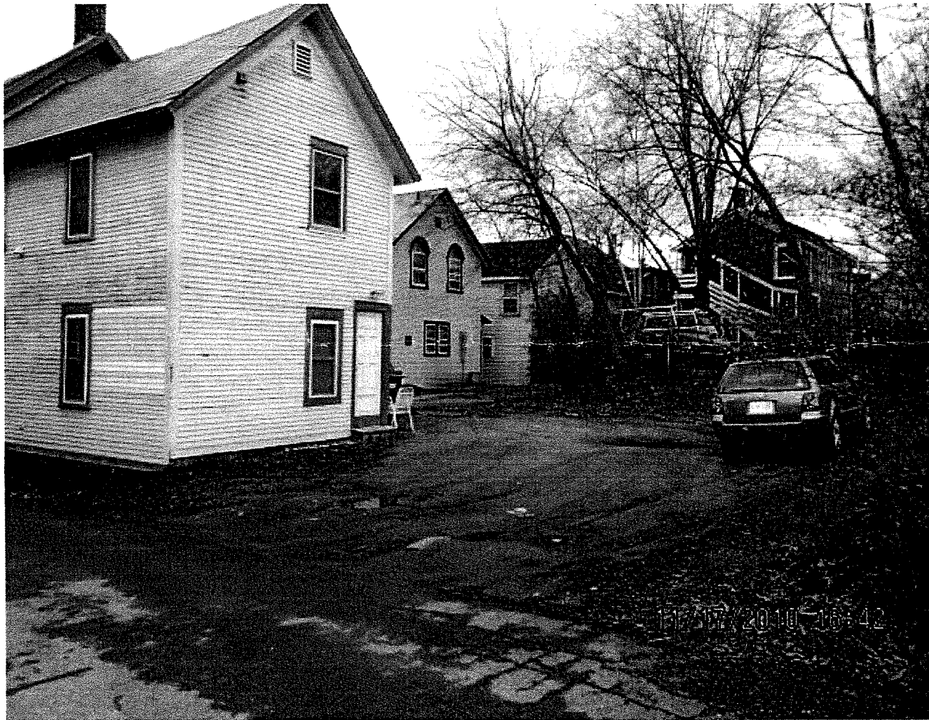
2010 Photo of rear yard. No gravel. No fence on southern boundary. Car is parked at a different angle than that shown in the 2004 Aerial Image.
