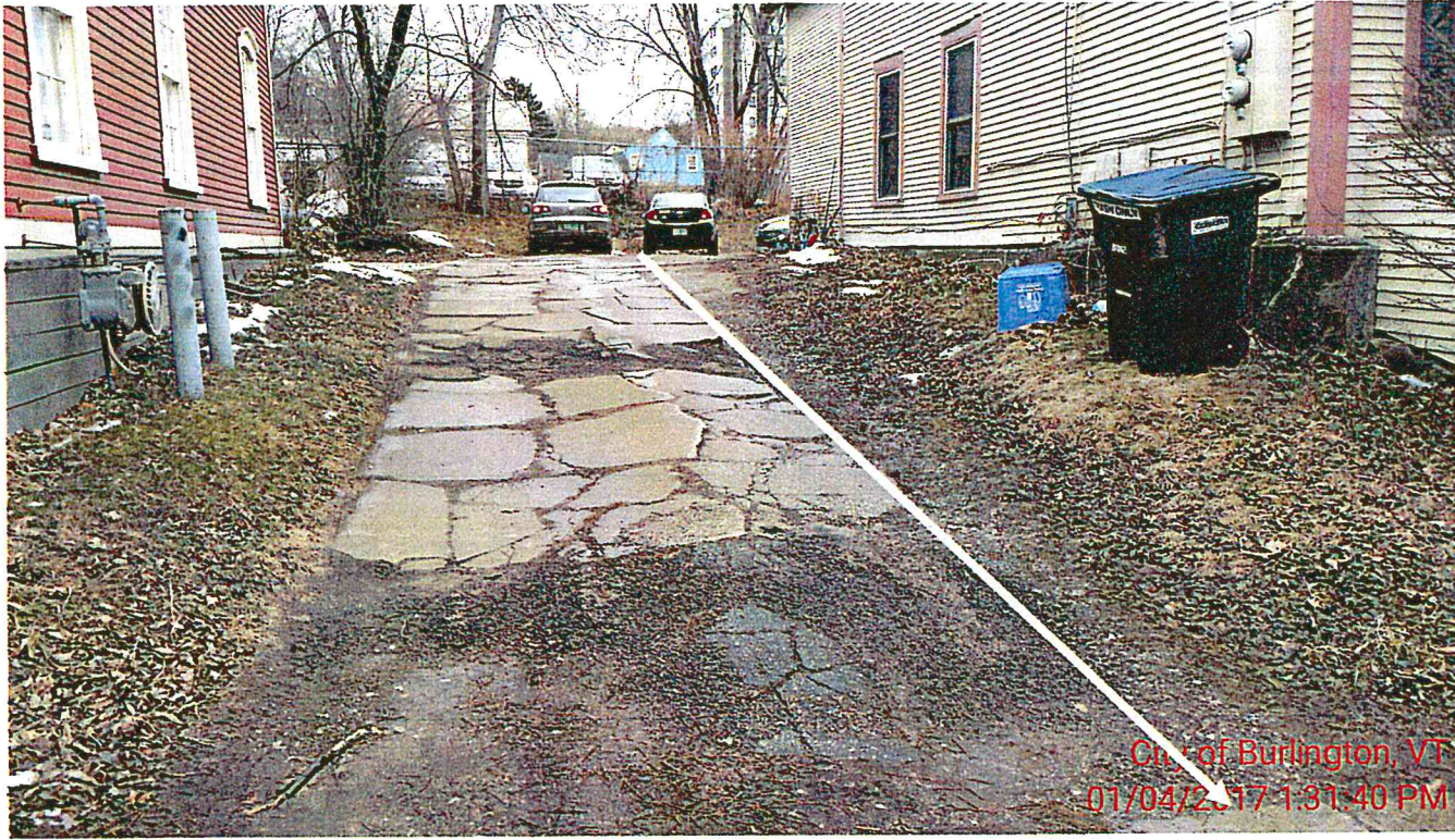
South of driveway widened.
