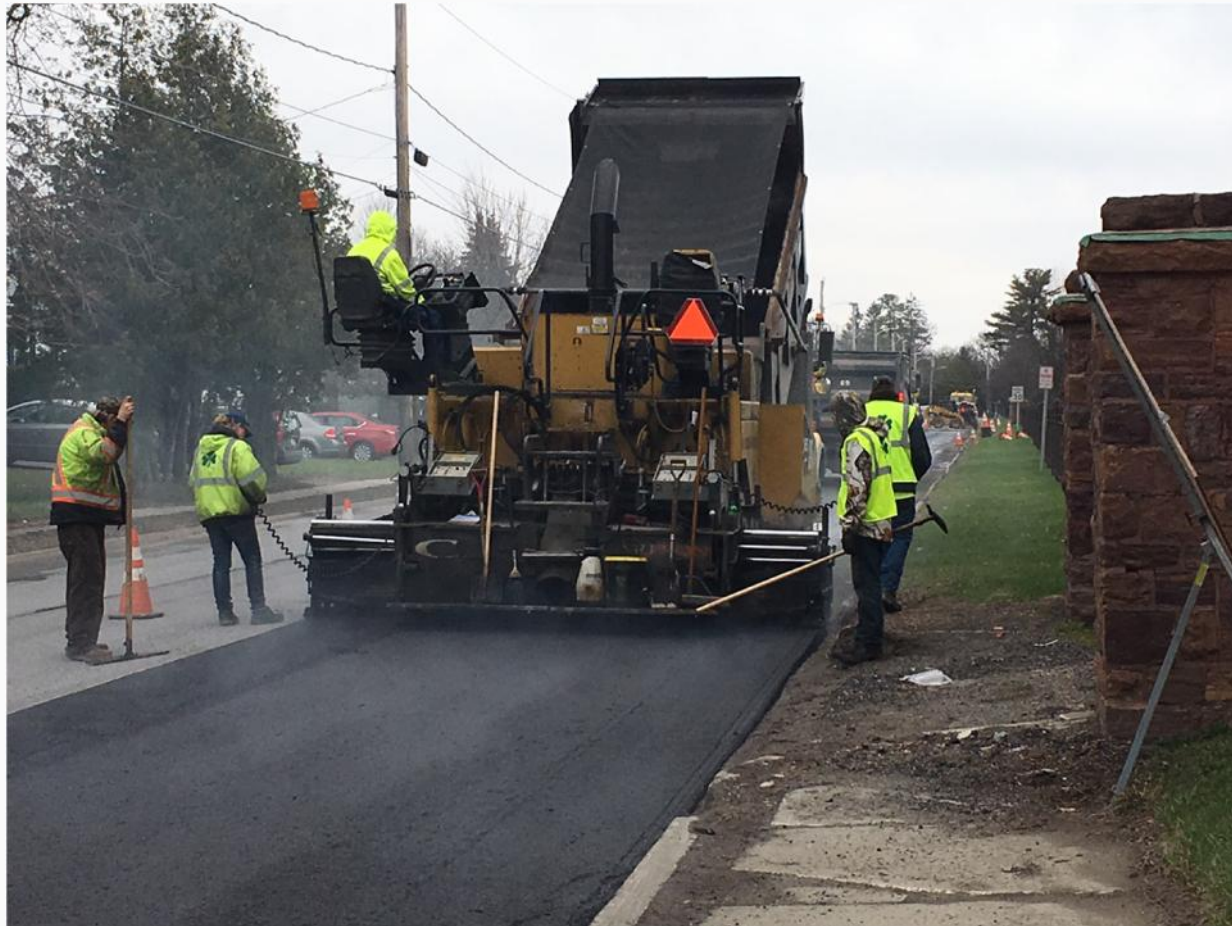
PLATTSBURG AVE PAVING, 4/27
