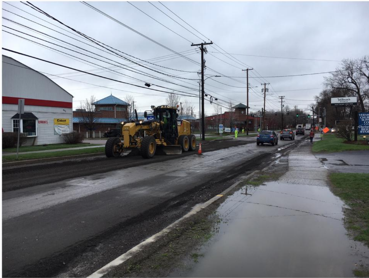
PINE ST GRADING, 4/30
