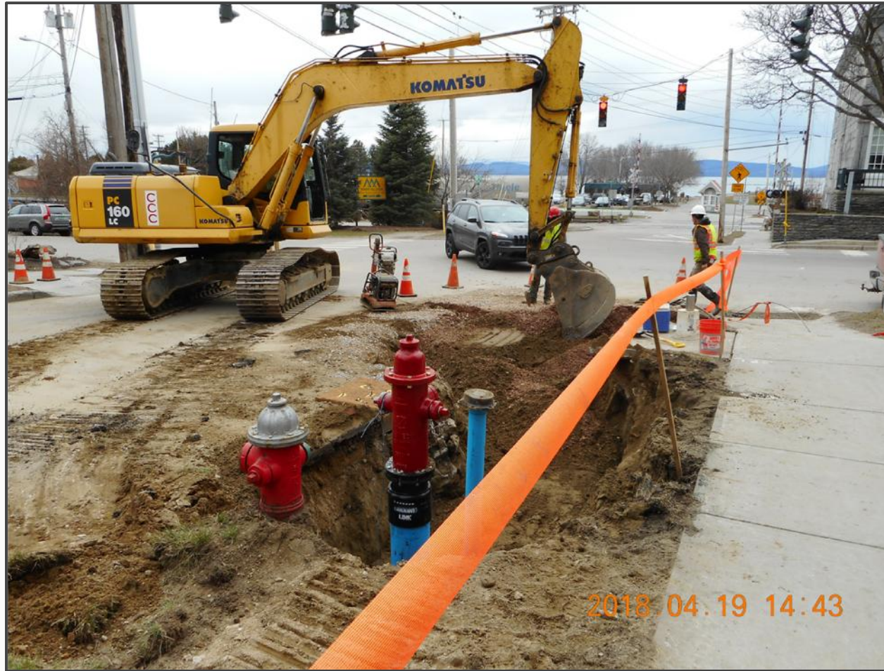
LOWER DOWNTOWN CAPITAL PROJECTS & LOWER PINE STREET
