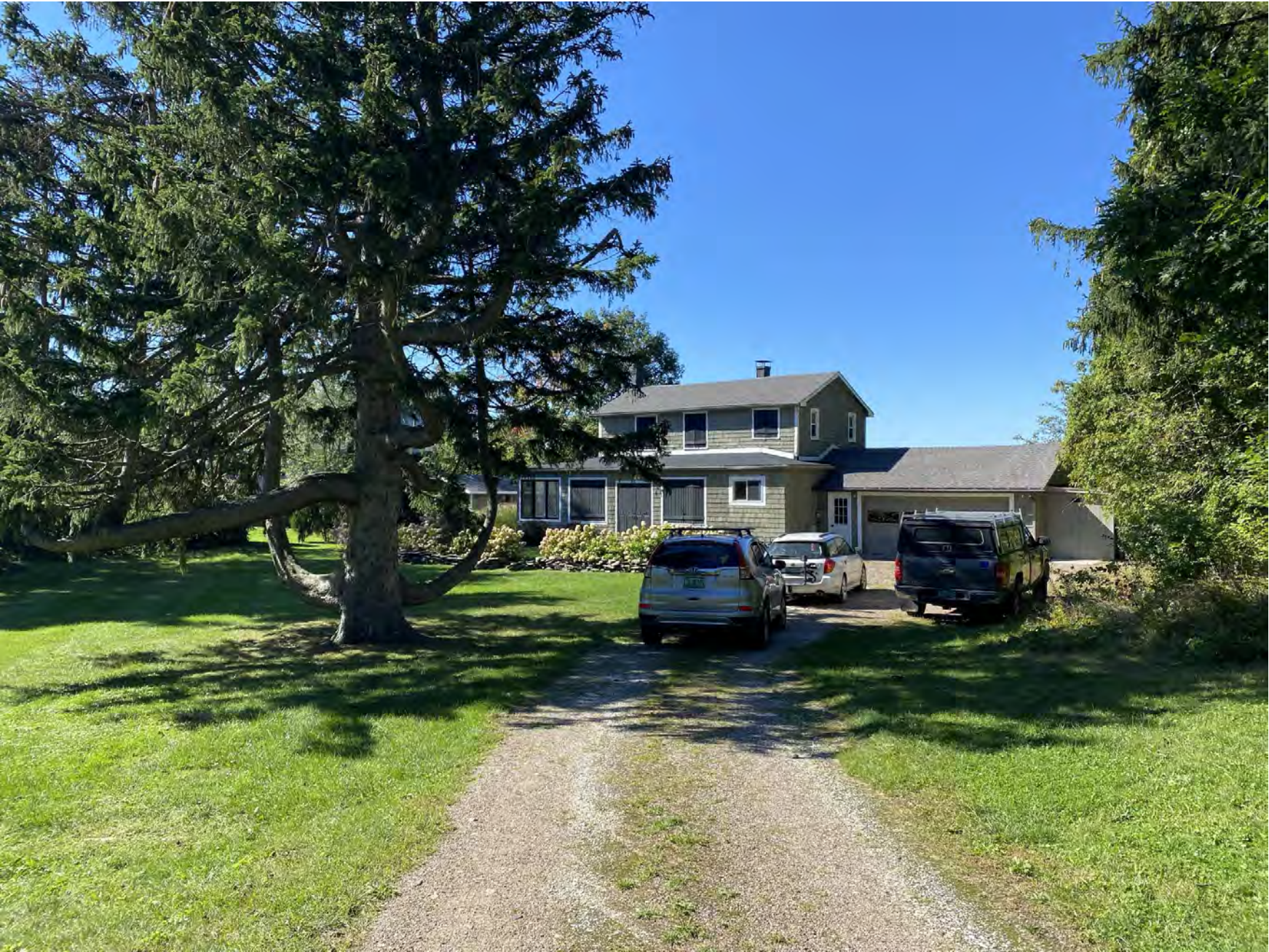
LOCATION 1 - LOOKING WEST
