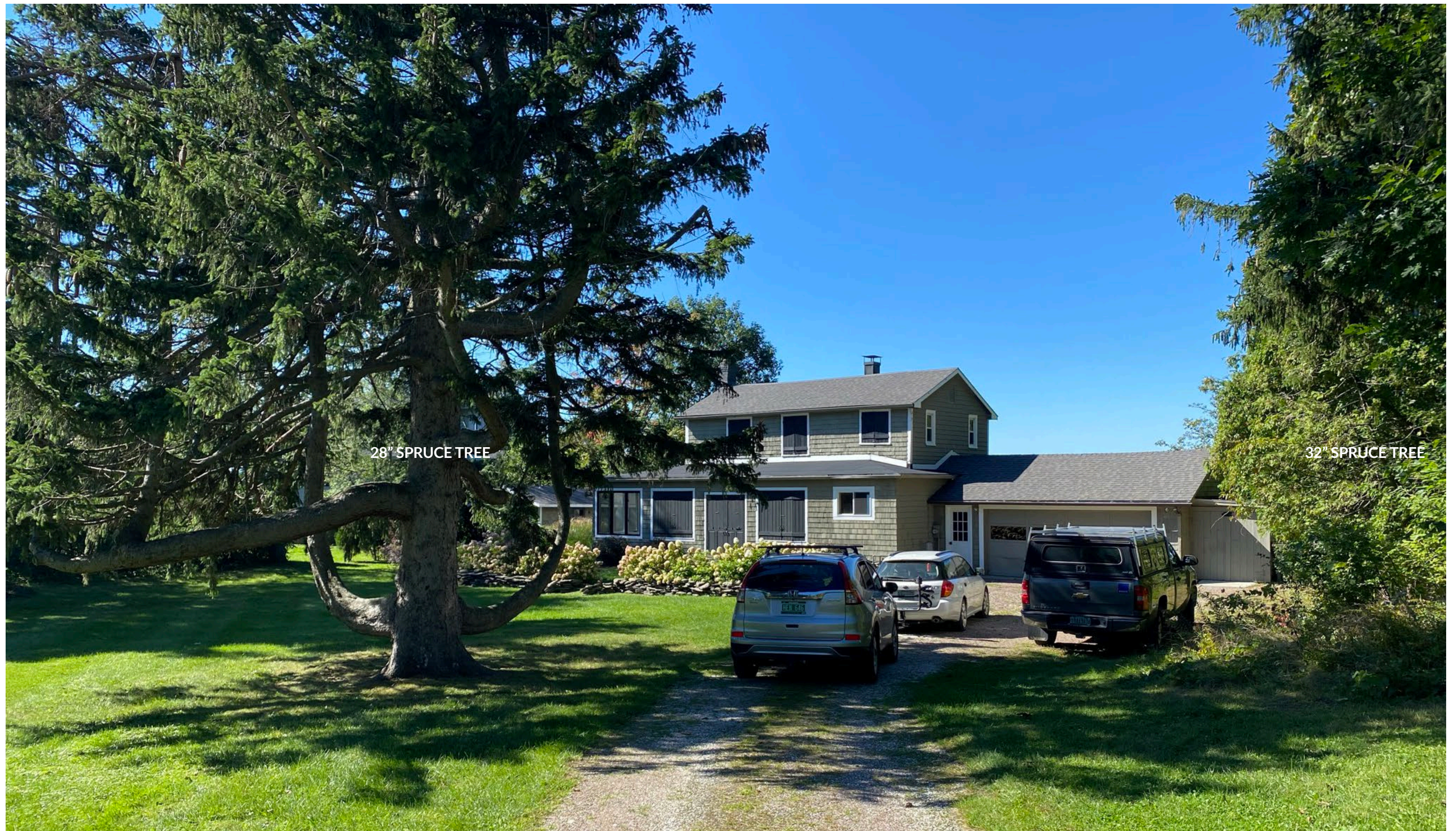
EXISTING SITE PHOTOS // Driveway looking west
