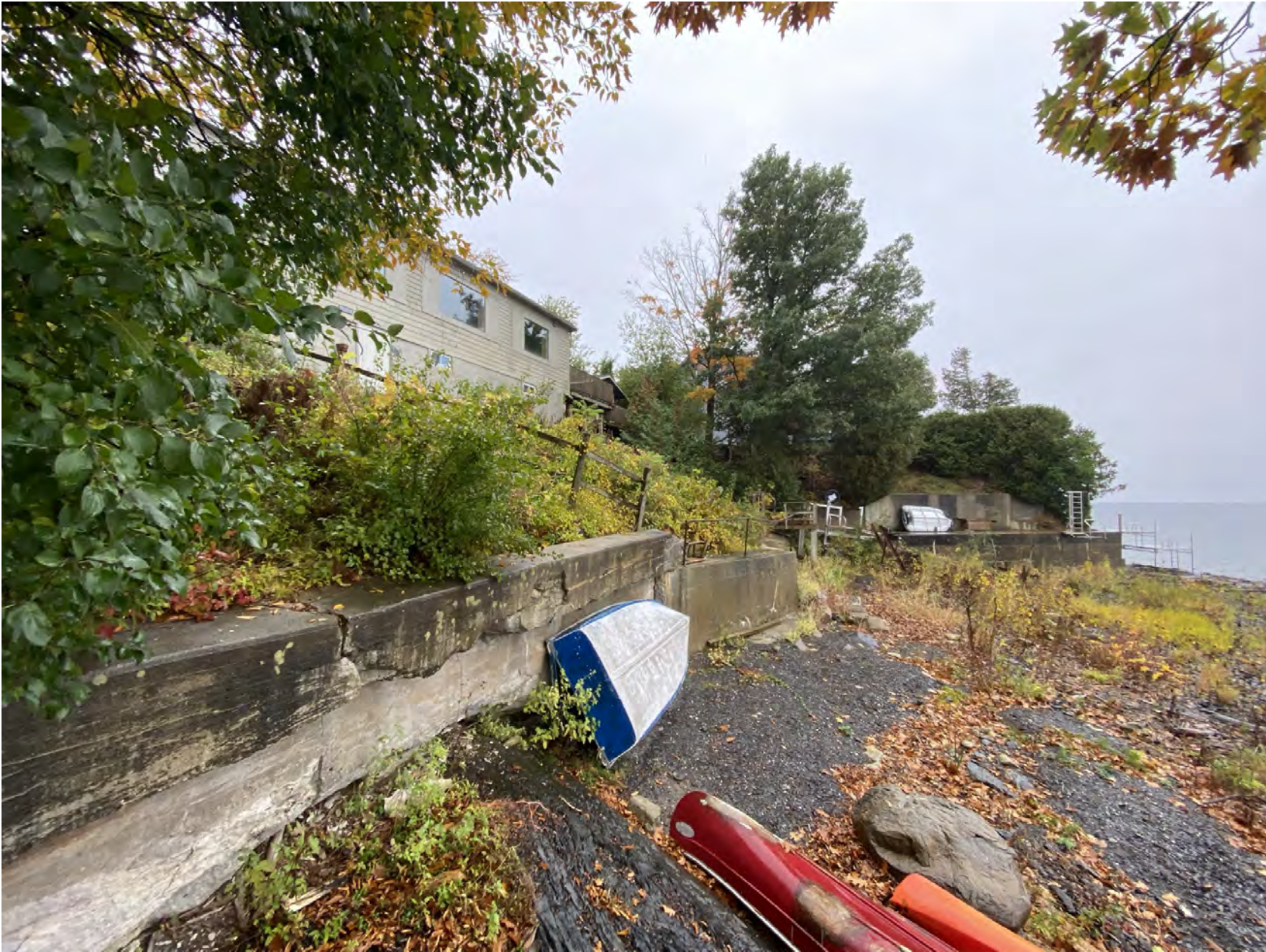
LOCATION 4 - LOOKING SOUTHWEST
