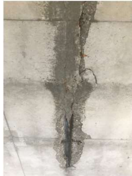
Spall Removal and Sealing
