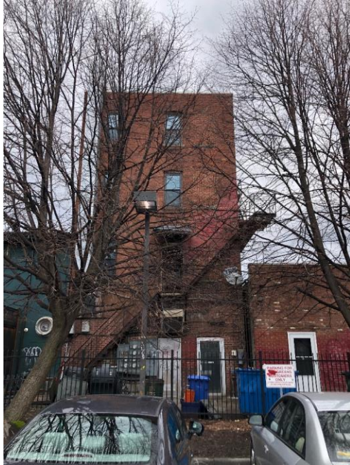
South elevation, photo taken from parking lot south of the alley. Note three windows infilled on the right.
