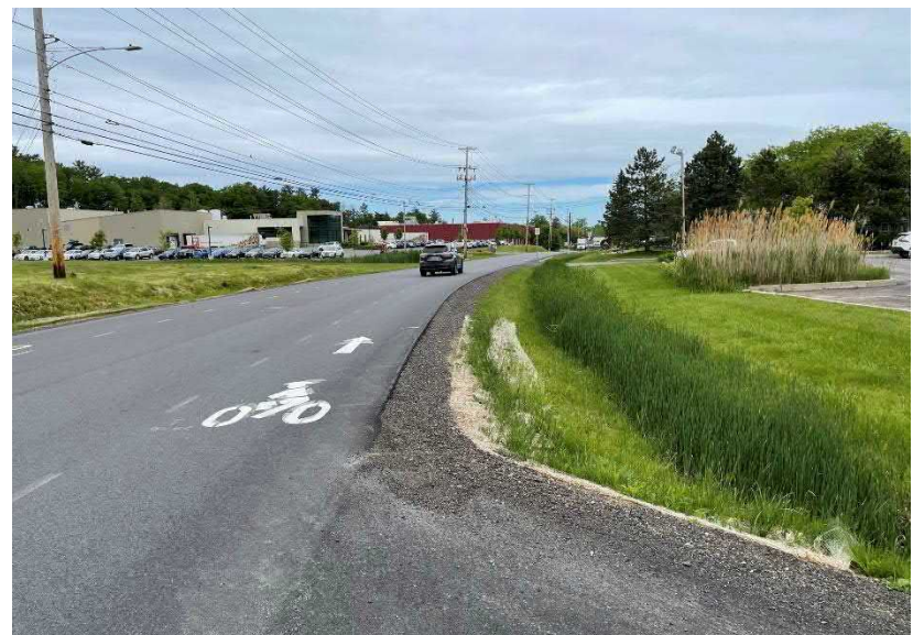
Drainage swale and utilities near Rhino Foods
