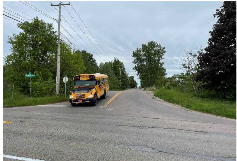
Pine Street intersection
