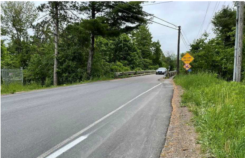
Approach to bridge from west
