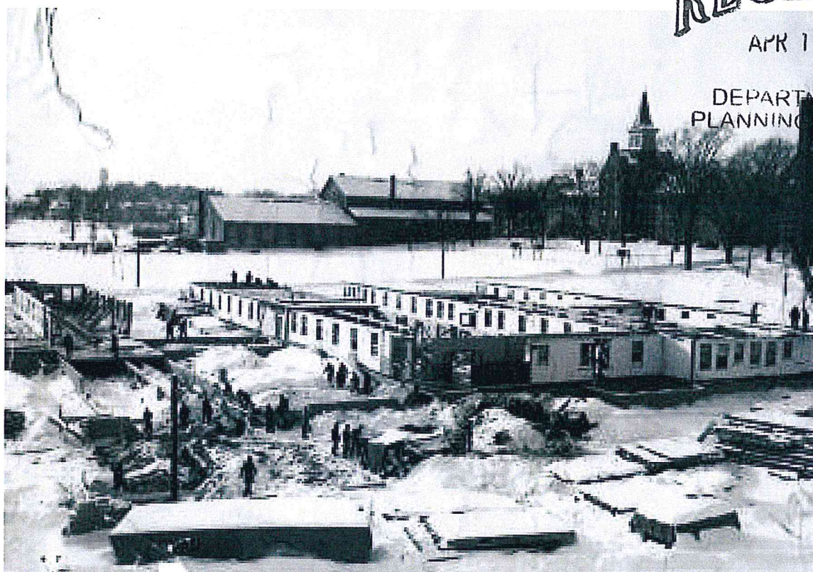
13. Construction of East Hall, 1946? Royall Tyler Theater (formerly the gymnasium) is in the background.
