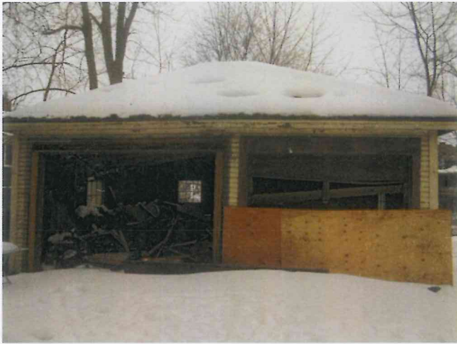
Photo #1 - Front (East) Elevation
