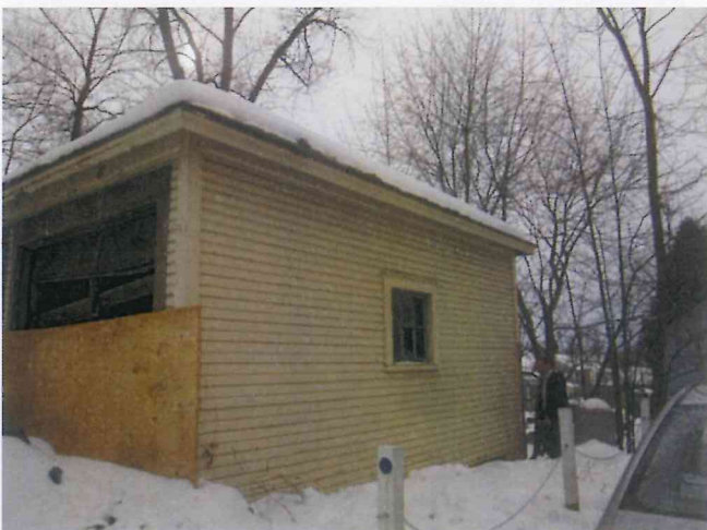
Photo #3 - North Side Elevation
