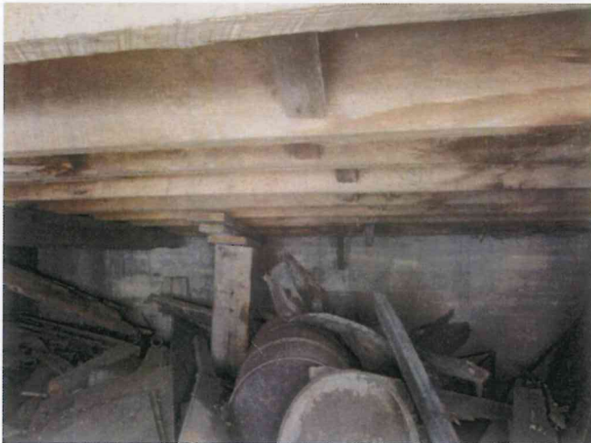
Photo #18 - East wall, and timber post with shims
