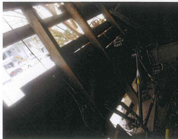
Photo #21 - West wall
