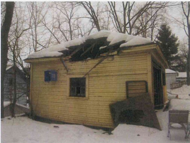
Photo #2 - South Side Elevation
