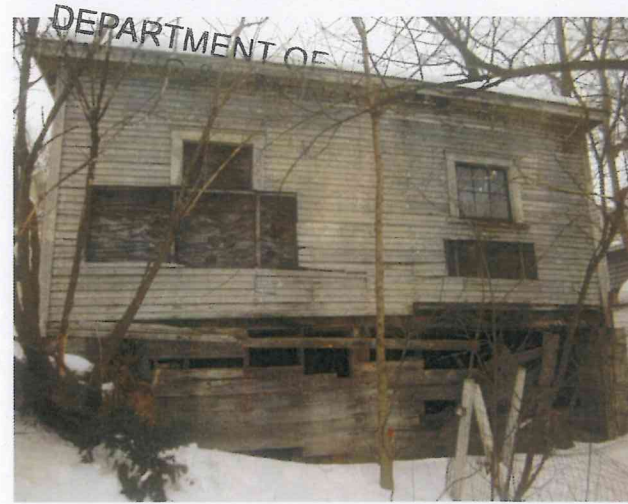
Photo #4 - Rear (West) Elevation
