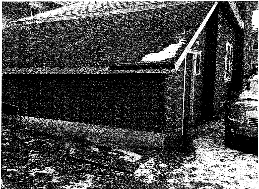
Existing attached shed to be converted
