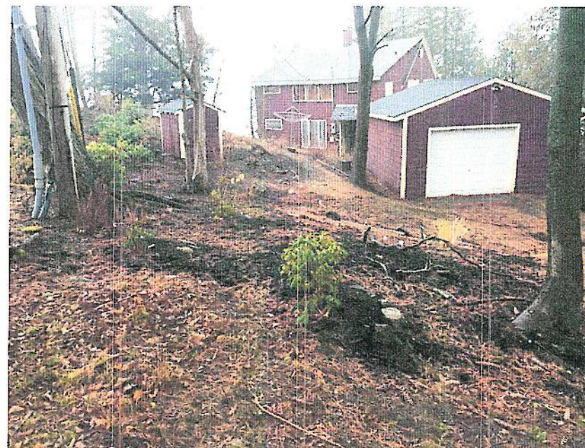
EXISTING GARAGE FROM EAST WITH HOUSE BEYOND
