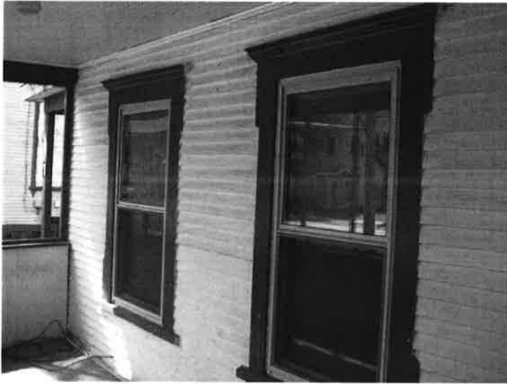
19. The window trim details around the two windows on the front elevation of the building are among the few remaining historic features on the building;
