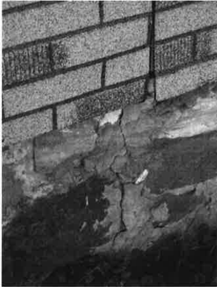
50. (Left) a substantial crack is visible in the south side foundation near the bay window; cracks also exist in the bay window (right) foundation.
