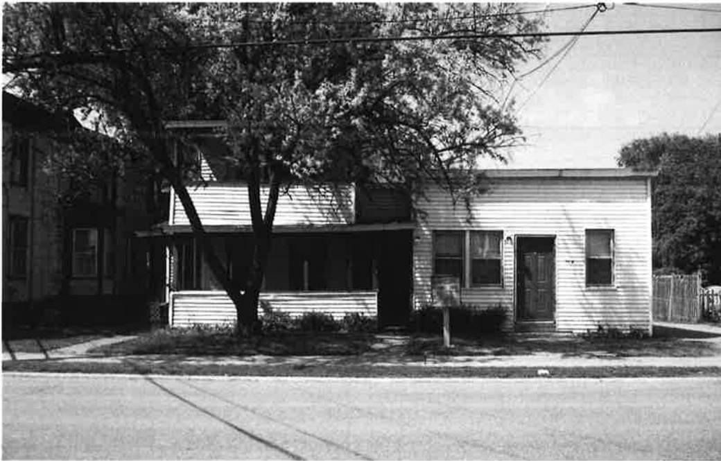
1. 114 Archibald Street looking north.
