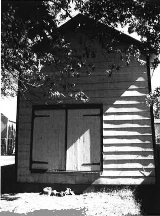
34. Rear (west) gable end.
