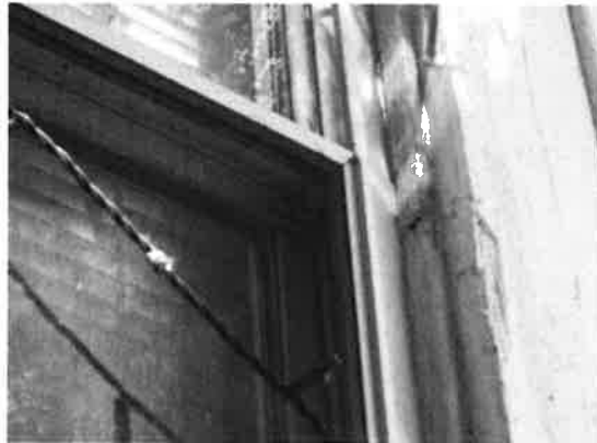
53. (Left) The bay window cornice is in poor condition in many areas such as above.
