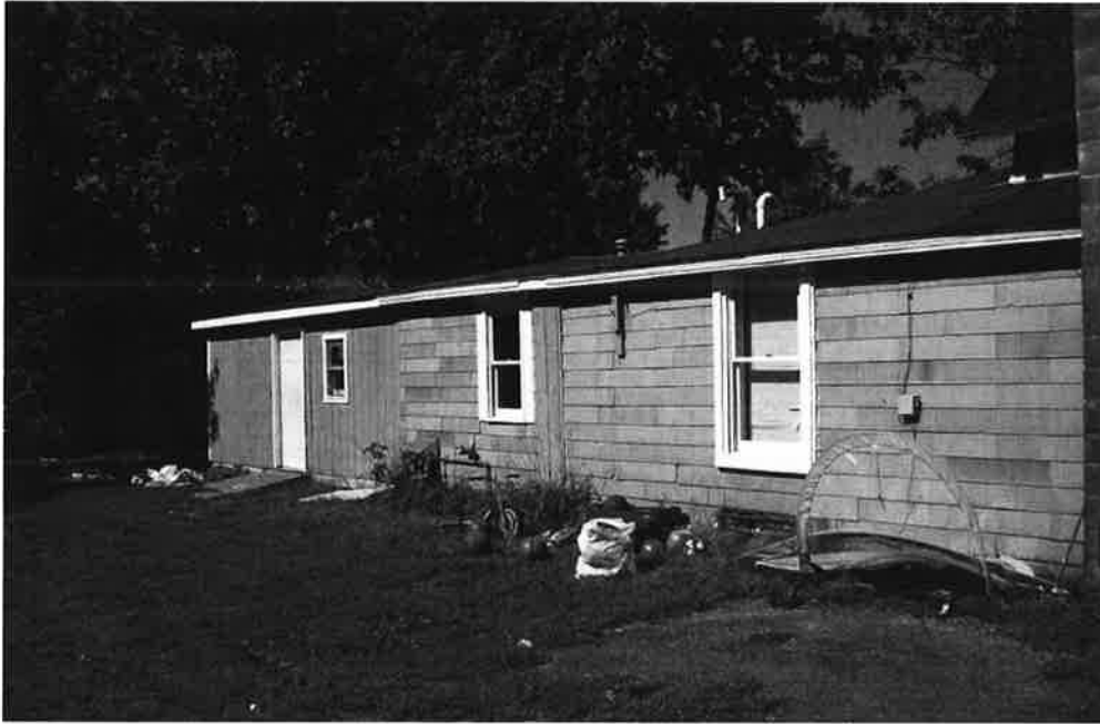
84. Additional view of the south elevation of the rear additions.
