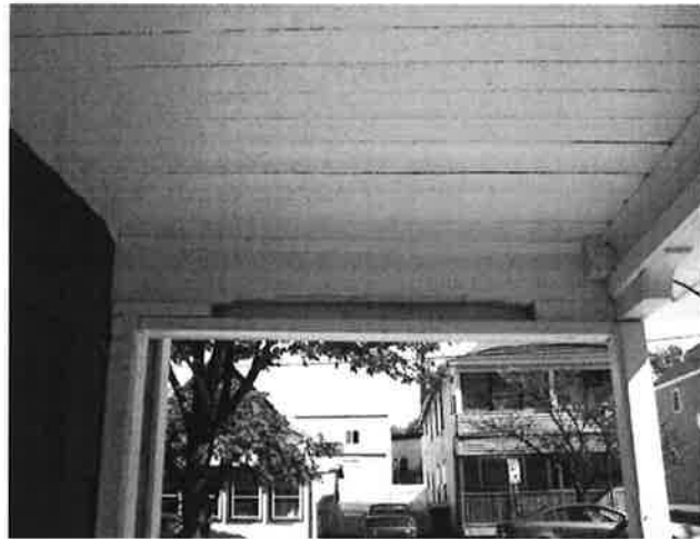
90. & 91. Front porch ceiling and frieze band appears old; other elements including posts are new.
