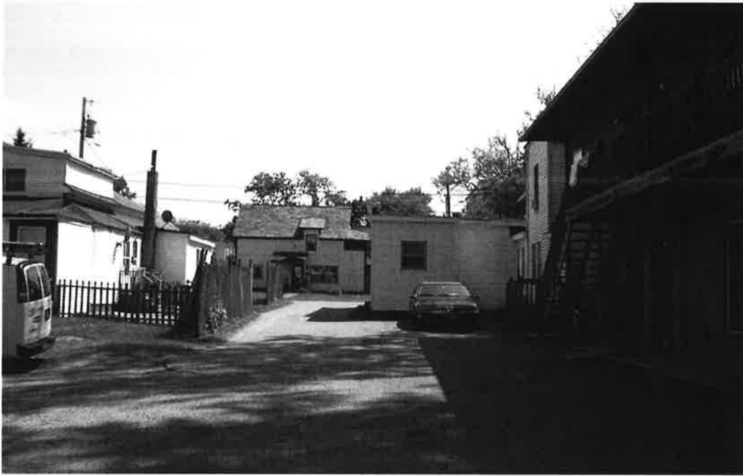
15. View looking south showing east elevation of 114 Archibald Street.
