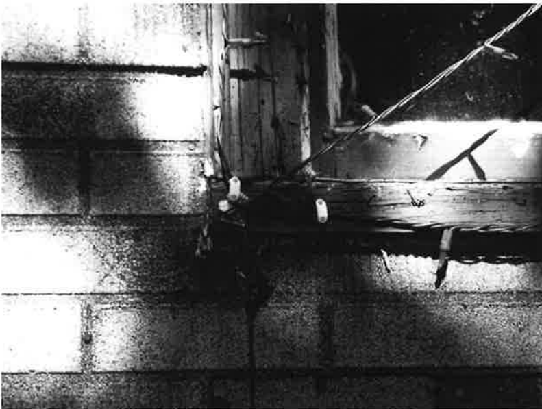
62. Additional view of window trim and sash.
