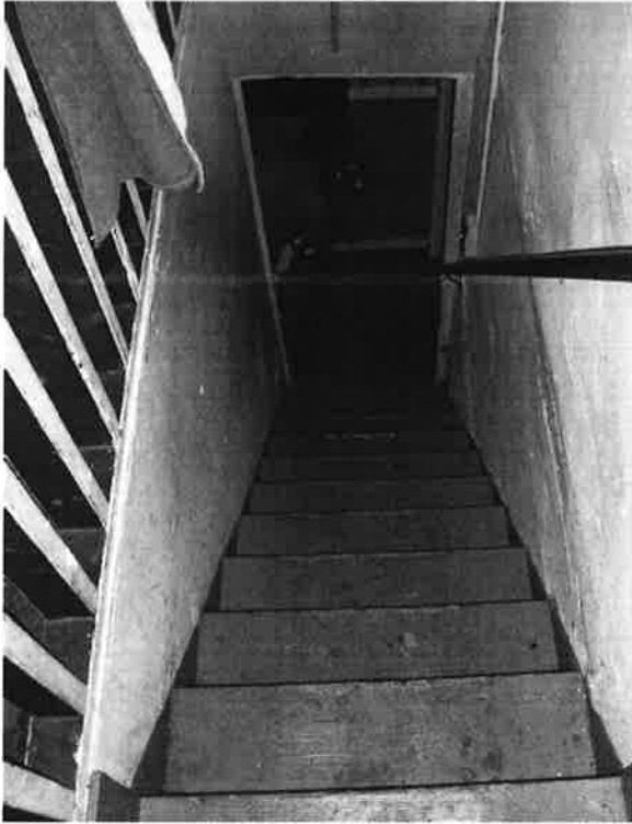
76. Looking down stairs to first floor of main block.
