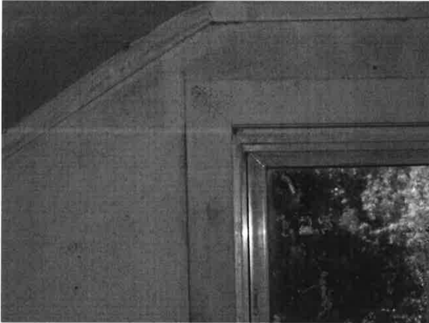
80. Typical view of replacement trim and window on second floor.
