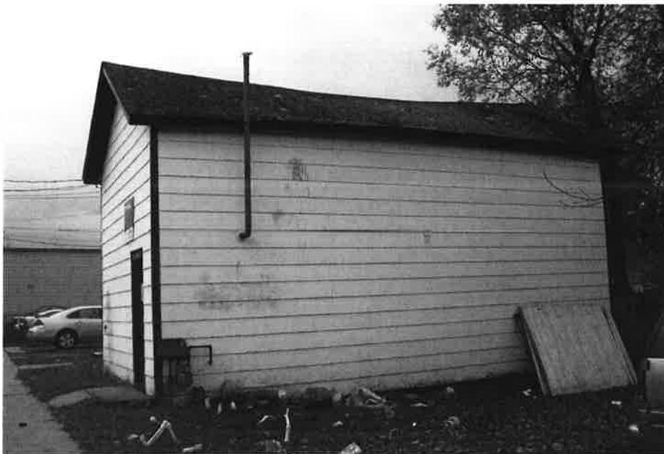
31. Storage shed, north and front (east) elevation. Note significant sag in roof.
