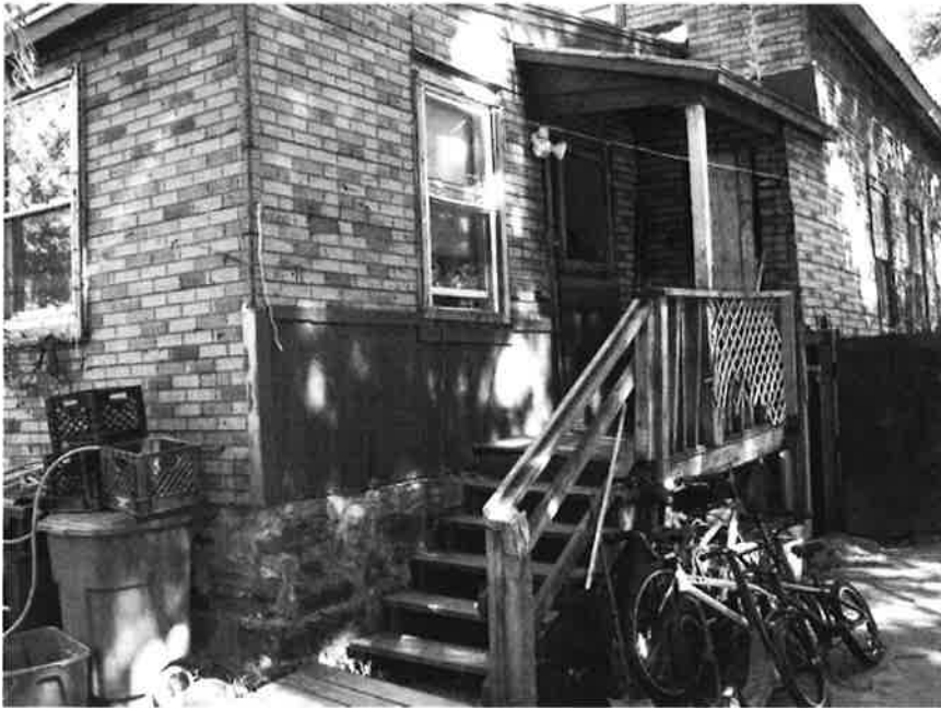
47. Detail of the southwest corner of the rear ell and main block. All porch features are new.
