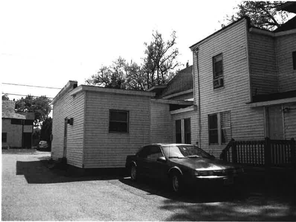
11. View looking south along the east elevation of 114 Archibald Street.
