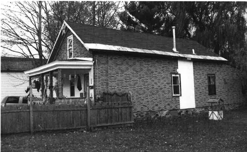
43. North elevation with two historic two-over-two windows at the far right. Note early redstone foundation.
