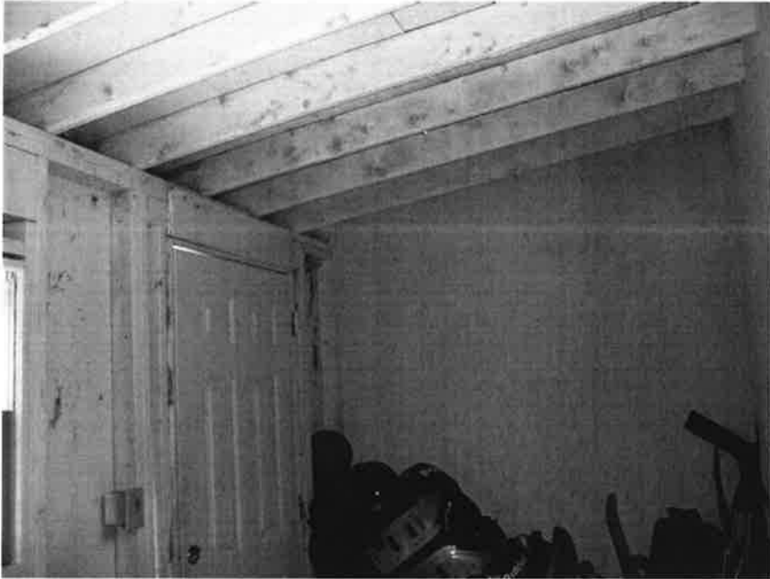
96. Interior view of west end appendage looking southwest.
