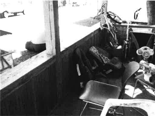
57. (Left) Front porch railing and posts are new.
