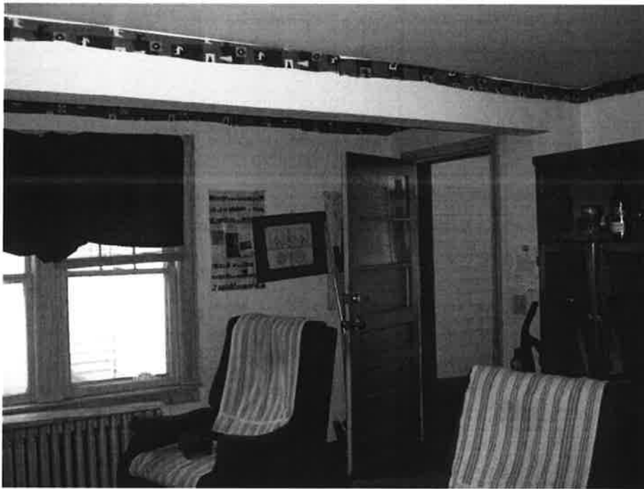
21. First floor unit in historic front portion of building; note that overall, historic features and finishes have been replaced, and floorplan configurations have also been changed.
