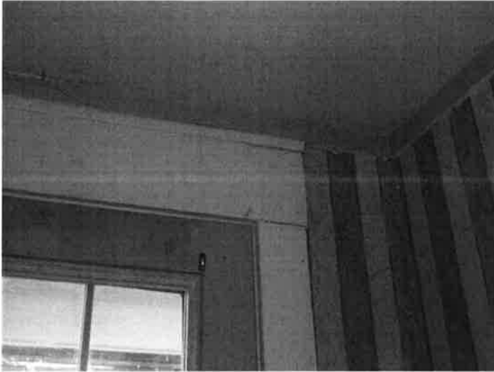
65. Interior view of replacement front entry door and flat stock trim.
