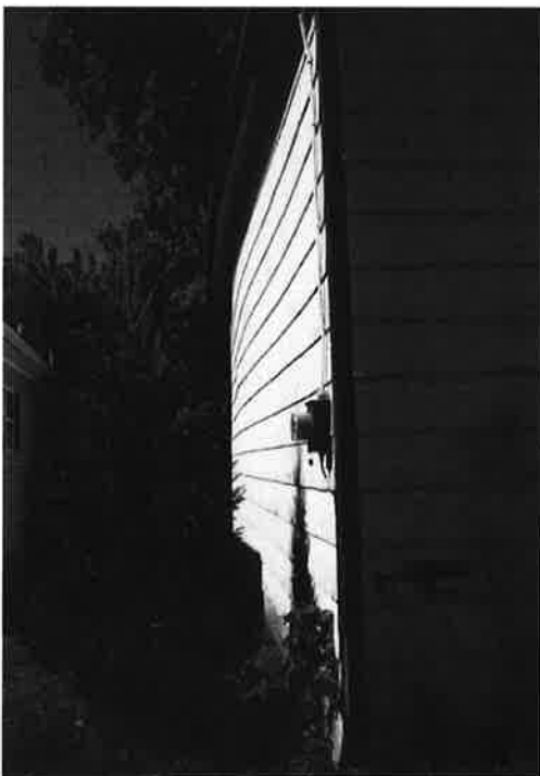
32. (Left) View of south wall on left which is bowing out.
