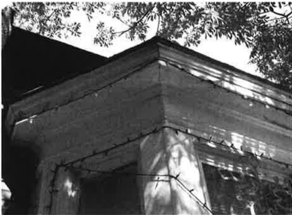
51. Detail of the wood trim on the bay window.
