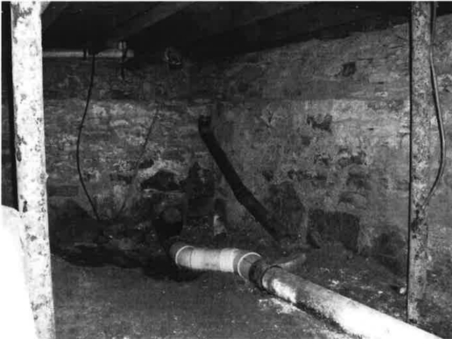
26. The stone and concrete foundation in the basement.
