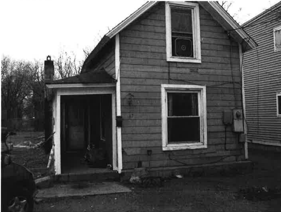
82. 47 Bright Street. Front elevation. Note replacement windows and front door, asbestos shingle siding, intrusive concrete block chimney on south elevation.
