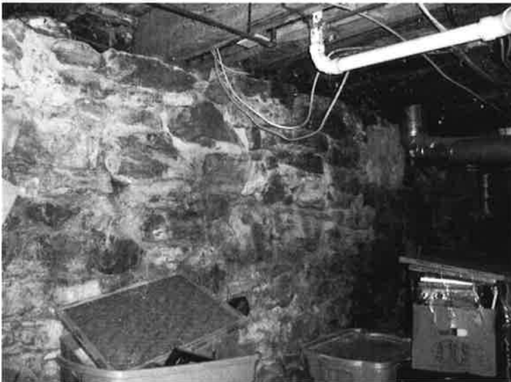
64. The stone and concrete basement foundation.
