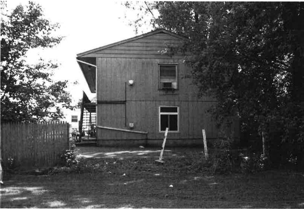
16. Rear (north) elevation of the modern rear addition.
