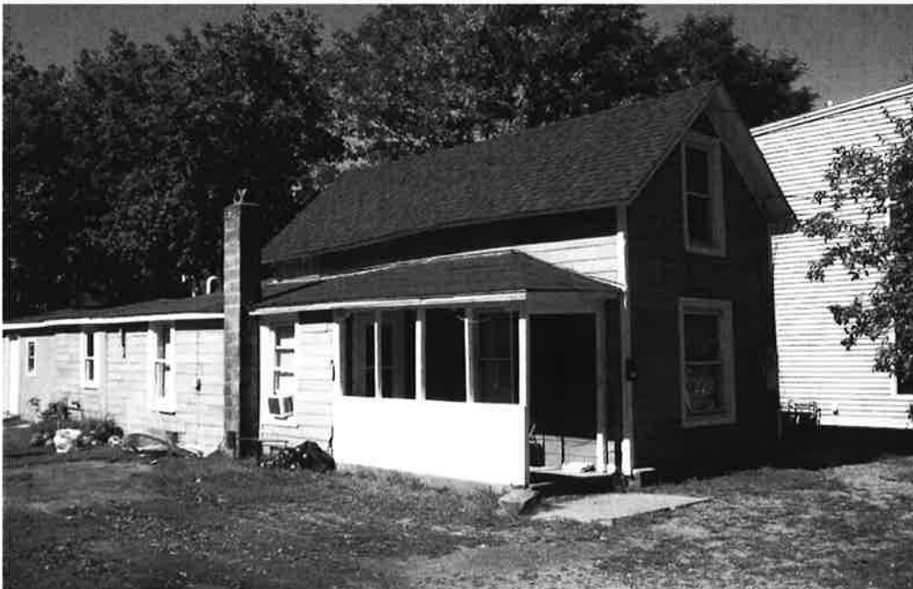
83. South elevation of 47 Bright Street. Rear additions and concrete block chimney appear to be non-significant additions, and the side porch appears to have been replaced with new posts and closed railing.
