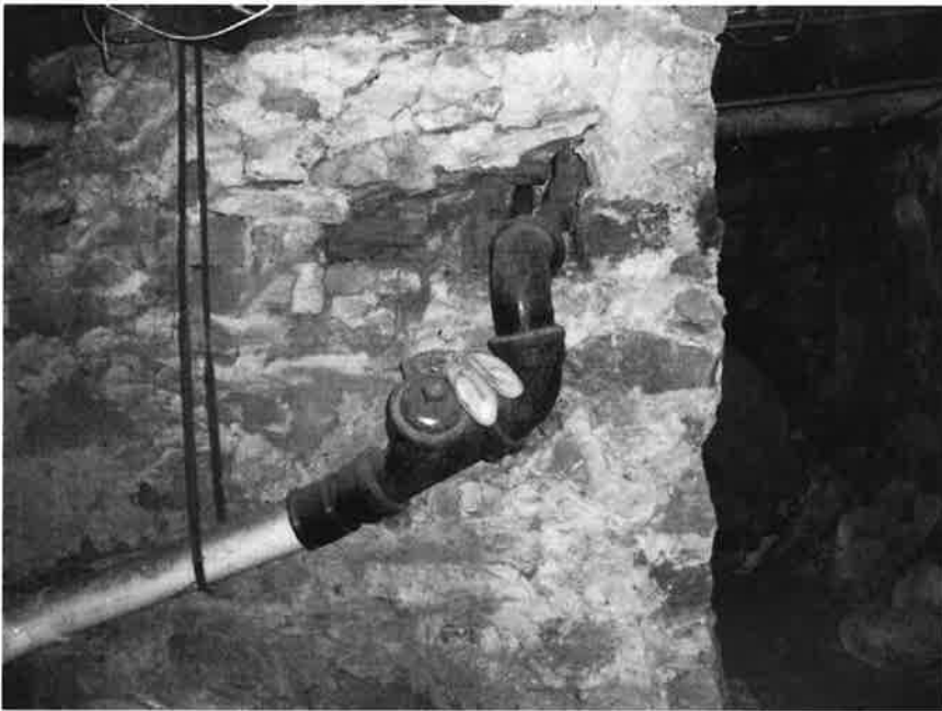
99. The stone foundation in the basement.
