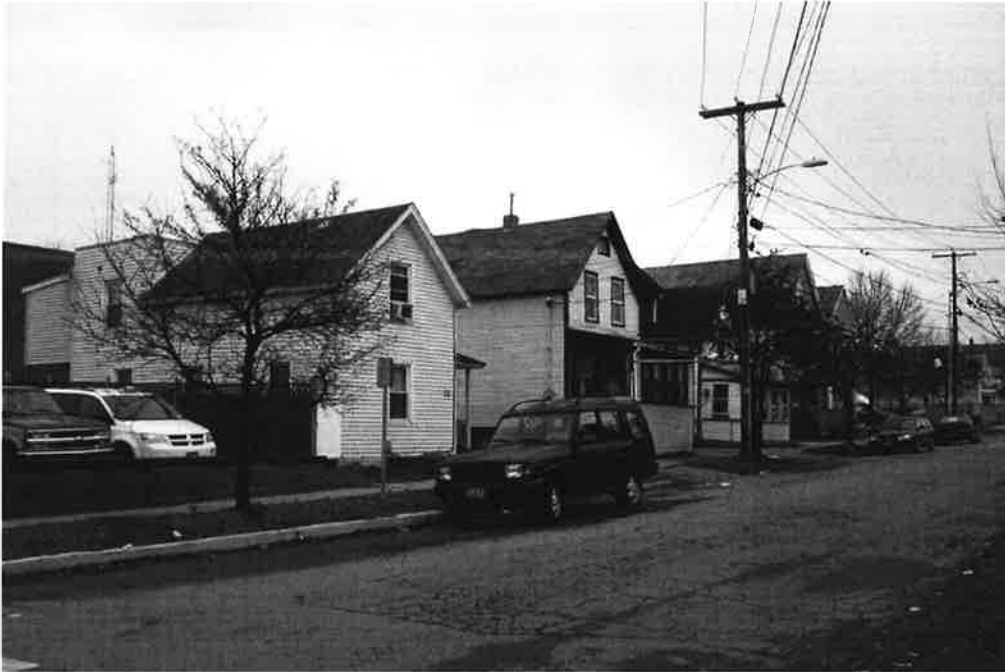
29. Context view of Bright Street looking south east; east side of street just south of Riverside Ave.
