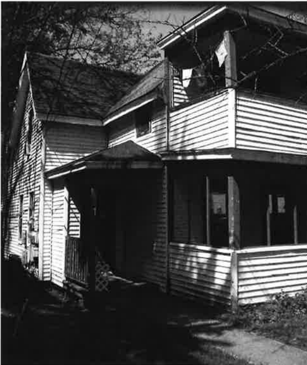
10. Additional view of the west elevation.
