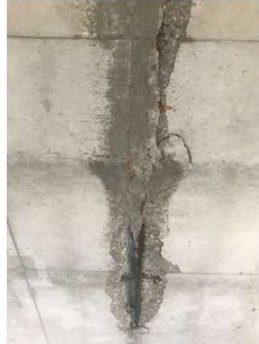
Spall Removal and Sealing
