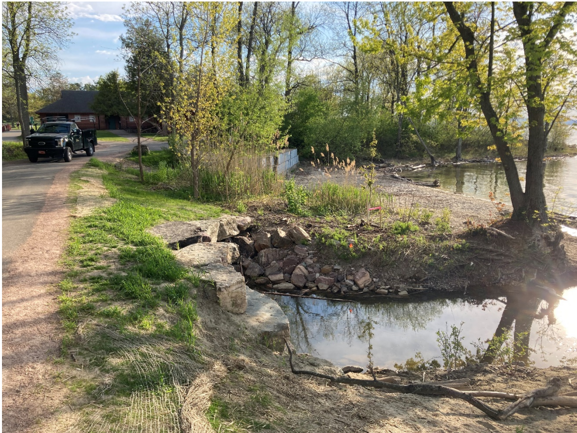
Photo 2. View of the outfall of the unnamed stream looking south from the Bike Path, showing the installation of shrub and sapling riparian buffer plantings on the south bank Photo by VHB, May 17, 2021.
