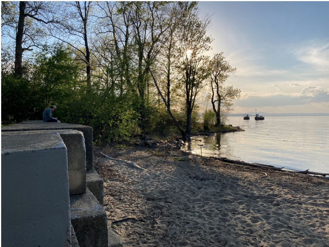
Photo 1. View of the waste block seawall and beach area proposed to be replaced by the Pause Place. View is to the west-southwest. Note the relatively intact shoreline vegetation in the background would be affected by shifting the Pause Place to the south. Photo by VHB, May 17, 2021.
