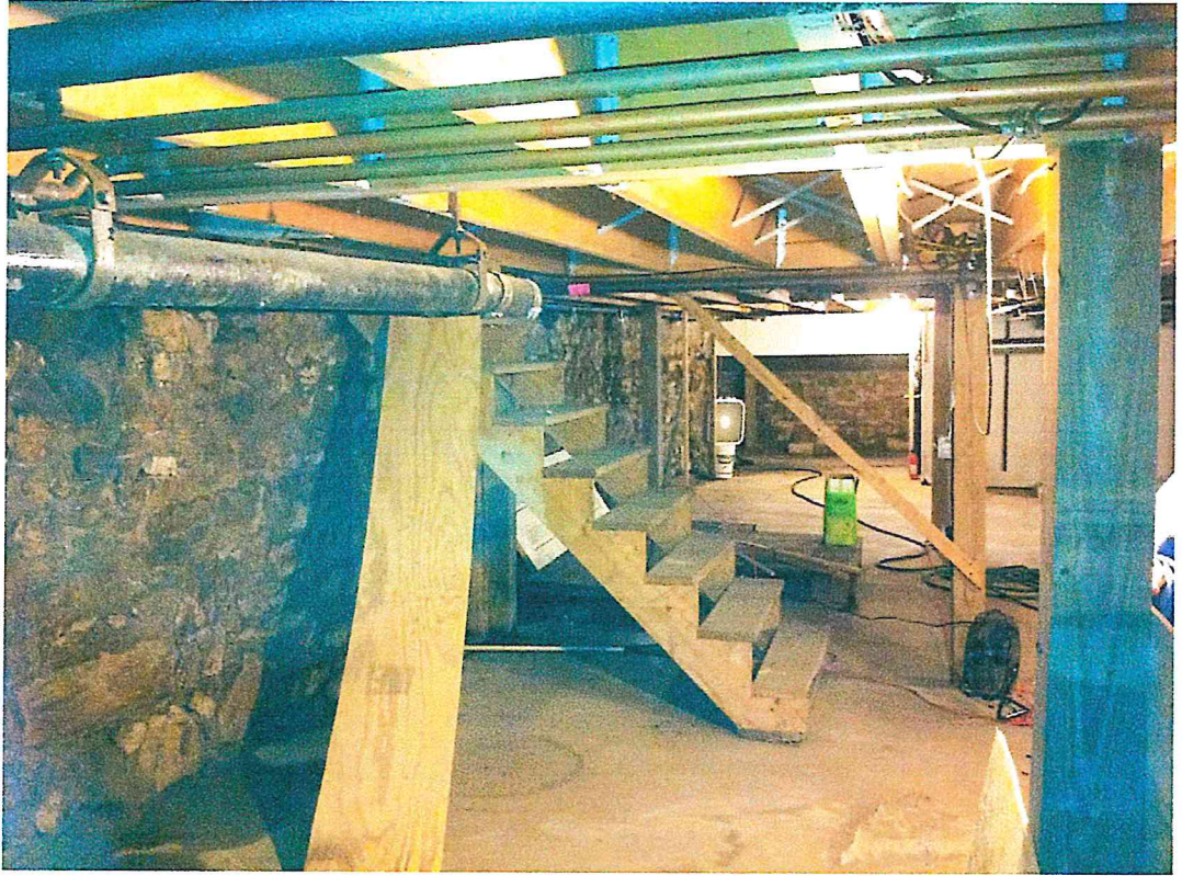
Photo 7. Existing south wall of cellar. Structure of First Floor above is modern, made of 2x10 joists and 6x6 posts spaced 12' apart.
