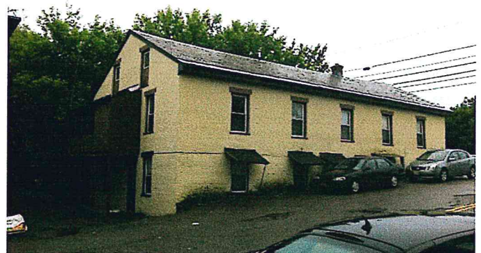
View of window wells and shed roofs over them we want to remove.
