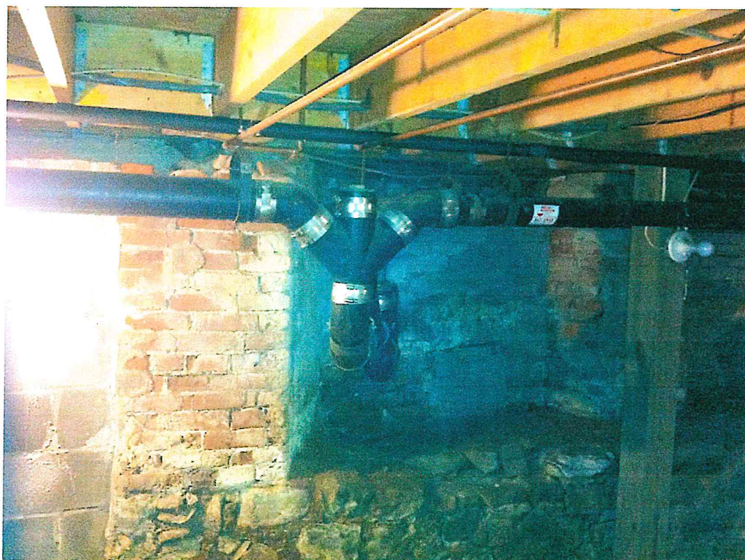
Photo 24. East wall of cellar, showing original on-grade entrance on the left, now blocked with concrete blocks. The pair of windows on the right, provided natural light and display features from the east end, which was fully above grade at this level before 1928. Now sewer lines from the apartments above gather and exit here.
