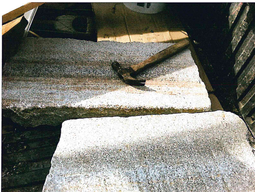
Photo 38. This photo shows two the granite stones that will be used to reconstruct the foundation wall between the top of the existing stone foundation that will remain and the bottom of the brick at the lifted building. Sizes are similar with similar cut to the existing stones, but these are grayer – compatible, but different so they do not fool someone to thinking they are the original stones. These stones will only be visible on the exterior and will be backed up to a new insulated concrete foundation wall on the interior, faced with plaster.
