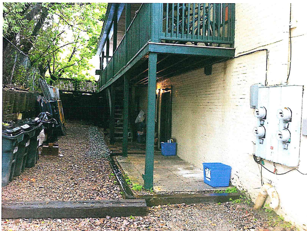
Photo 39. Location of existing meters on east end of south elevation. Intent is to move these to the west end of the south elevation after the building is lifted and service the building with an underground primary feed from the existing power pole near that location. One additional meter will be included for the Café. If possible, all meters may be put inside the building if Green Mountain Power can accept "smart metering" at this location with a remote reading ability for each meter.
