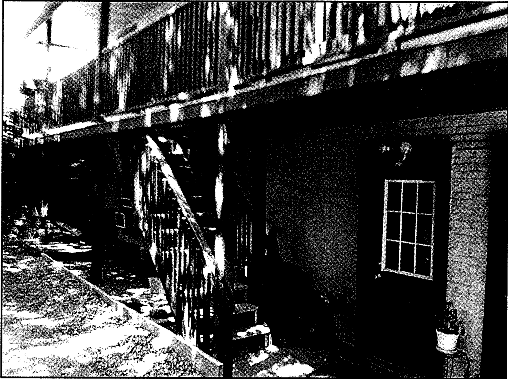
EXISTING CONDITIONS, SOUTH SIDE COURTYARD
