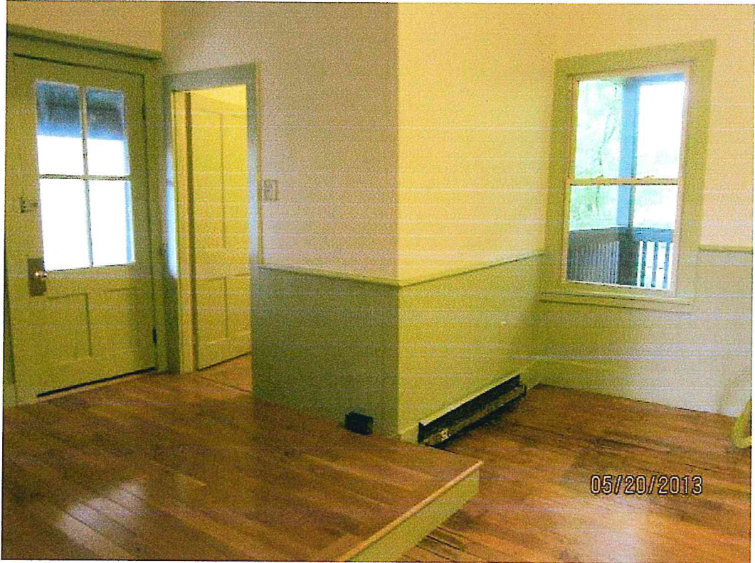
Photo 33. Kitchen (on raised platform) and living space of apartment (#2) at east end of Second Floor. Door with glass leading to the mostly-enclosed east porch replaces an historic window.
