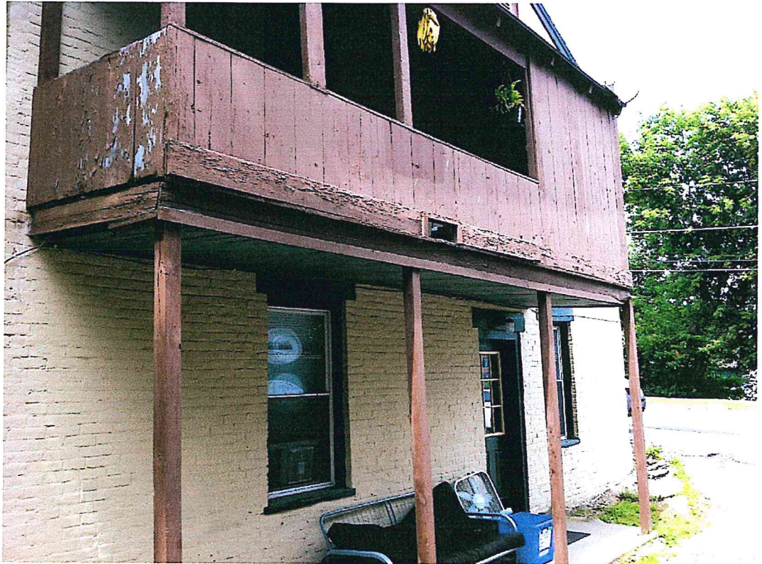
Photo 21. East side showing added porch and door cut in to access the apartment at the east end of the first floor in 1928. The porch was built after 1928.
