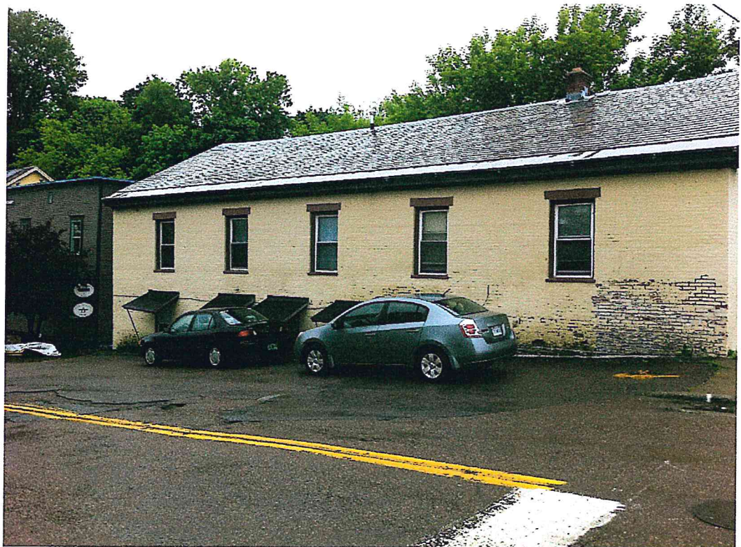
Photo 4. North elevation photo taken 2014.
