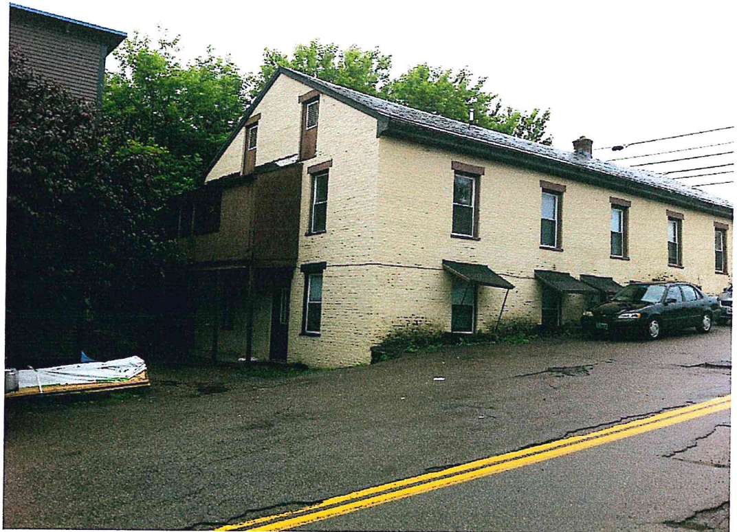
Photo 20. East and North elevation showing location of first and second floor doors and windows. The door just to the left of the window on the east elevation is not original and was cut in to access the apartment at the east end of the first floor in 1928.
