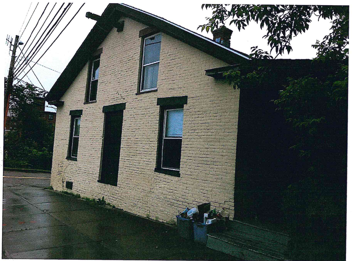
Photo 2. West elevation taken 2014. What is now a blocked in doorway just above the sidewalk used to be a door to the second floor porch seen in Photo 1. The porch was removed when the building was buried. Windows have been replaced with 1-over-1 windows, instead of the original 2-over-2 windows seen in the historic photograph.
