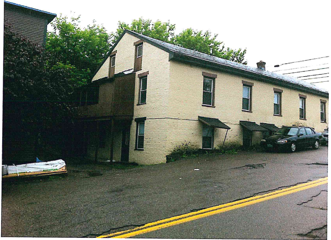
Photo 9. The first floor apartments are currently at grade level on the east end of the building shown here. The apartment door is not original and was cut into the brick façade. Originally this floor was about 9 feet above grade with the cellar having an on-grade access at this end of the building.
