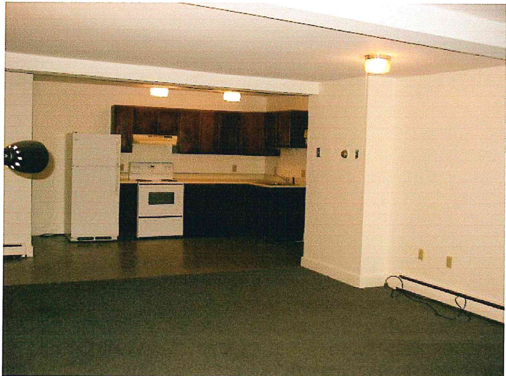
Photo 26. First Floor, west end apartment (#3). The rooms in this mostly buried apartment get almost no natural light. The original beams supporting the second floor are 8x8 wood beams that have been covered in sheetrock. No historic fabric remains at the interior of this level, except for the heavy timber frame made of 8x8 beams that support the second floor and attic floor.
