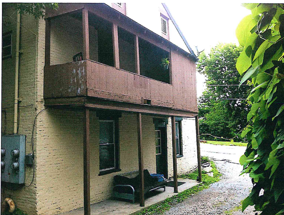
Photo 13. Exterior porch, east side was first built in 1916 and remodeled later to its present condition shown here. The door at the upper level replaced a former window from the 1820 design. The lower door was put in after 1929, as the first floor was well above the ground floor on the east side.
