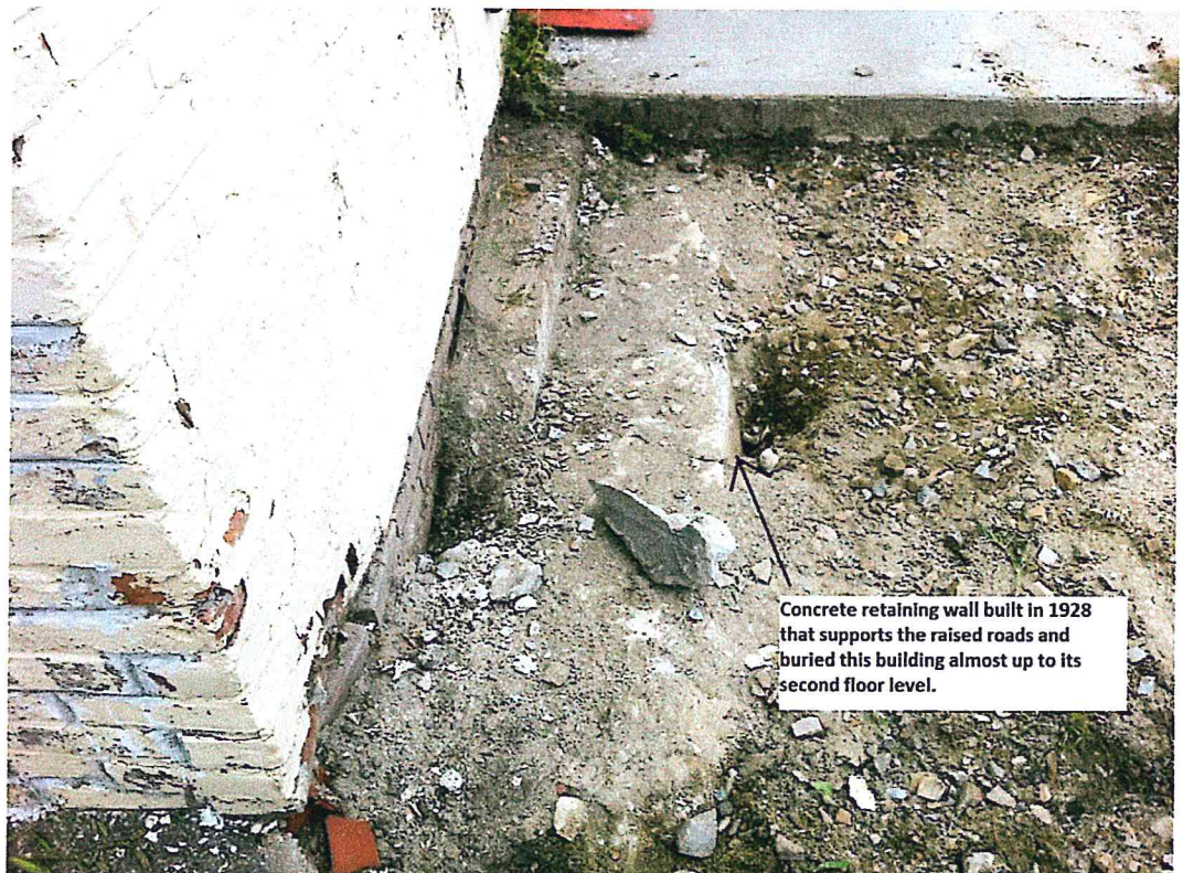
Photo 36. Detail at top of retaining wall at west side of building.
