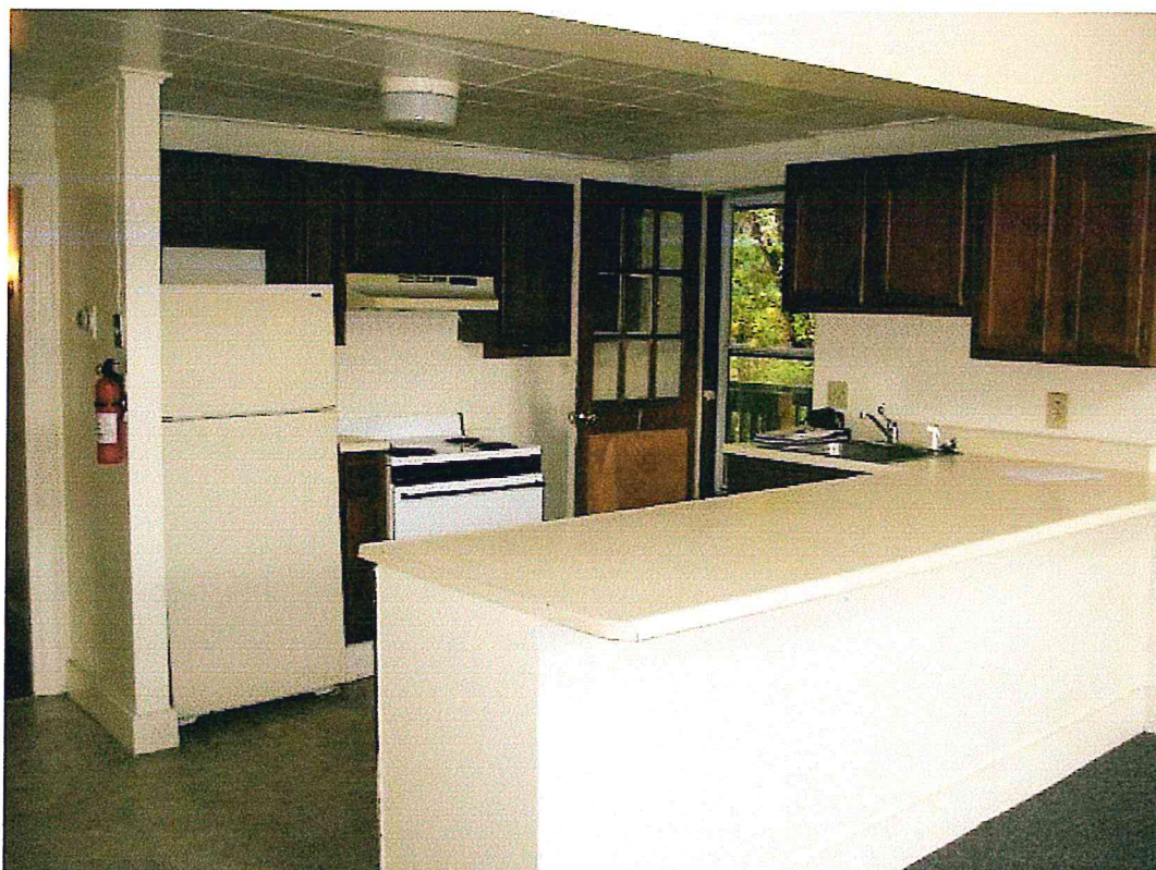
Photo 32. Kitchen of apartment (#1) at west end of Second Floor. Beam in foreground is one of the original 8x8 framing timbers, now wrapped in Sheetrock. No historic fabric exists at the interior of the first or second floors.
