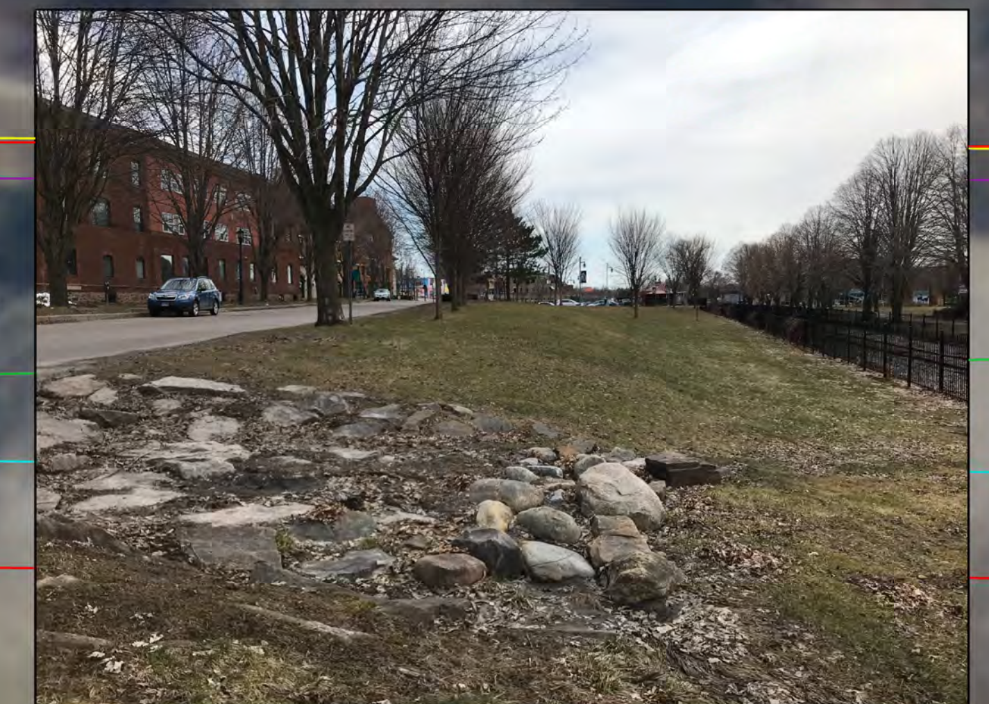
EXISTING TREATMENT LOOKING SOUTH
