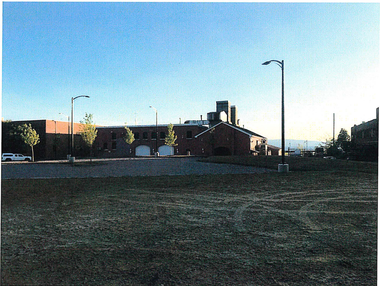
Burlington Electric to South
