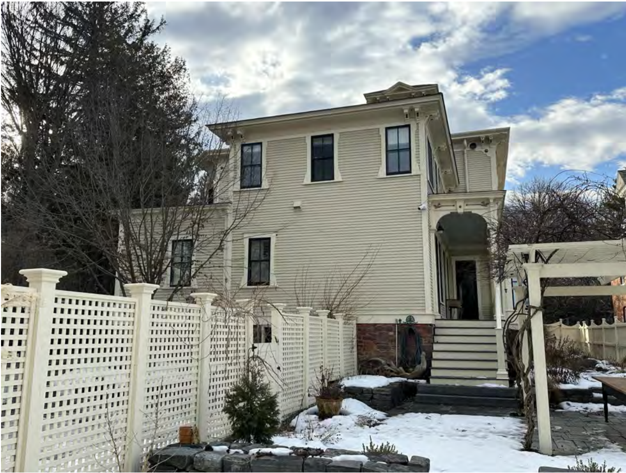
MAIN HOUSE - NORTH FACADE (LOOKING SOUTH)
