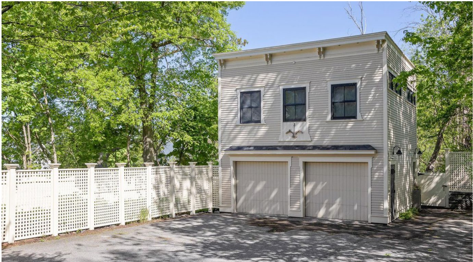
SOUTH FACADE - PRESENT DAY
