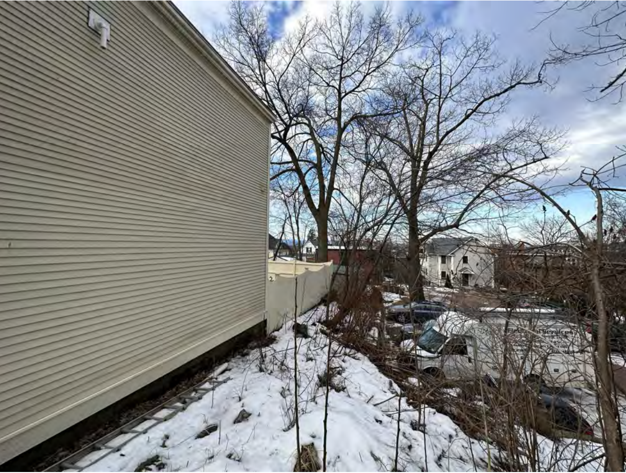
CARRIAGE BARN - NORTH PERIMETER (LOOKING WEST)
