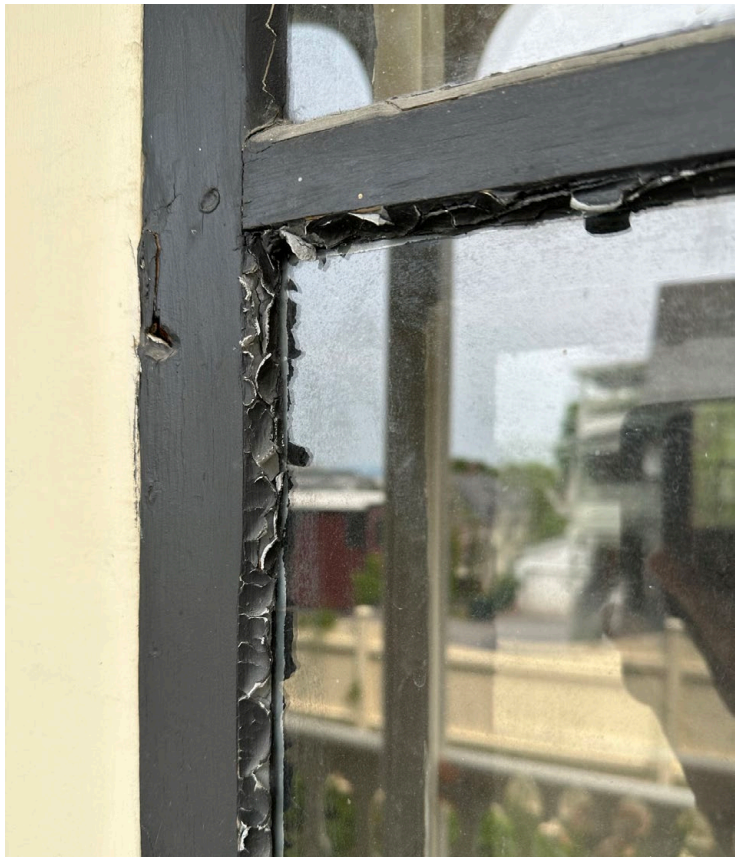
SEALANT FAILURE
