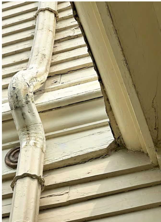
MAIN HOUSE - TYPICAL CONDITIONS OF GUTTER & TRIM DETAILS
