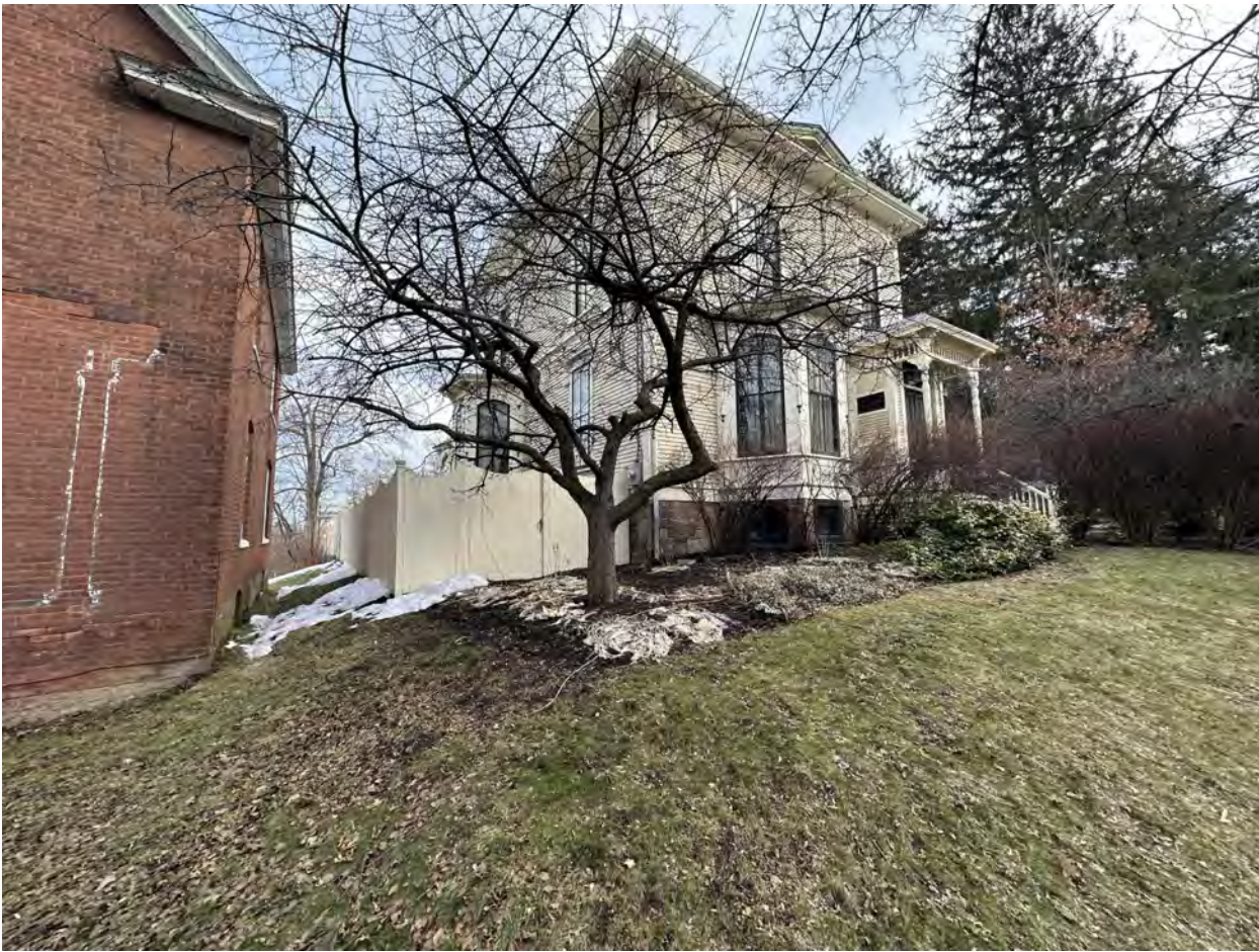
MAIN HOUSE - SOUTHWEST FACADE (LOOKING NORTHEAST)
