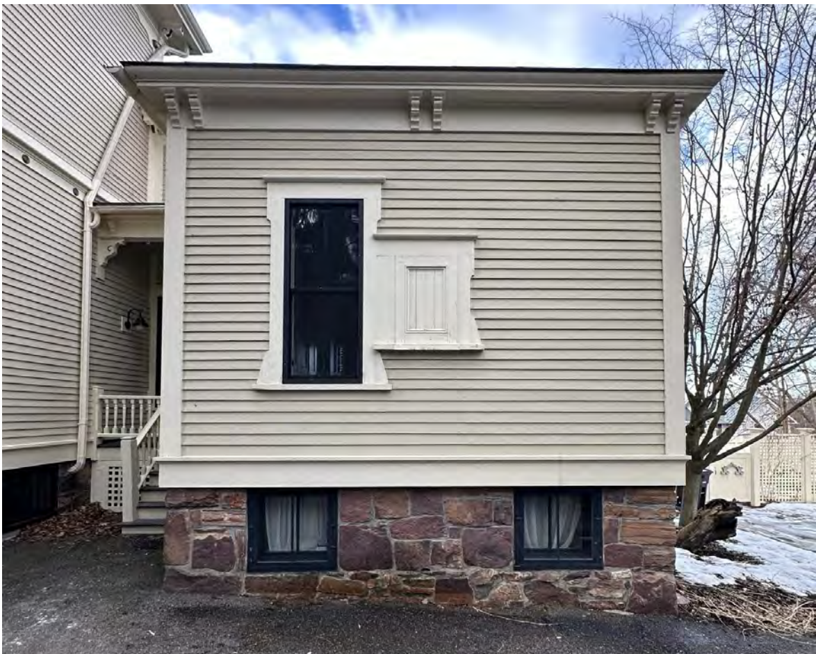
MAIN HOUSE - NORTHEAST FACADE (LOOKING WEST)
