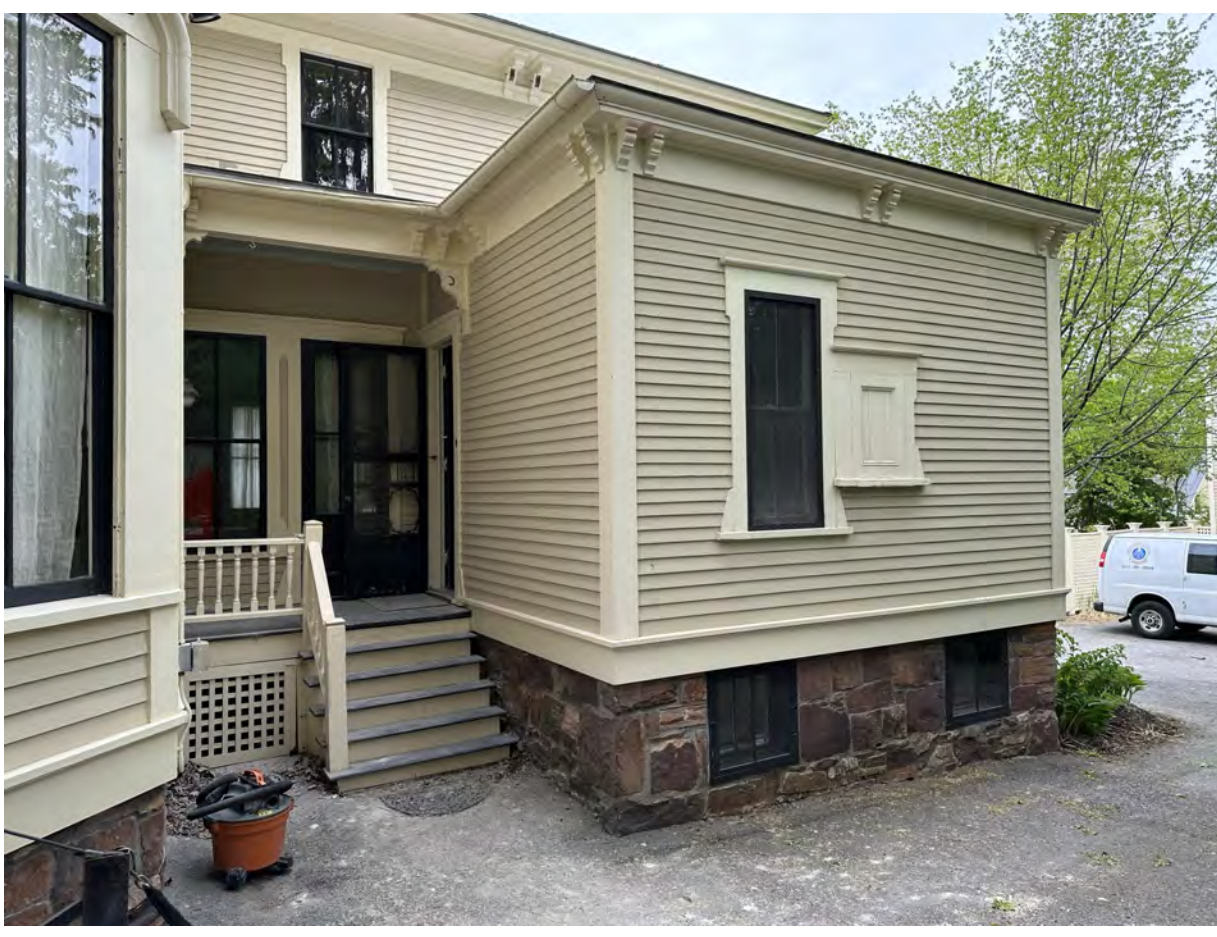
MAIN HOUSE - NORTHEAST CORNER (LOOKING WEST)
