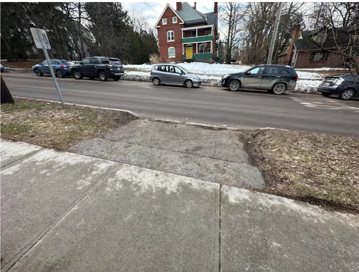
MAPLE STREET CURB CUT (LOOKING SOUTH)
