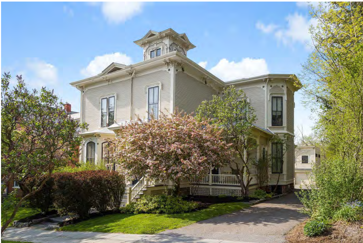
MAIN HOUSE - SOUTHEAST FACADE (LOOKING NORTHWEST)
