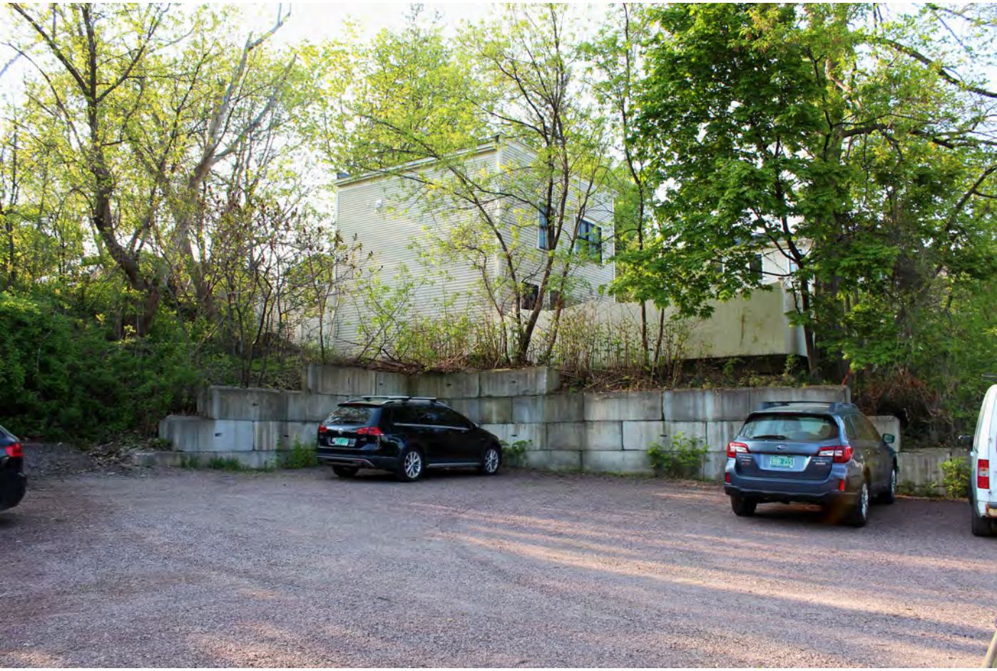
CARRIAGE BARN - NORTHWEST PERIMETER (LOOKING SOUTH)
