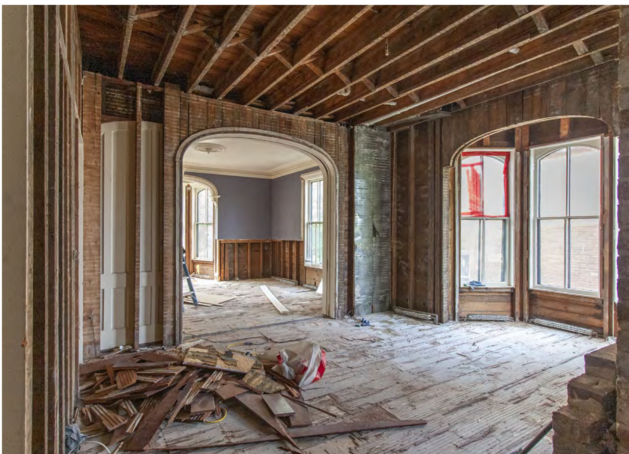
MAIN HOUSE - INTERIORS (DURING ONGOING WATER DAMAGE DEMOLITION)
