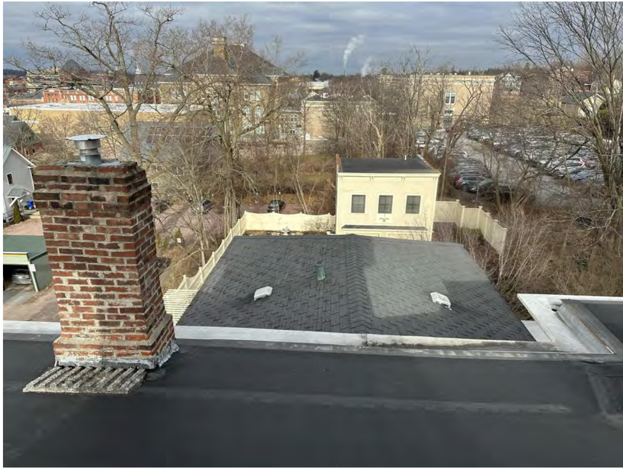
CARRIAGE BARN - SOUTH FACADE/ROOF (LOOKING NORTH)
