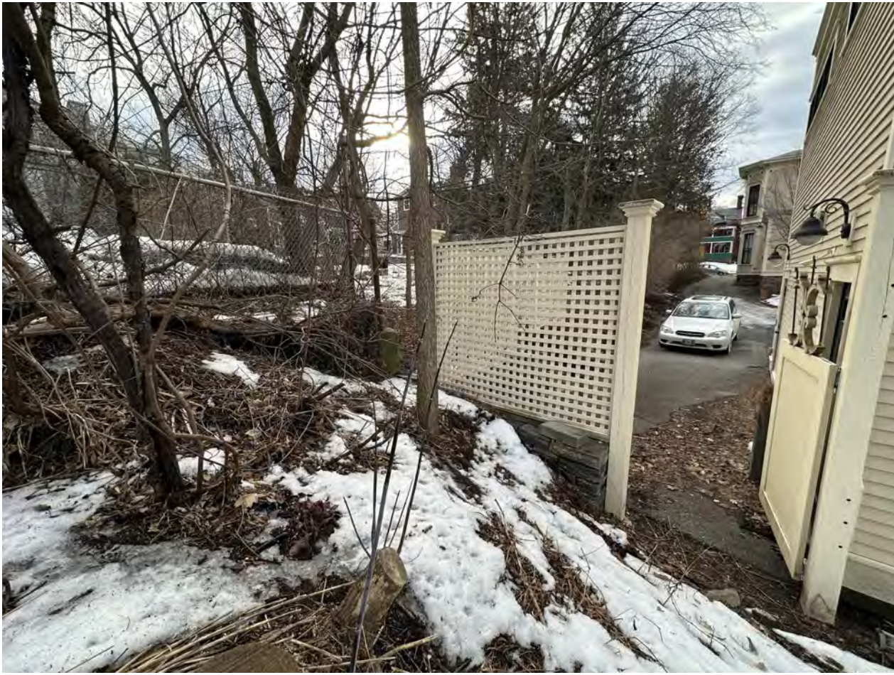
CARRIAGE BARN - NORTHEAST PROPERTY BOUNDARY (LOOKING SOUTH)
