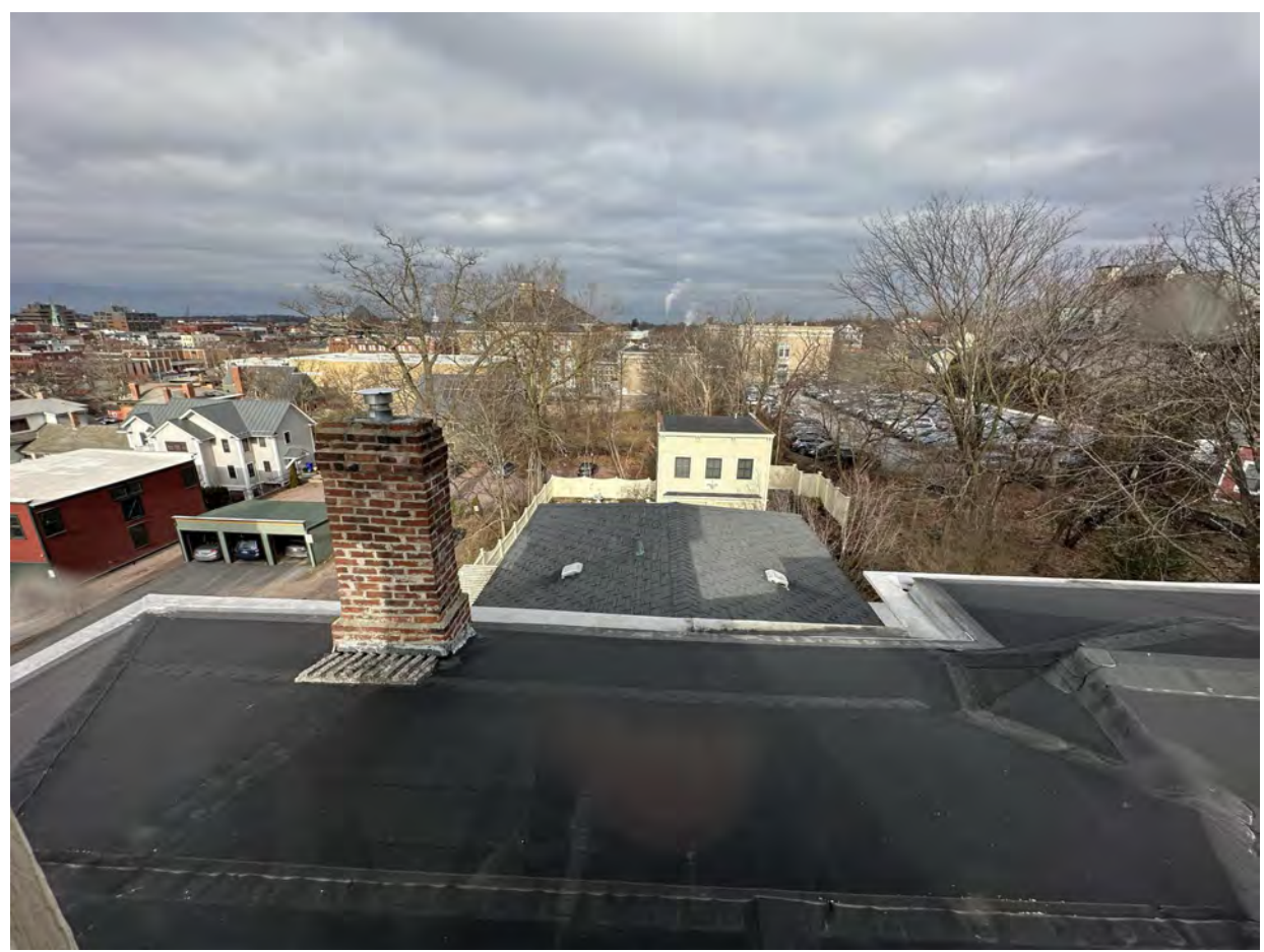
MAIN HOUSE - UPPER ROOF (LOOKING NORTH FROM CUPOLA)
