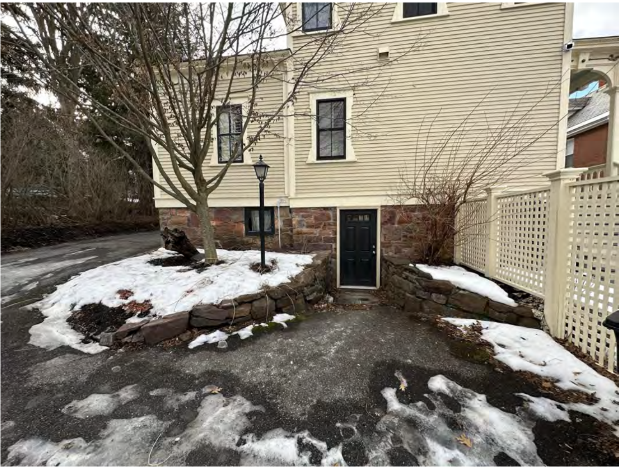
MAIN HOUSE - NORTH FACADE (LOOKING SOUTH)
