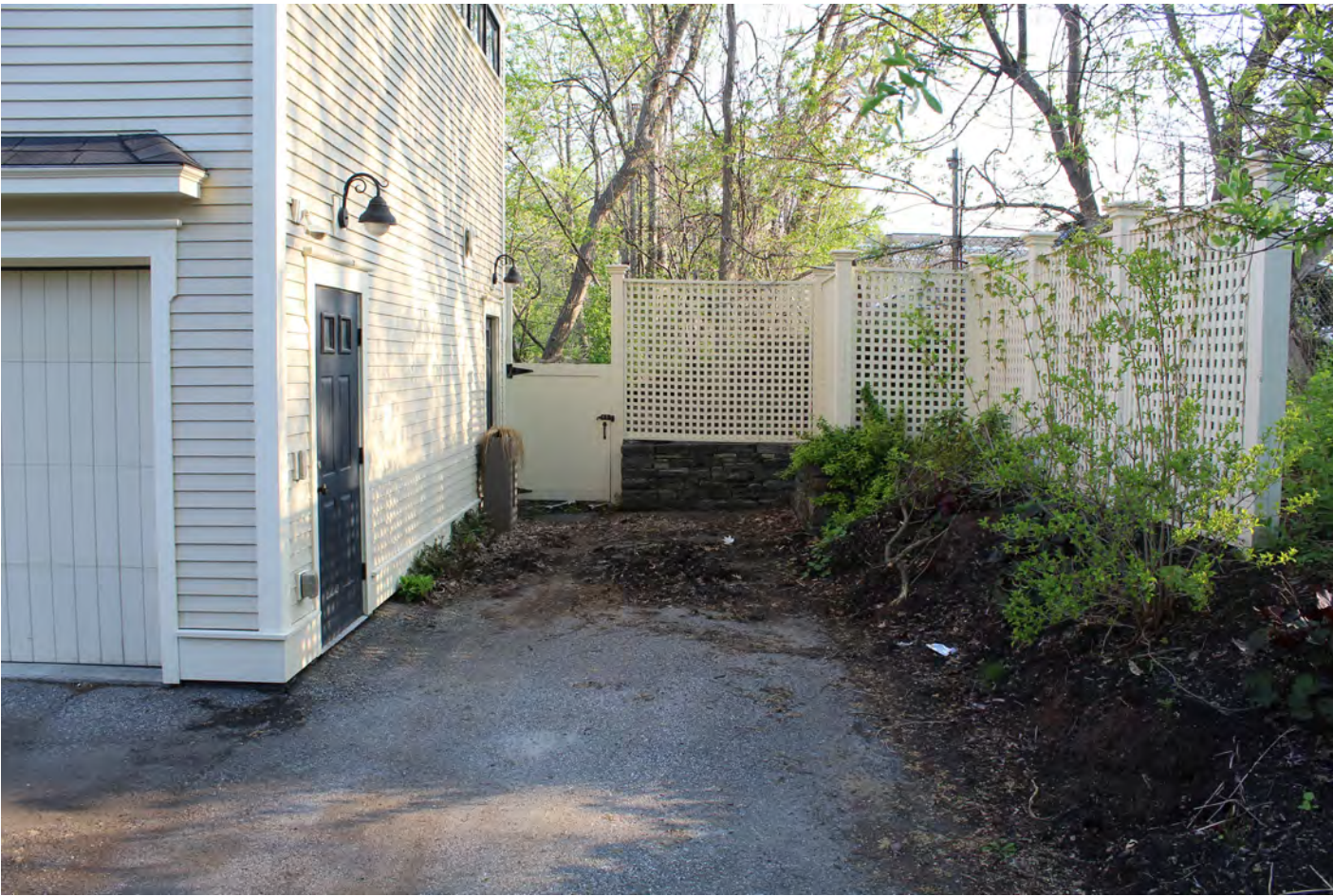
CARRIAGE BARN - EAST FACADE RETAINING WALL & PRIVACY FENCE
