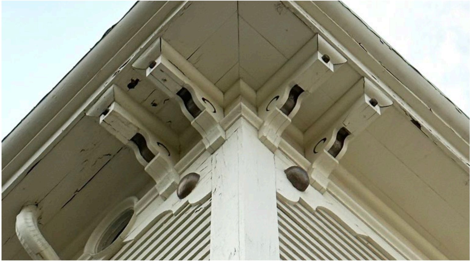
SOFFIT, BRACKETS & INTERNAL DOWNSPOUT
