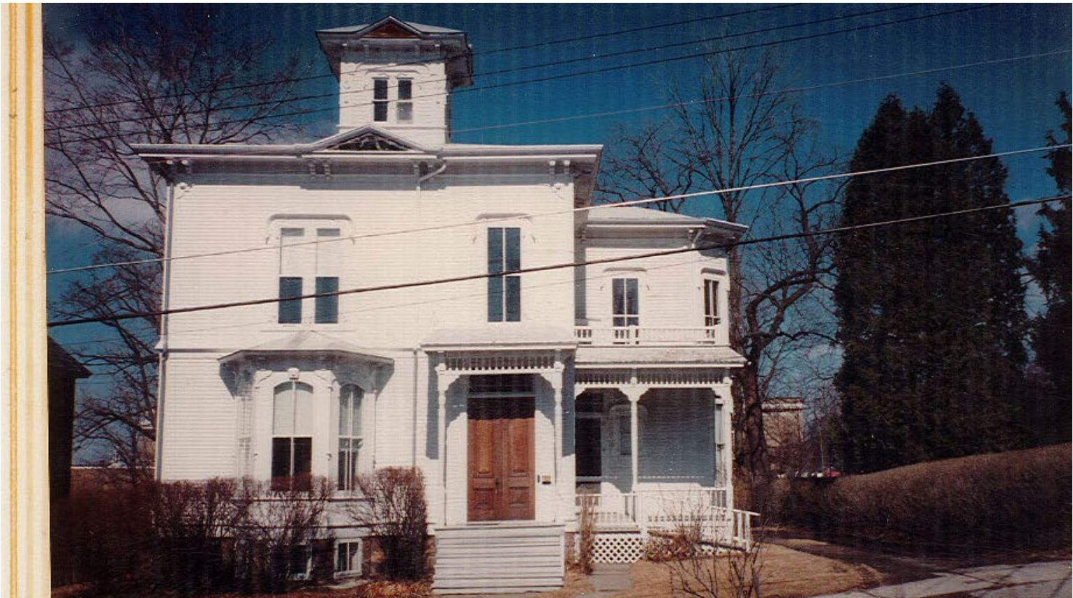
SOUTH FACADE ON MAPLE STREET
