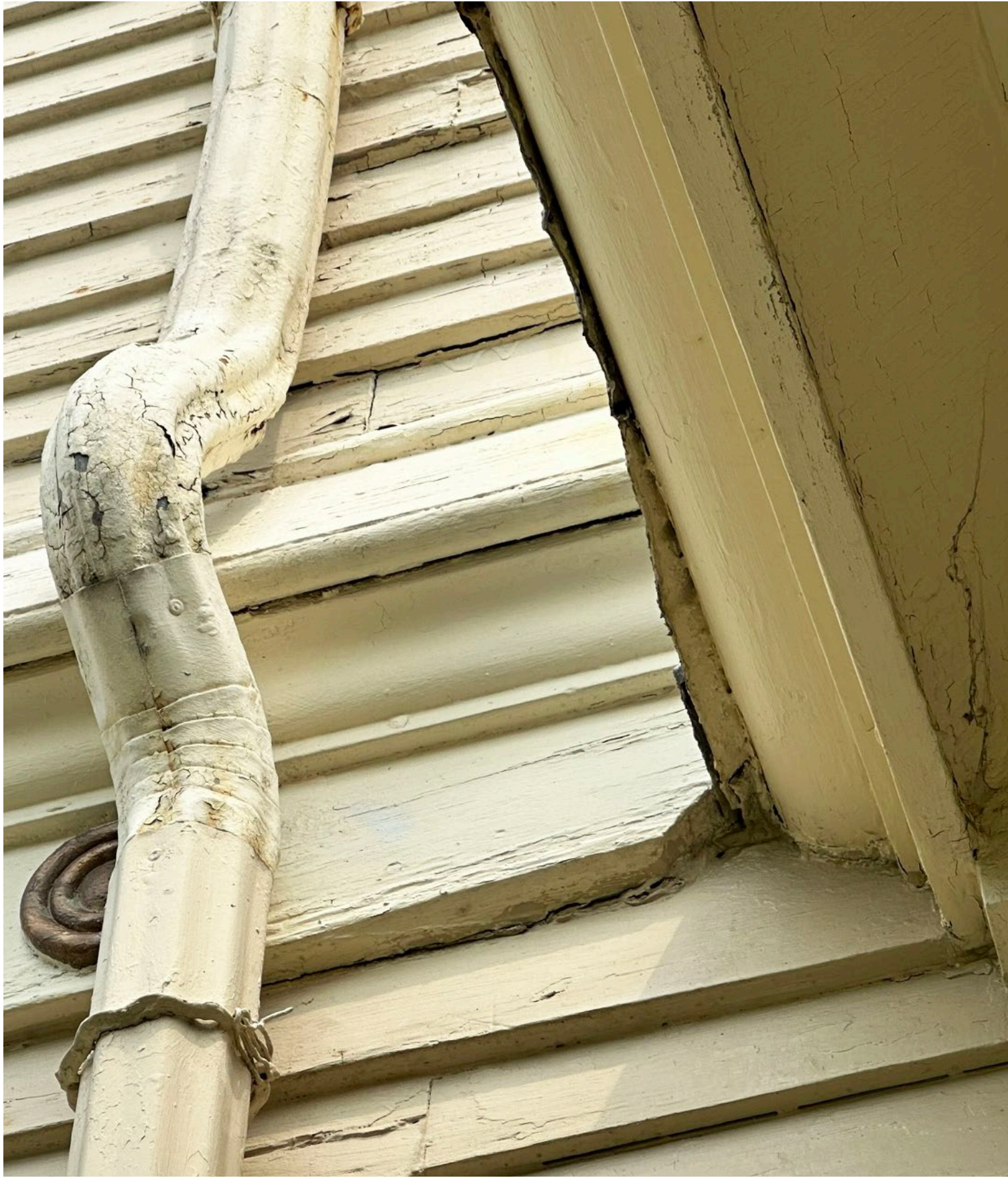
DOWNSPOUT & HORIZONTAL TRIM EXISTING SITE PHOTOS // Main House - Trim & Gutter Downspout conditions
