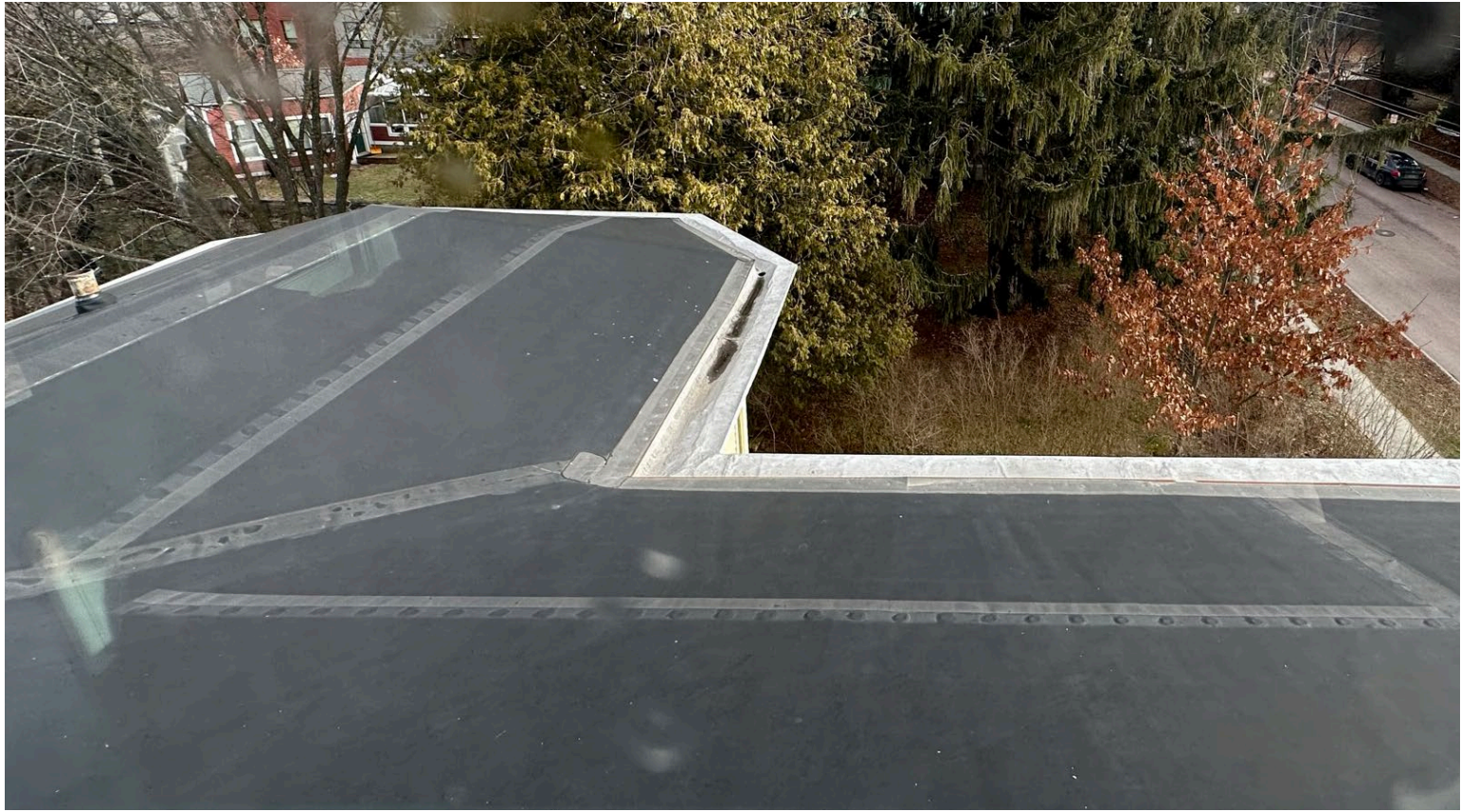
UPPER EPDM ROOF WITH INTEGRATED GUTTERS
