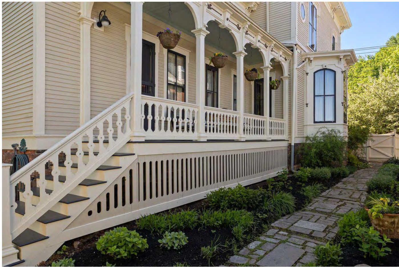
MAIN HOUSE - WEST PORCH (LOOKING SOUTH)
