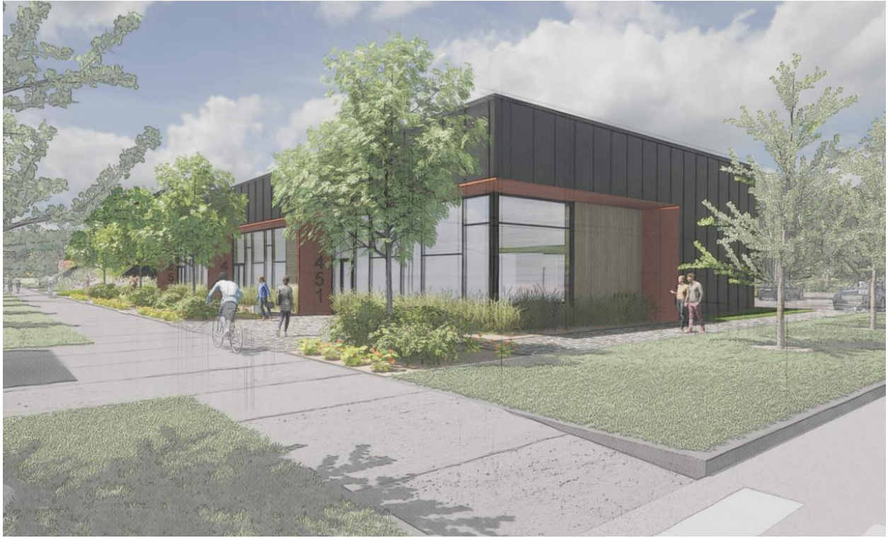
The commercial building, looking southwest. Building fronts Pine Street.
