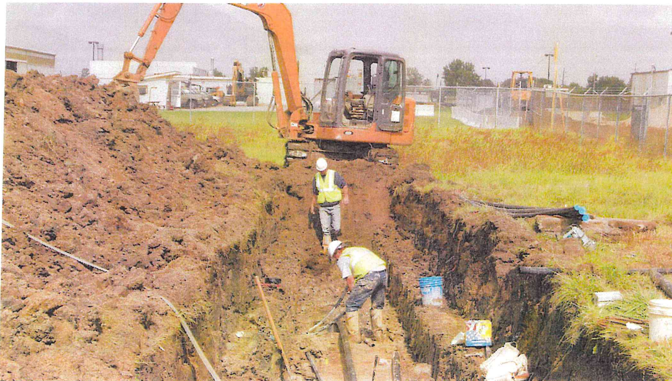
Workers prepare to splice a "T" pipe while installing a geothermal system at Selfridge Air National Guard Base, Michigan, September 29, 2011. (Department of Air Force photo by John Swanson)
