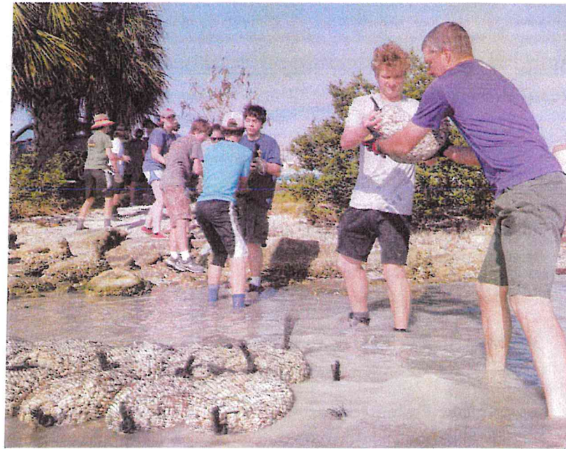
Members of MacDill Air Force Base and the local community build oyster reefs at MacDill Air Force Base, Florida, March 30, 2018. MacDill's eastern shoreline is prone to erosion, however oyster reefs aid in stabilizing the shoreline as well as improving MacDill's vast natural habitats. This build is part of the ongoing Oyster Reef Shoreline Stabilization project, which started in 2004. (Department of the Air Force photo by Staff Sgt. Teri Long)
