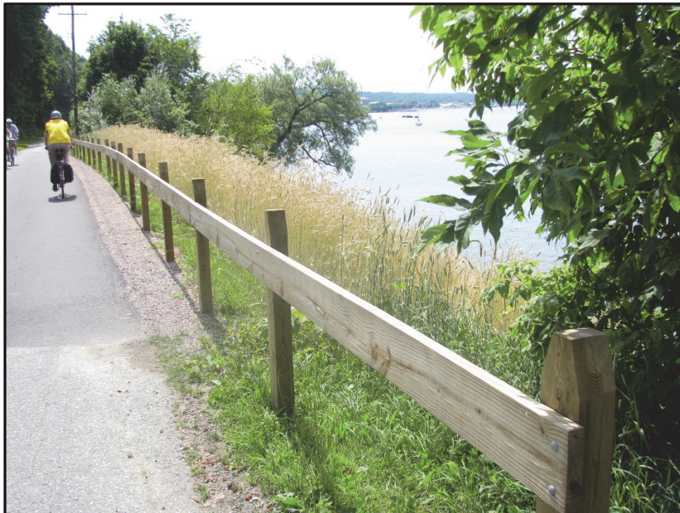
Photo 12. View of non-standard bicycle railing along west side of Bike Path. View is to the southwest.
