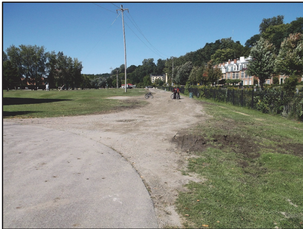
Photo 8. Existing gravel road where Bike Path is to be realigned through the Event Grounds section of Waterfront Park. View is to north.
