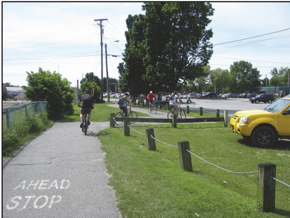
Photo 4. Right angle in Bike Path alignment. Initially aligned to allow for crossing old railroad rails at right angle. View is to south.
