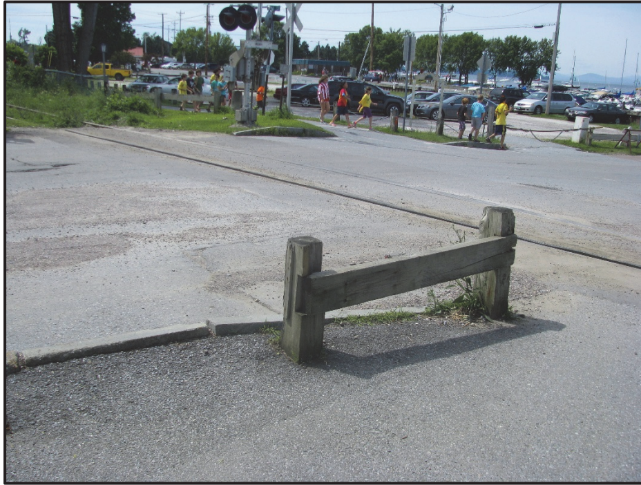
Photo 5. Current Bike Path alignment encouraging crossing railroad tracks at angle. View is to the southwest.
