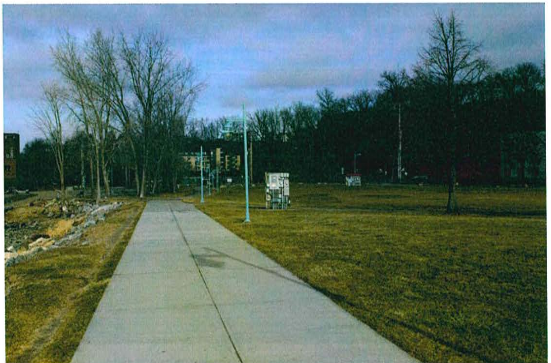
Photograph 4: View of backboard and electrical panels, west side of Event Grounds at intersection of Bike Path and sidewalk. (VHB, 12/4/13)
