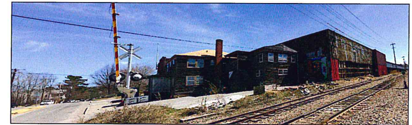
VIEW: WEST ELEVATION FROM FLYNN AVE (Buildings 1&6)
