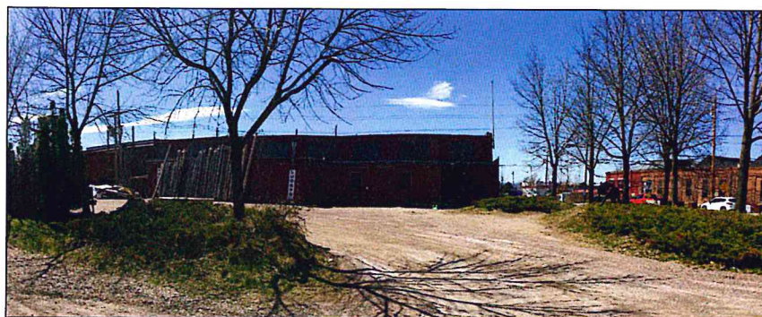
VIEW: EAST ELEVATION FROM BRIGGS STREET (Buildings 4&5)
