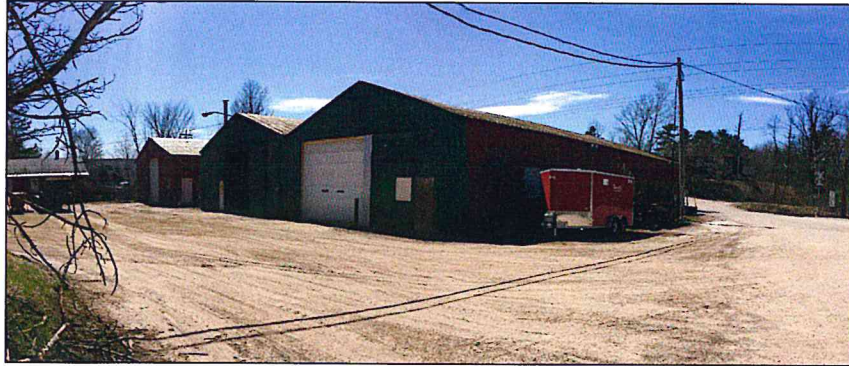
VIEW: EAST FACADE FROM BRIGGS STREET (Buildings 7&8)
