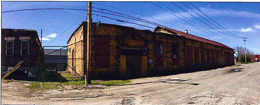
VIEW: EAST ELEVATION FROM BRIGGS STREET (Buildings 2&3)
