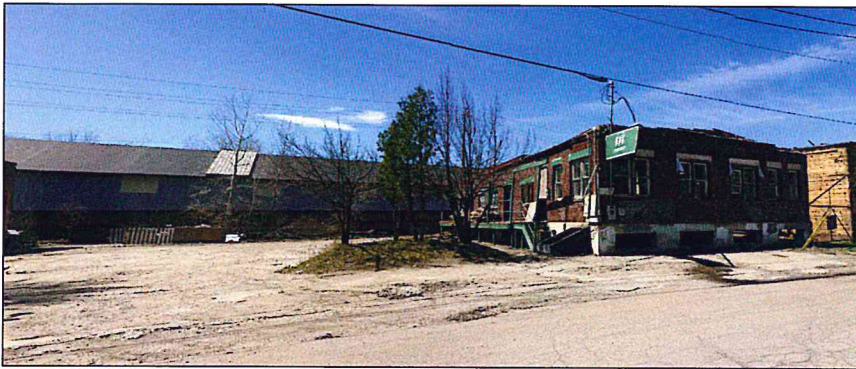
VIEW: EAST ELEVATION FROM BRIGGS STREET (Buildings 6&9)
