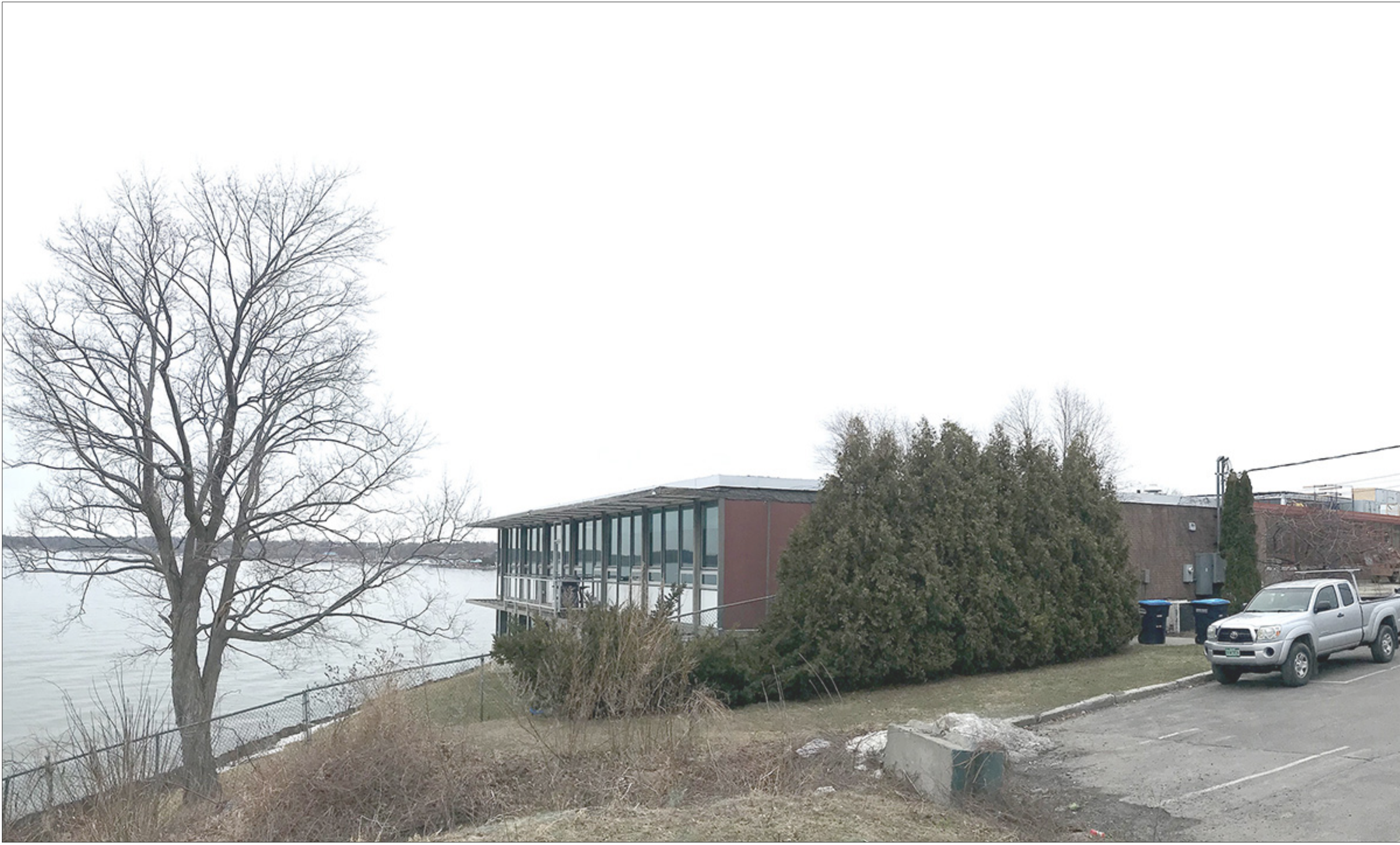
VIEW FROM SOUTHWEST
