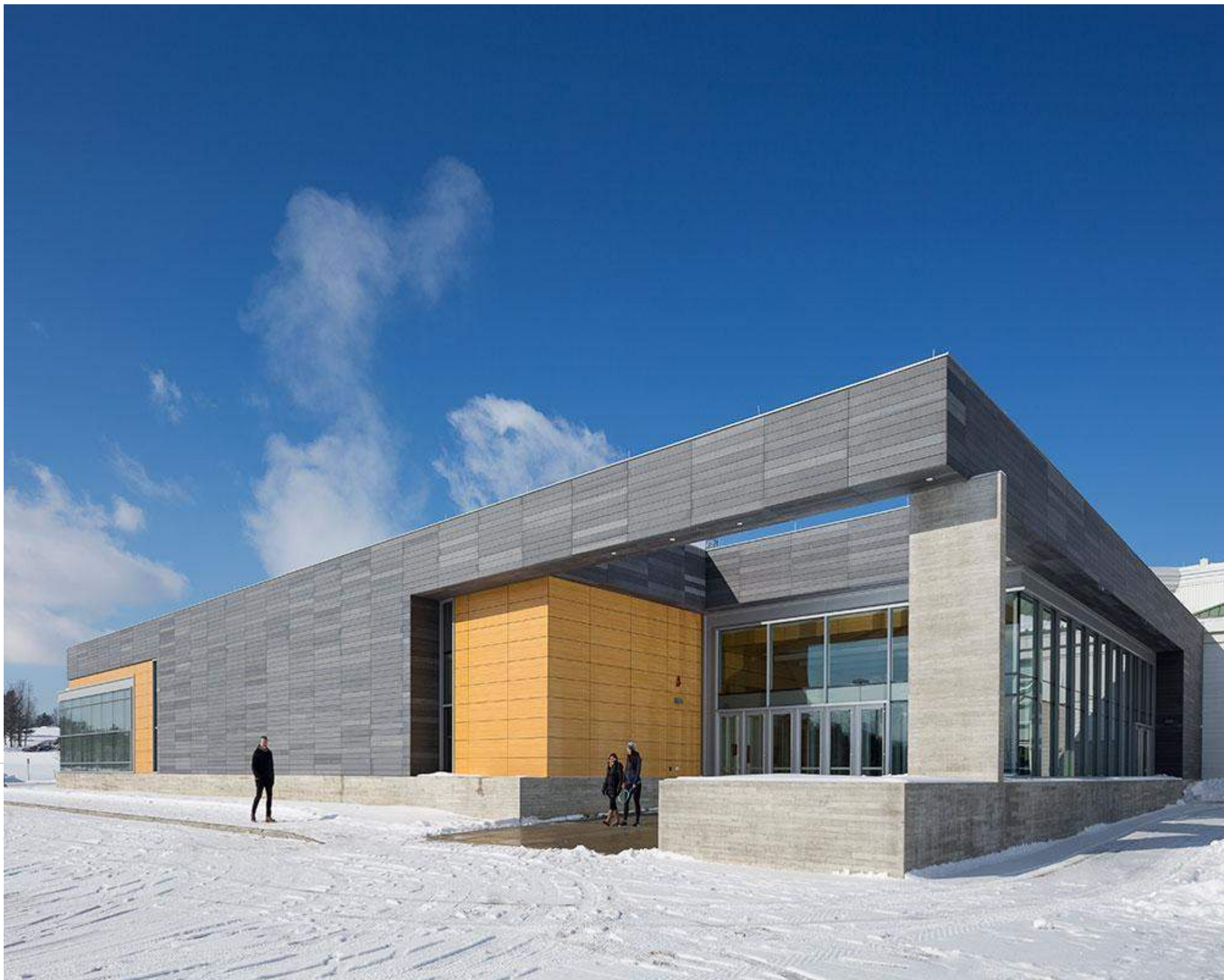
FACADE SLATS MADE OF GLASSFIBRE REINFORCED CONCRETE
