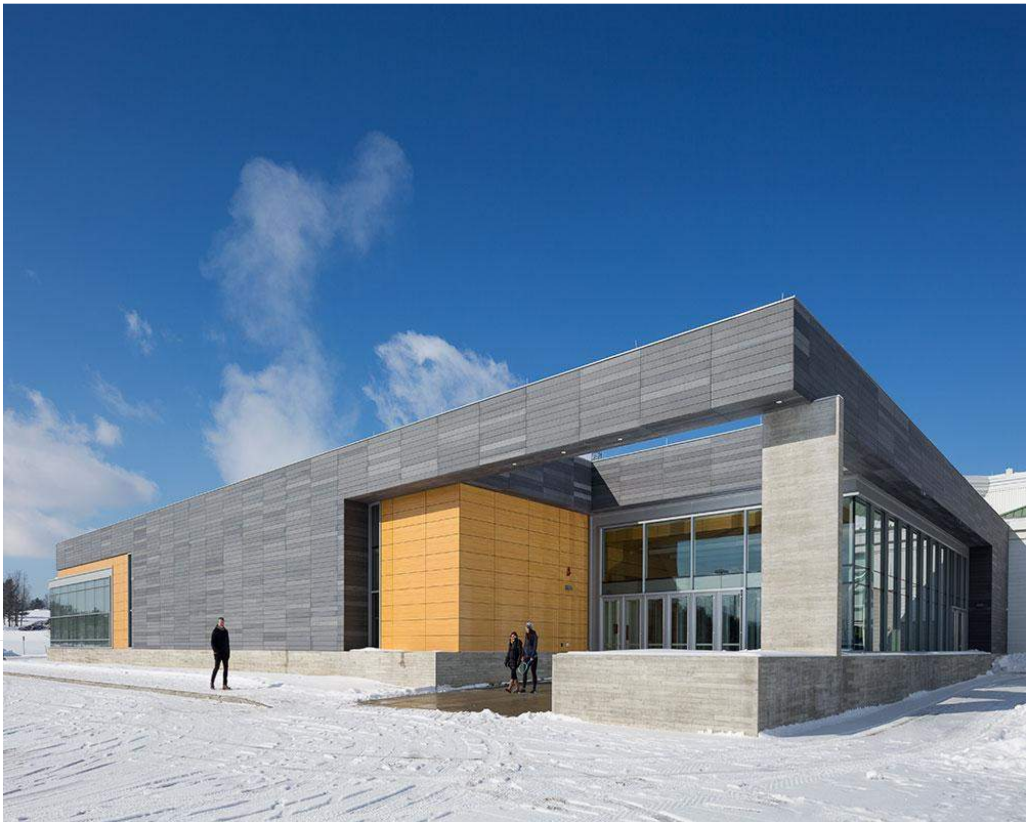
FACADE SLATS MADE OF GLASSFIBRE REINFORCED CONCRETE
