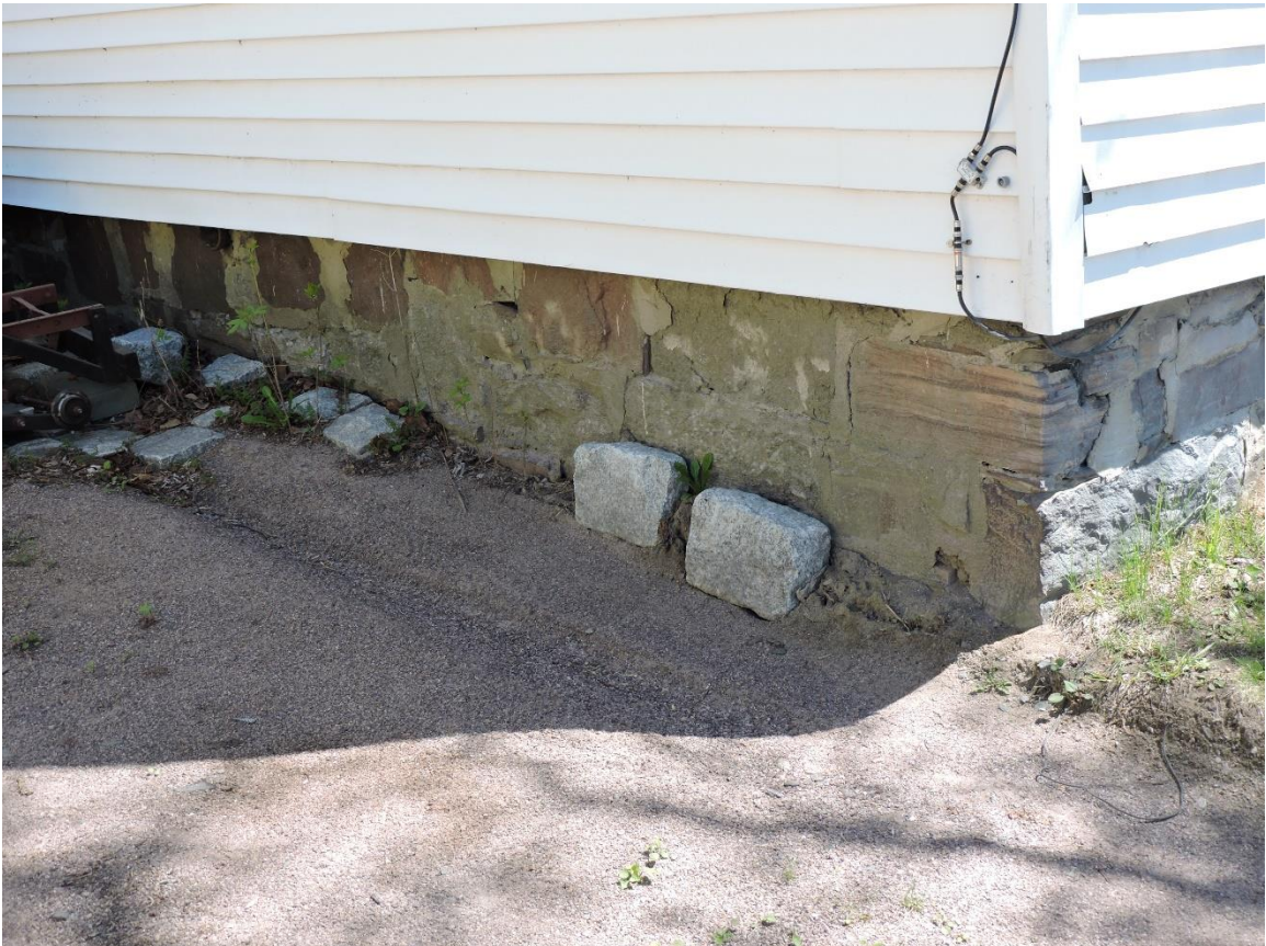
6. View southeast at stone foundation.
