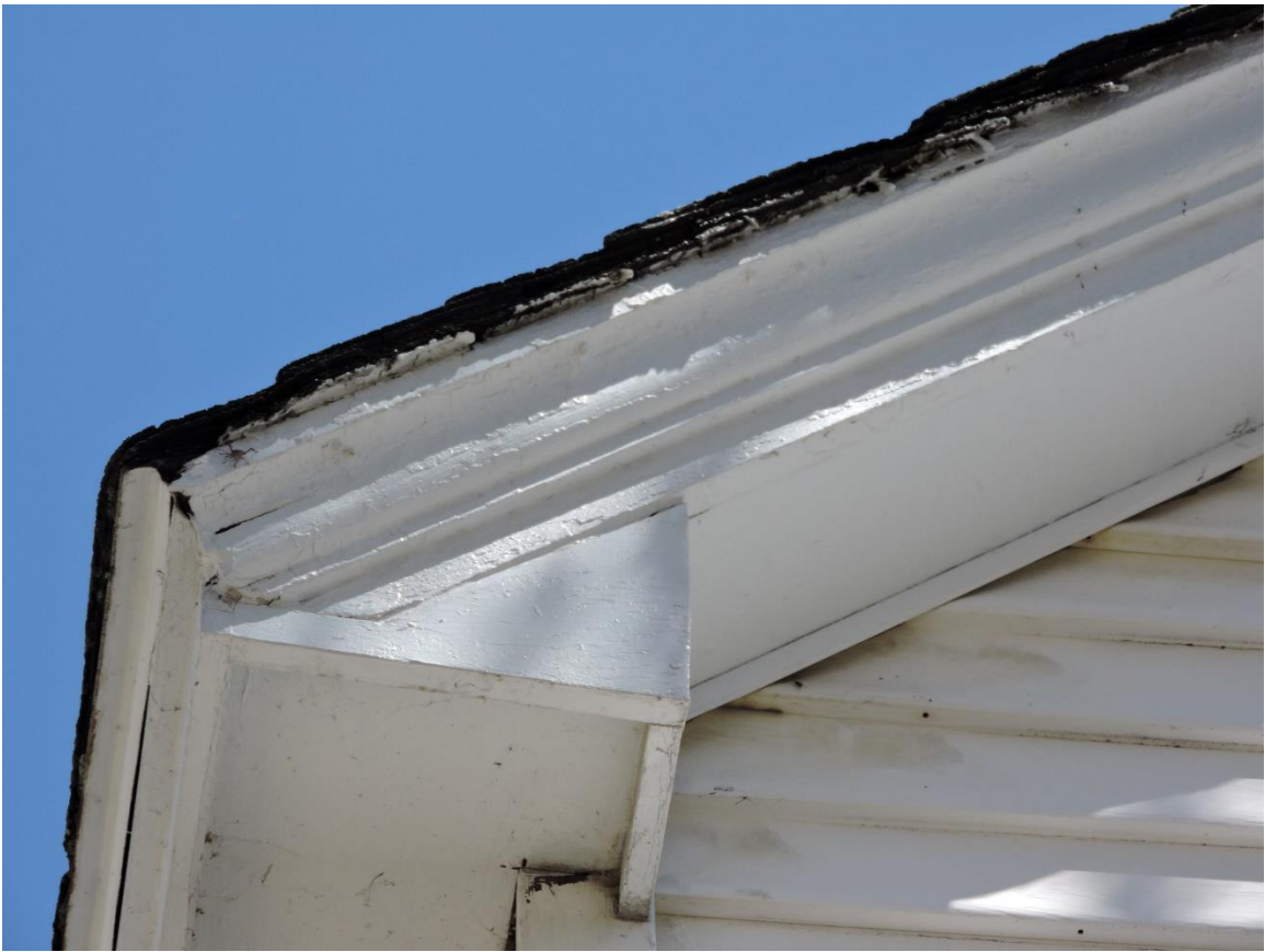
5. View east of molded cornice on front eave.
