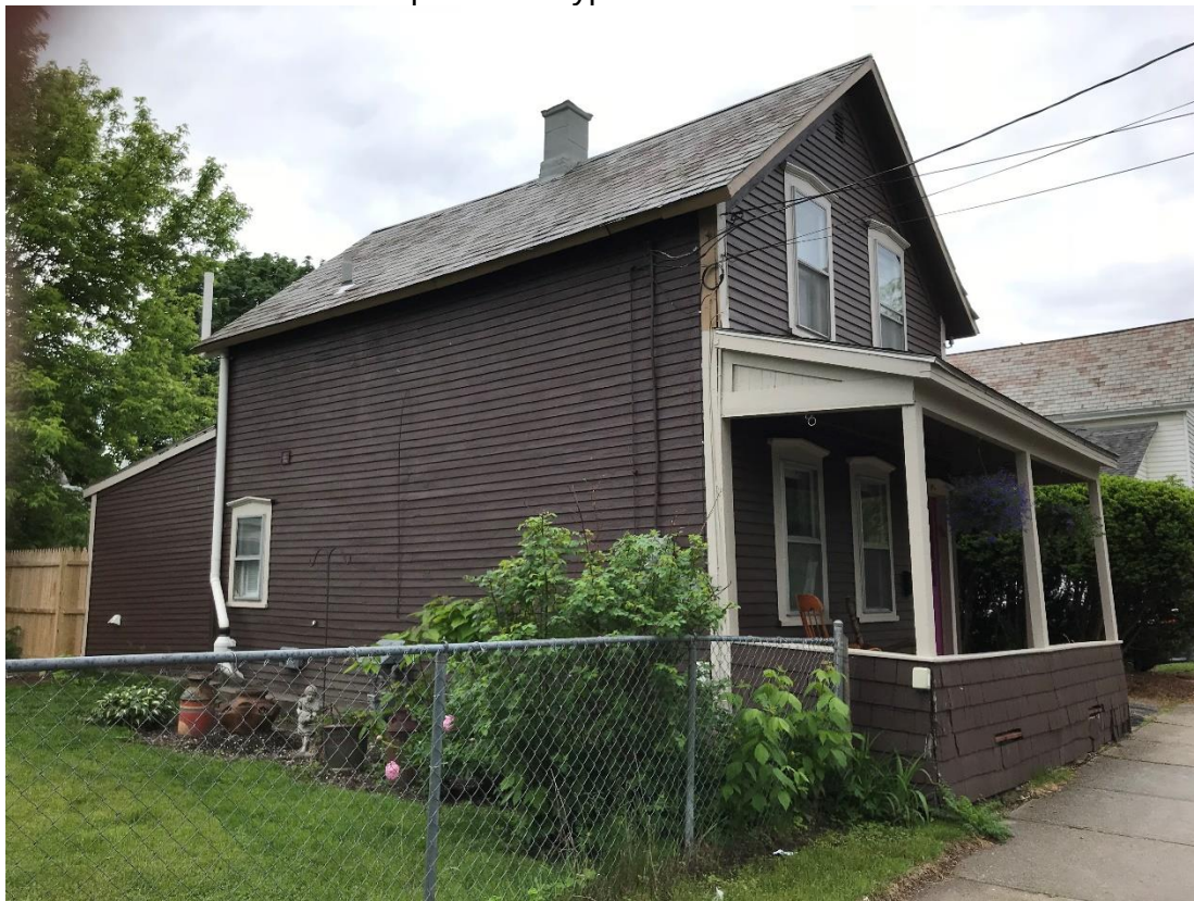
9 Convent Square front (north) and east sides with shed roof rear addition commonly found in the neighborhood. This house appears to be an intact example of the house type seen at the subject building at 36 Convent Square. Front proc is an early 20 th century addition.
