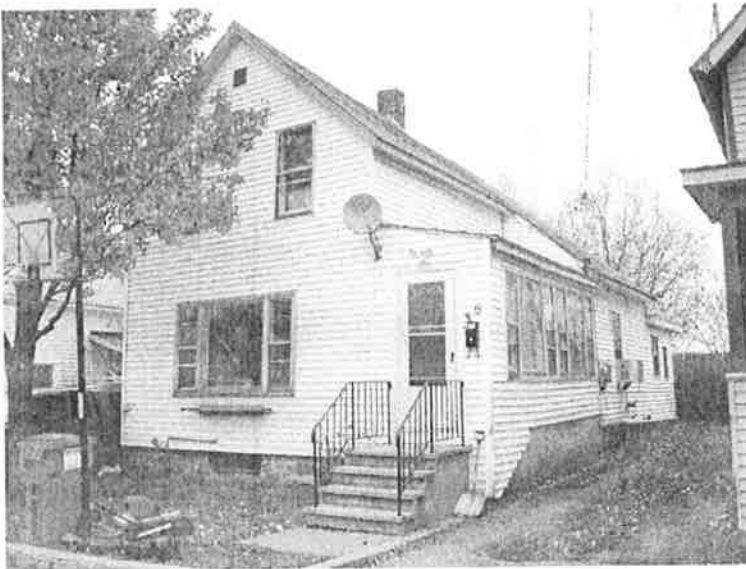
View of front elevation looking easterly.
