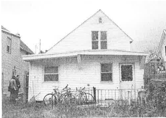
Rear elevation, showing non-historic rear addition.
