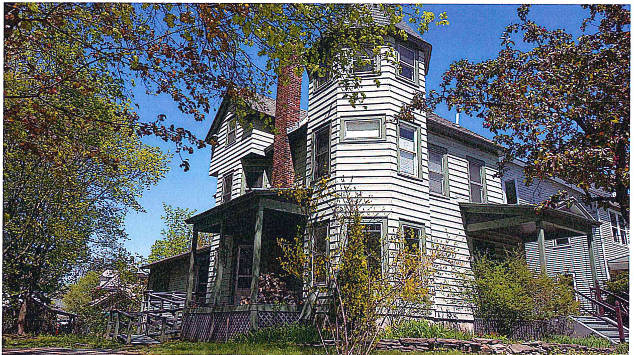
16 Wilson Street – view from street.
