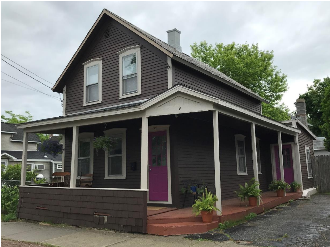
9 Convent Square front and west sides with typical single story shed roof addition projecting beyond plane of main block.
