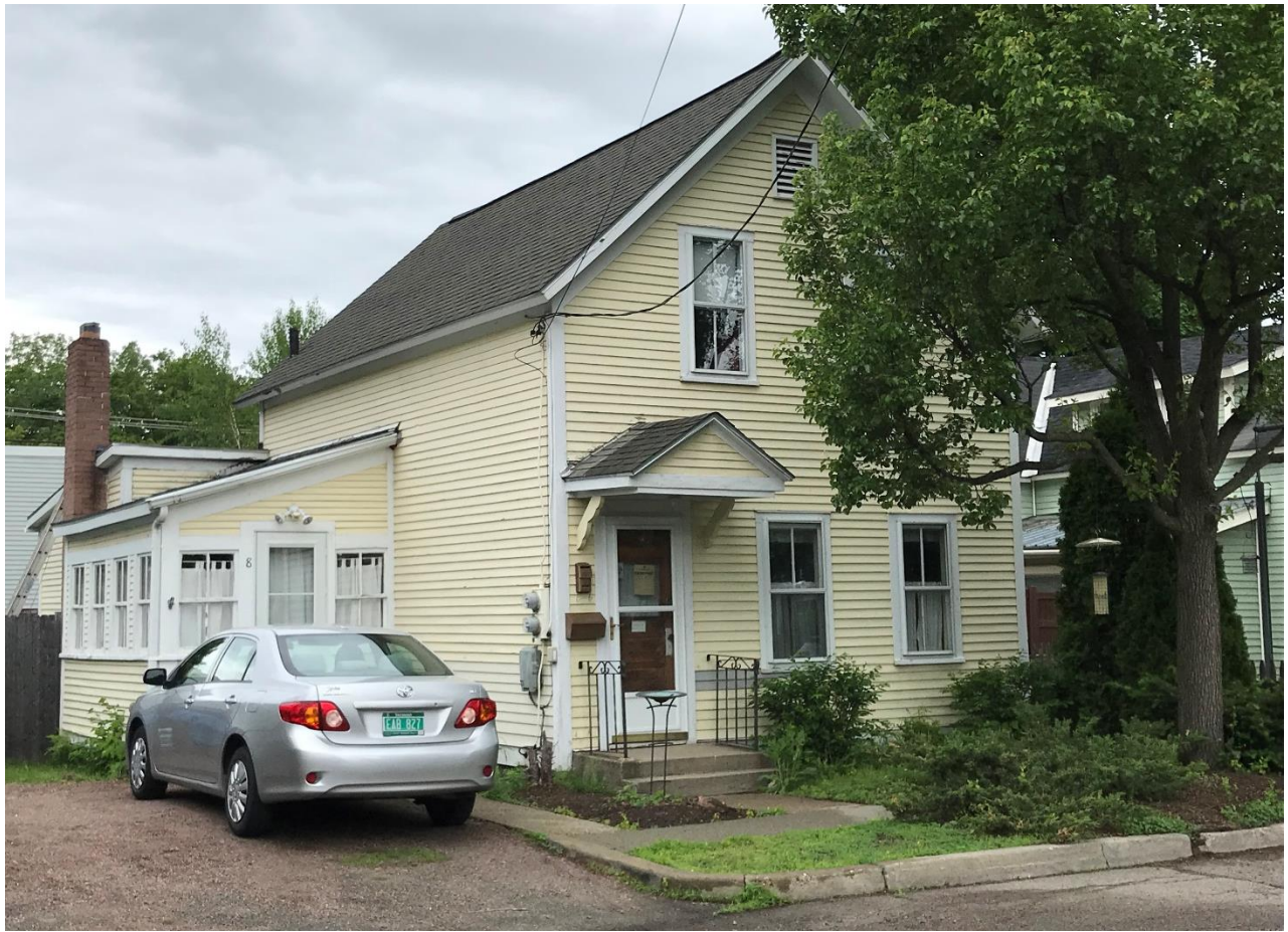
8 Convent Square with single-story shed roof rear addition common in neighborhood.
