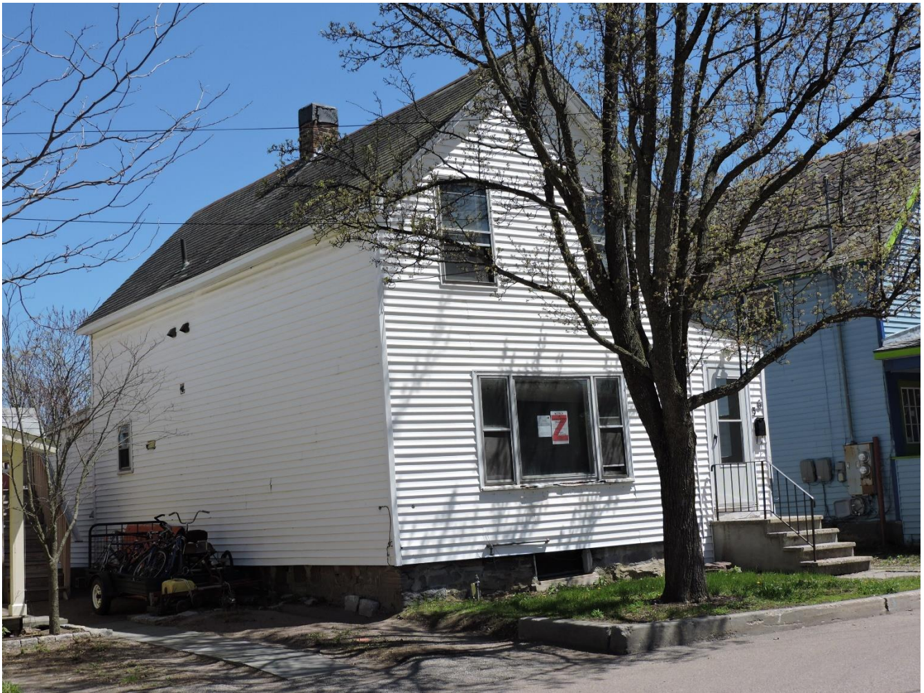
2. View east of front and north sides with windows likely removed.
