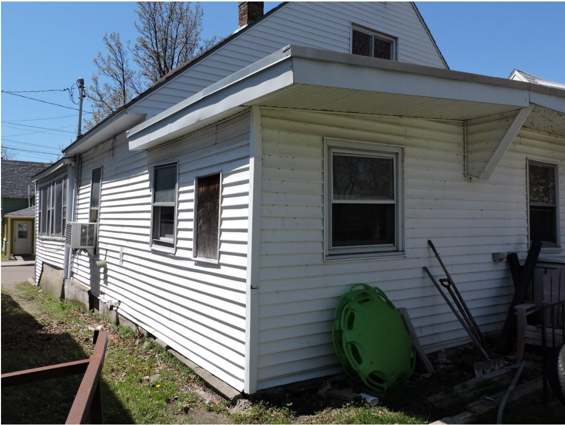
3. View west of back (east) and south sides.
