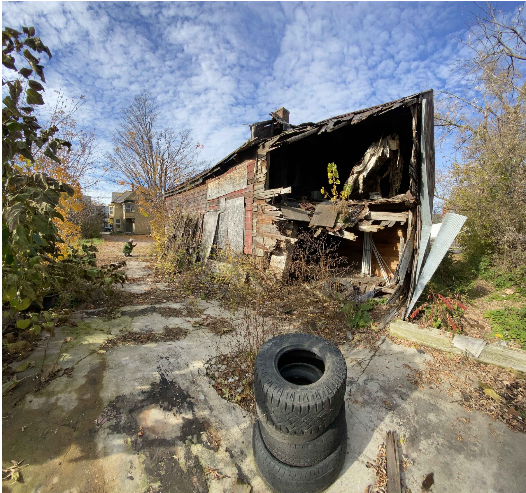
PHOTO 4 - VIEW FACING NORTHWEST
