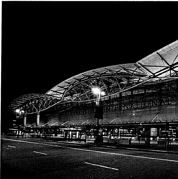
ROADWAY AREA LIGHTING
