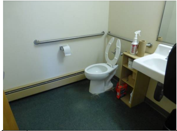
Photo #14: First floor restroom
