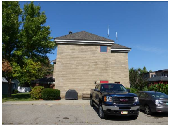
Photo #4: Rear elevation
