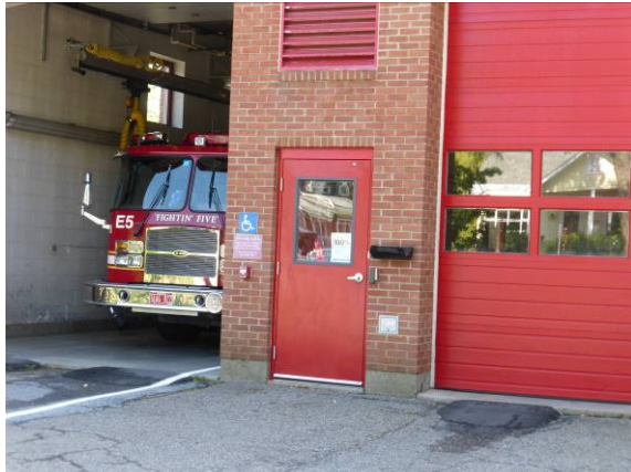
Photo #7: Exterior doors
