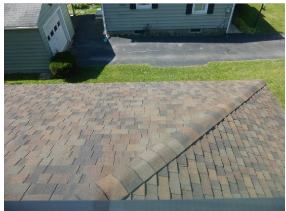
Photo #12: Roofing detail
