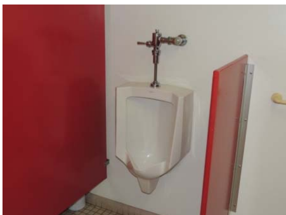
Photo #23: Second floor restroom located in living quarters
