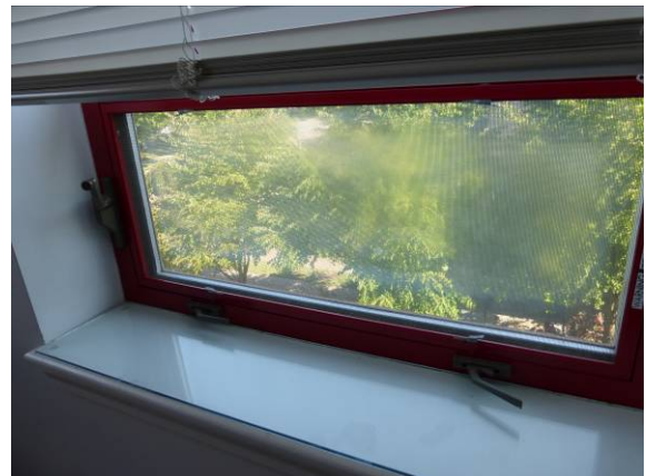
Photo #28: Window detail
