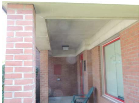
Photo #34: Porch lighting at main north elevation
