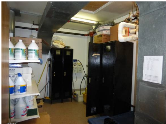
Photo #17: Storage and mechanical room
