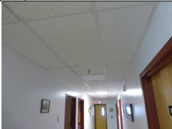
Photo #29: Ceiling detail
