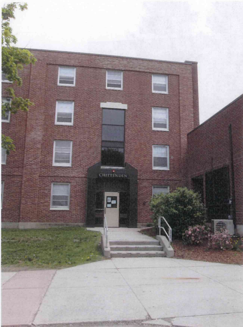
Chittenden, South Entry on West Façade
