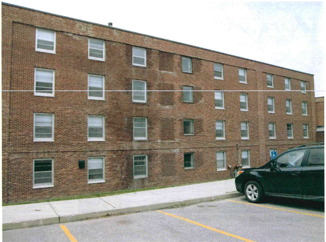
Buckham, East Façade
