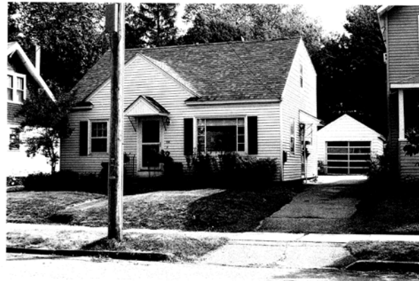
Survey 0402-5: 114 Charlotte Street Burlington, VT. View northeast. Photograph by Devin Colmar, 9/5/2007 Digital image on file at VT Division for Historic Preservation
