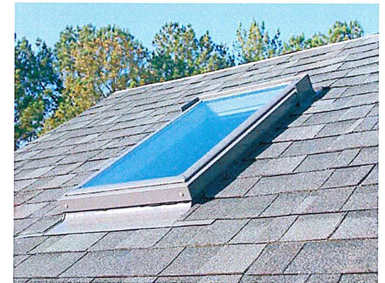
EXAMPLE: VELUX DECK MOUNTED SKYLIGHT
