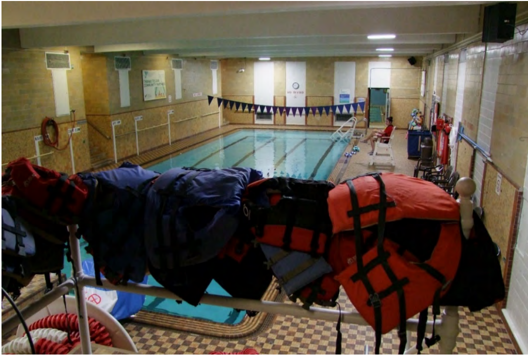
Photograph 33: Interior of the existing, basement-level pool in the 1934 gymnasium/ pool wing. Note the contrasting tile in the former window openings. This wing is proposed to be replaced by the new addition and two levels of underground parking.
