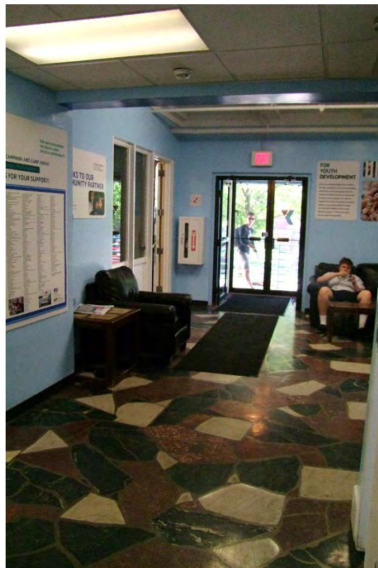
Photograph 26: Interior of main lobby accessed via College Street entrance at center. The interior will be remodeled, although this entrance will remain.
