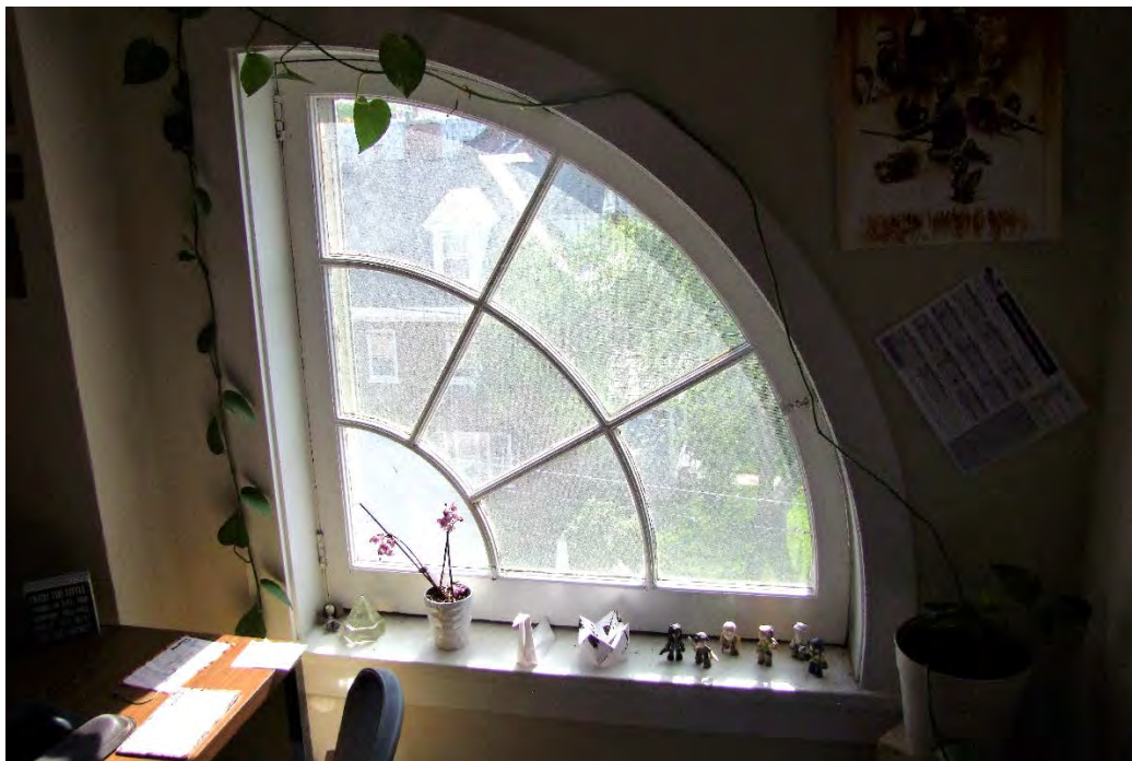
Photograph 40: Interior of an existing office on the fourth floor in the east portion of the main south block of the YMCA. The existing quarter fanlight will be preserved.
