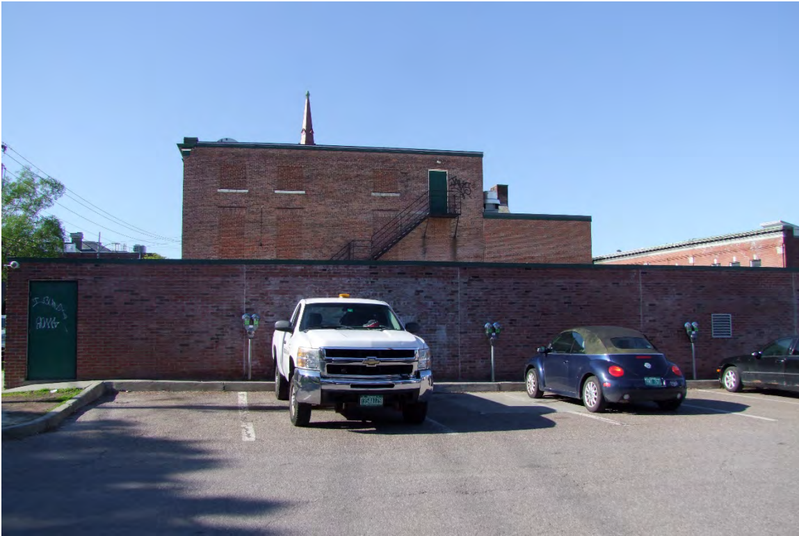
Photograph 13: North elevations of the 1934 and 1984 pool/ gymnasium wings. Note the infilled windows on the north façade of the gymnasium. Beyond is the College Street Congregational Church steeple.
