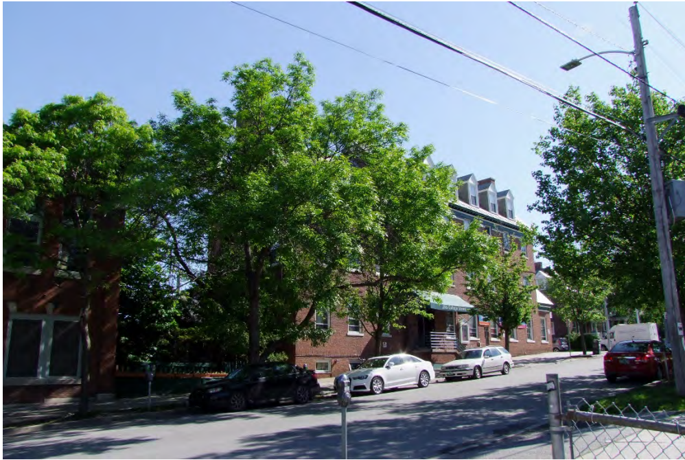
Photograph 1: South elevation of YMCA building.
