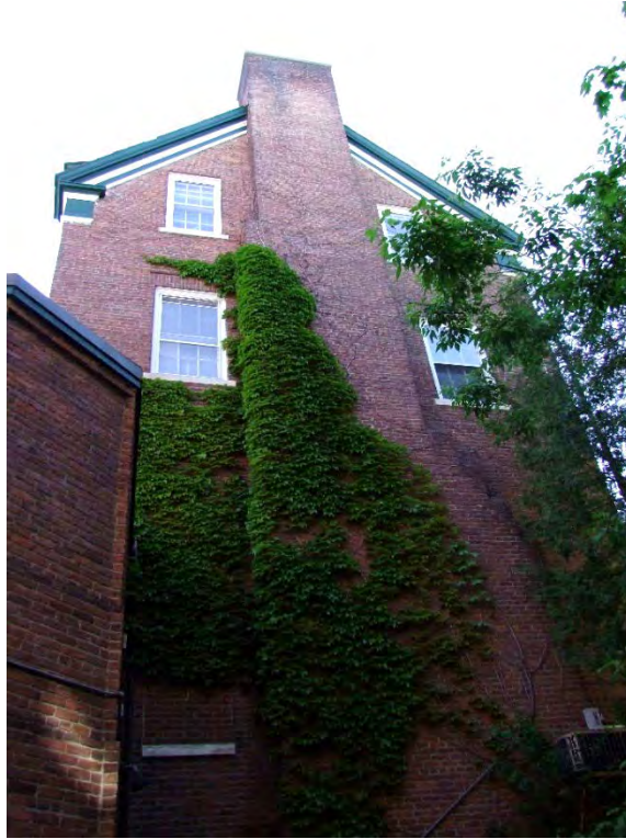
Photograph 23: View of the upper west elevation of the south block of the building. The new addition will extend north from about the middle of the existing exterior chimney.
