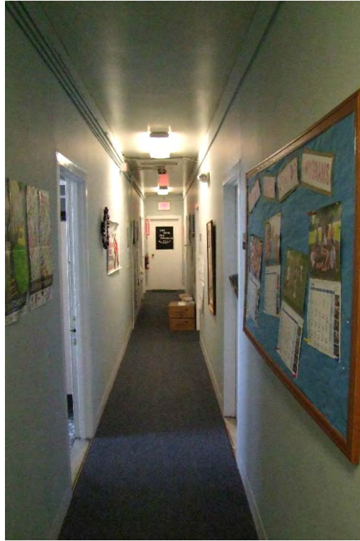
Photograph 39: Representative interior hallway within the main south block of the YMCA building. This portion of the building, which historically contained boarding rooms, will be preserved and converted into apartments.
