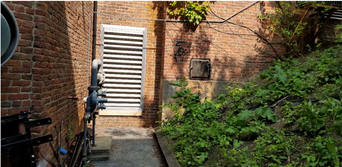
Photograph 22: View of the west elevation of the south block of the building. The exterior chimney, visible at center right, will be retained, and the new addition will extend to the north from the chimney. The entrance to the new underground parking garage will be in this approximate location.
