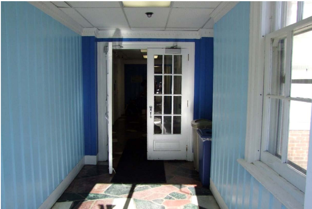
Photograph 24: Interior of the lobby of the east gabled wing. The wing will be retained as the primary entrance, but the interior will be remodeled.
