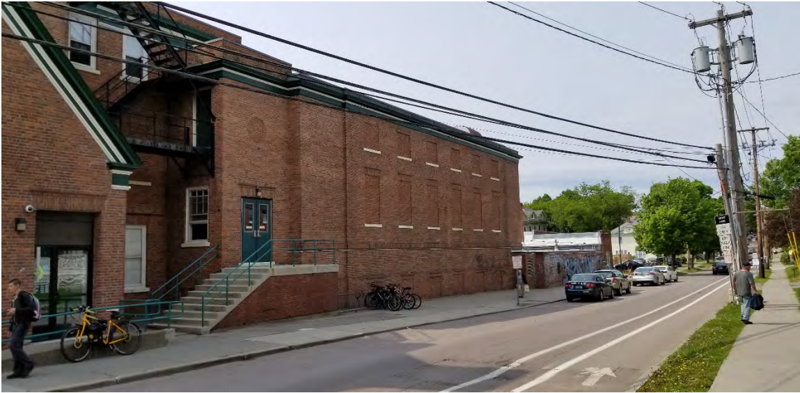
Photograph 11: East elevation of the 1934 gymnasium and pool wing along S. Union Street. The windows were infilled with brick sometime before the mid-1970s. This addition is proposed to be removed and replaced with the new building.
