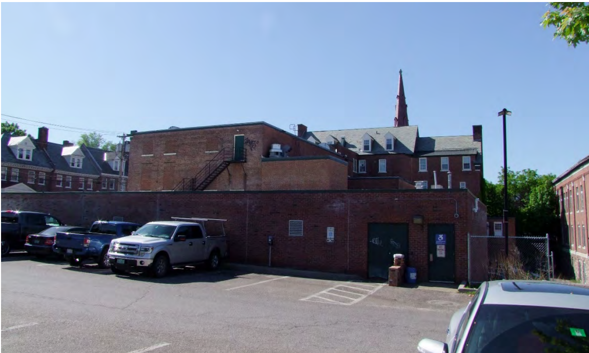
Photograph 14: North elevations of the building, beyond which is the College Street Congregational Church steeple.
