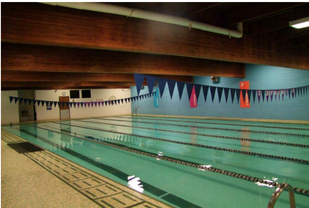
Photograph 34: Interior of the one-story, 1984 north pool wing which is proposed to be replaced by the new addition.
