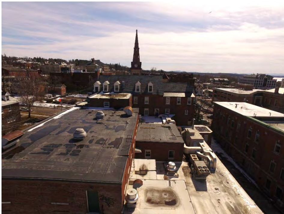
Photograph 44: Birds-eye view of the YMCA building, looking south. Clearly visible are the multiple additions and rooflines of the 1934 pool/ gymnasium addition proposed to be replaced by the new hotel building.
