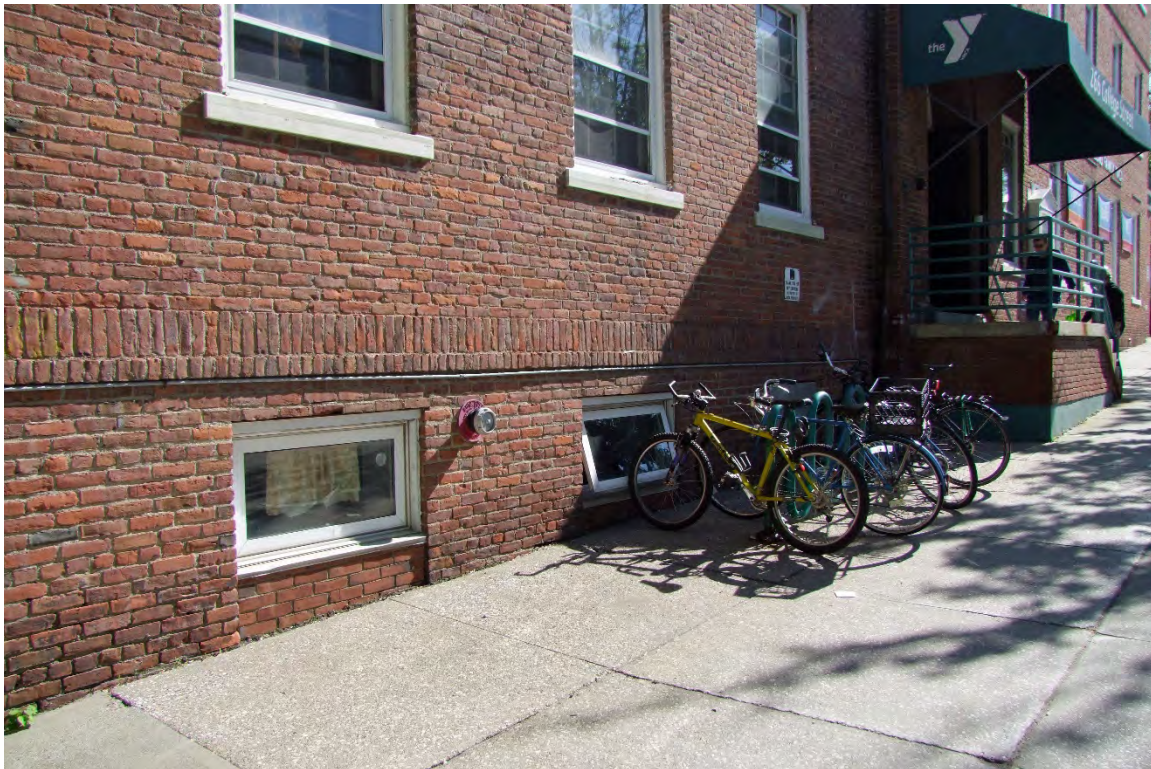
Photograph 6: Detail of replacement windows on basement of south elevation, as well as modern entrance stairs and awning on south elevation
