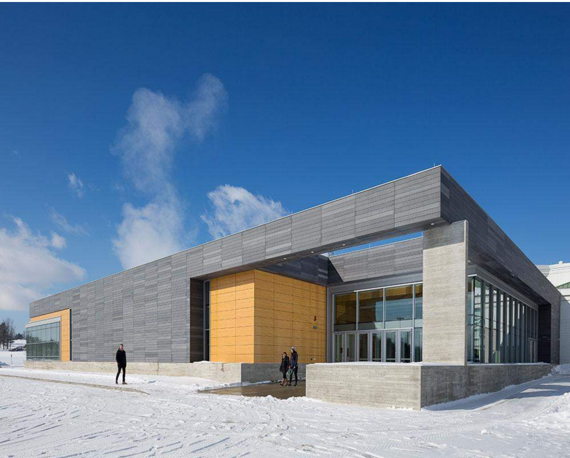
FACADE SLATS MADE OF GLASSFIBRE REINFORCED CONCRETE
