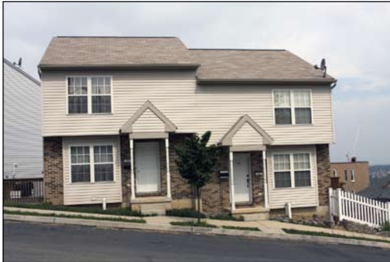
Examples of how sloped topography can affect the location of buildings. Notice how, in each example, the buildings are terraced to provide a flat building pad for the house.
