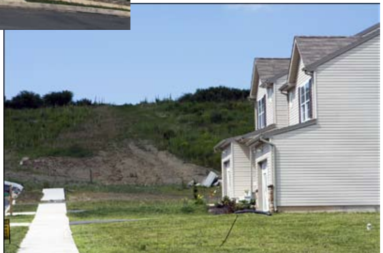
Examples of how sloped topography can affect the location of buildings. Notice how, in each example, the buildings are terraced to provide a flat building pad for the house.
