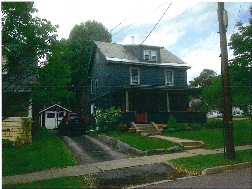
82 Henry St House to the East of site
