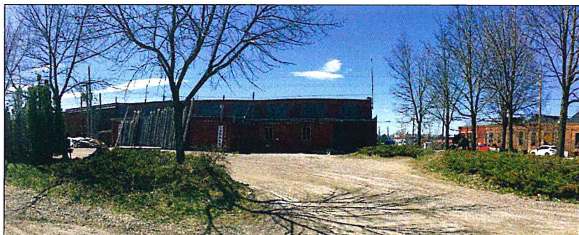
VIEW: EAST ELEVATION FROM BRIGGS STREET (Buildings 4&5)
