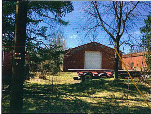
VIEW: EAST ELEVATION FROM BRIGGS STREET (Building 7)
