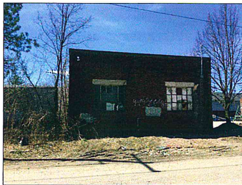
VIEW: EAST ELEVATION FROM BRIGGS STREET (Building 10)
