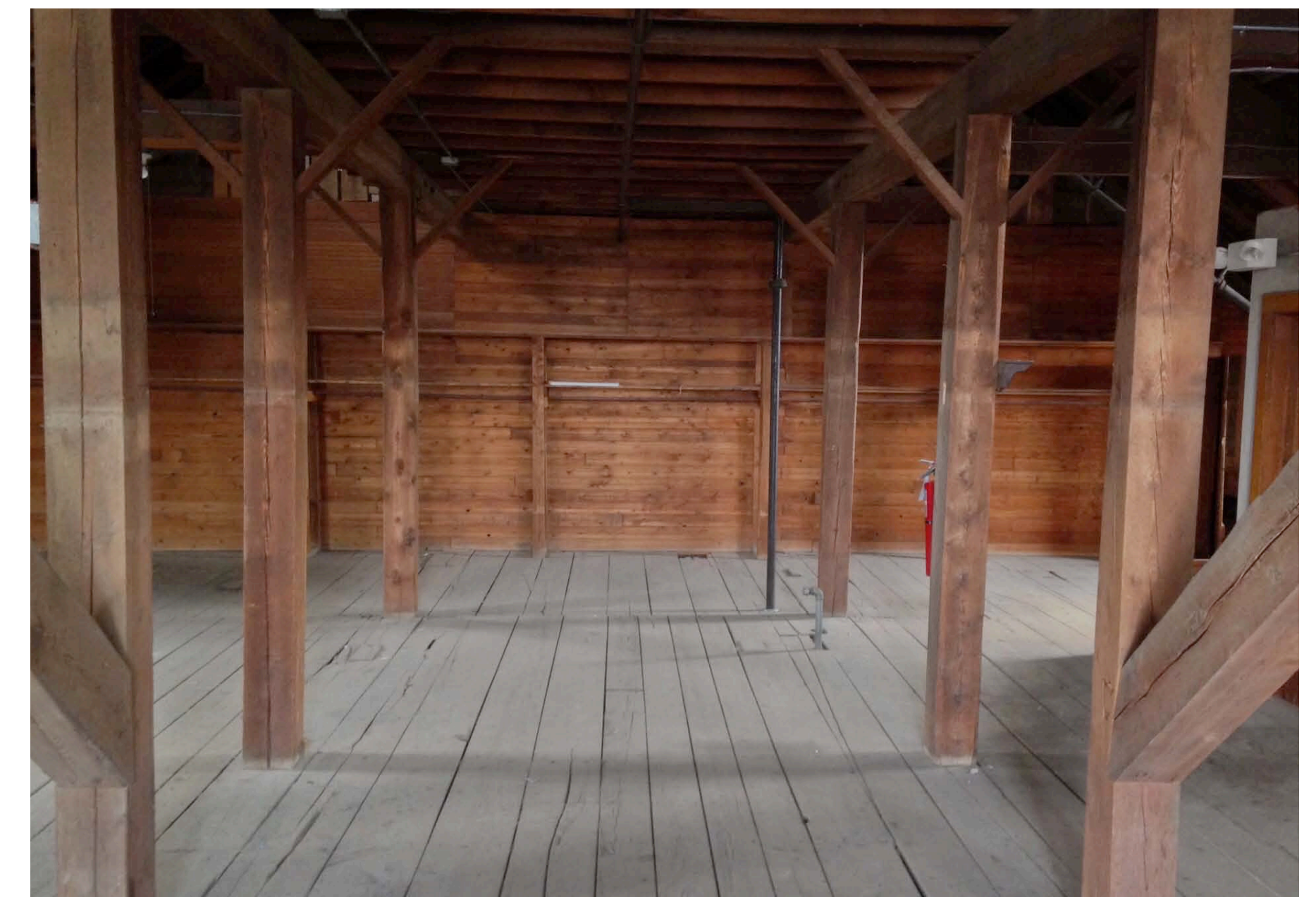
ATTIC LEVEL - BELOW MEZZANINE, NORTH END
