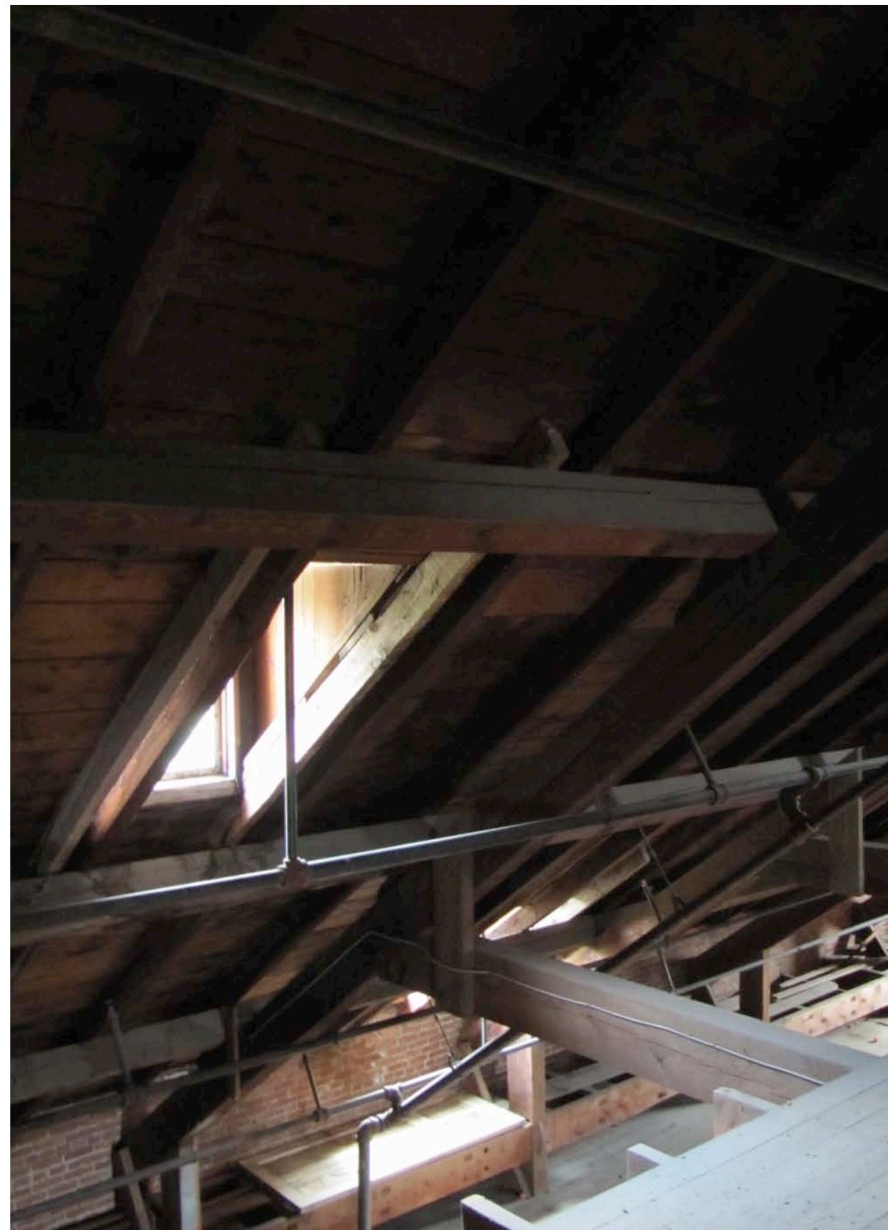
MEZZANINE LEVEL - HIGH DORMER
