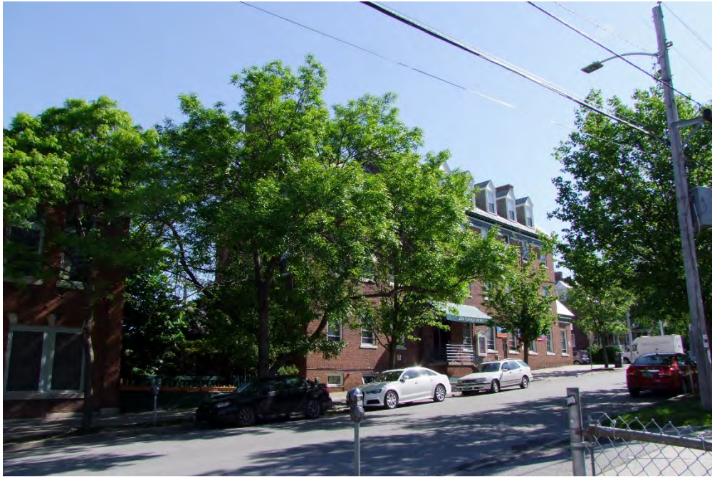
Photograph 1: South elevation of YMCA building.
