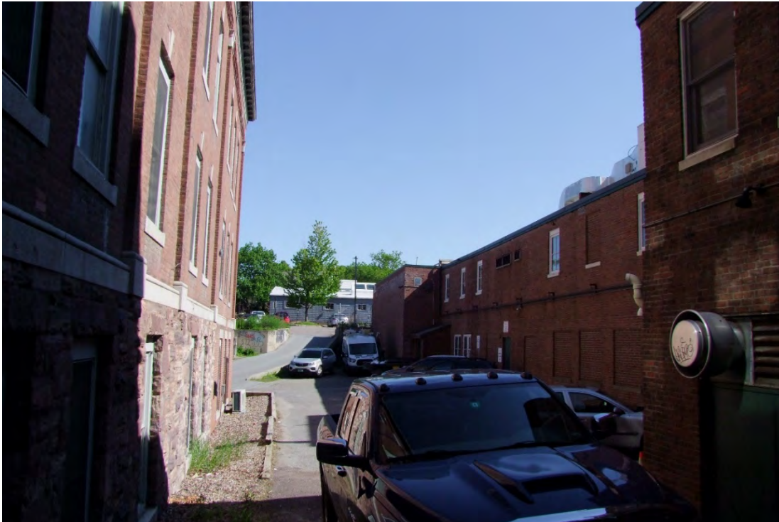
Photograph 17: Existing driveway and parking area along the west façade of the YMCA building. The new building will extend further west than the existing building.
