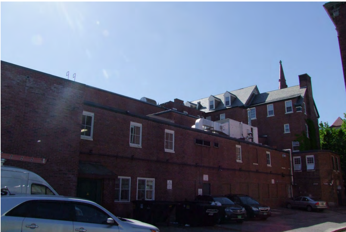
Photograph 16: North and west elevations of the building. Note the replacement windows on the west façade of the gymnasium wing, which are not compatible with the Colonial Revival style of the historic building.
