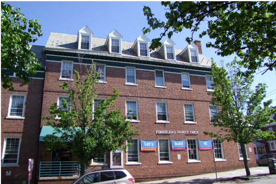
Photograph 2: South elevation of YMCA building
