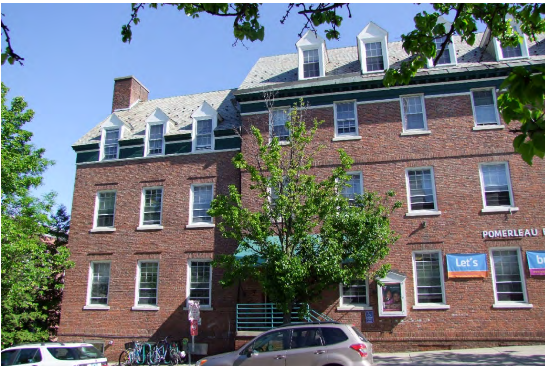
Photograph 4: West wing of the main block of the building. The new hotel building addition will extend to the west (left) of this wing but will be set back from the main façade.
