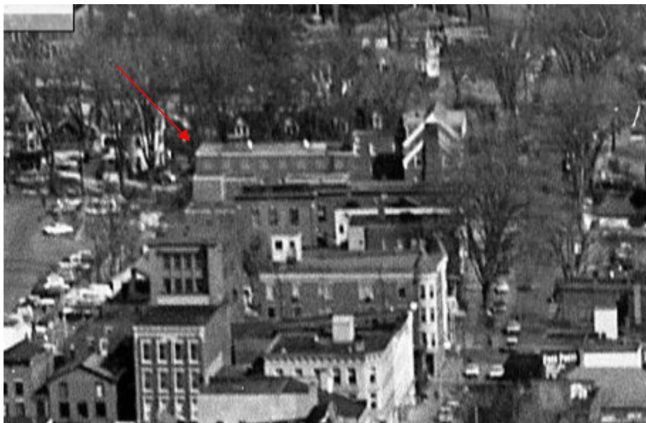
Figure 7: March 24, 1965 aerial photograph depicting the YMCA building with the gymnasium windows infilled with brick (see arrow). Image courtesy of UVM Special Collections via UVM Landscape Change Program (#LS37426).
