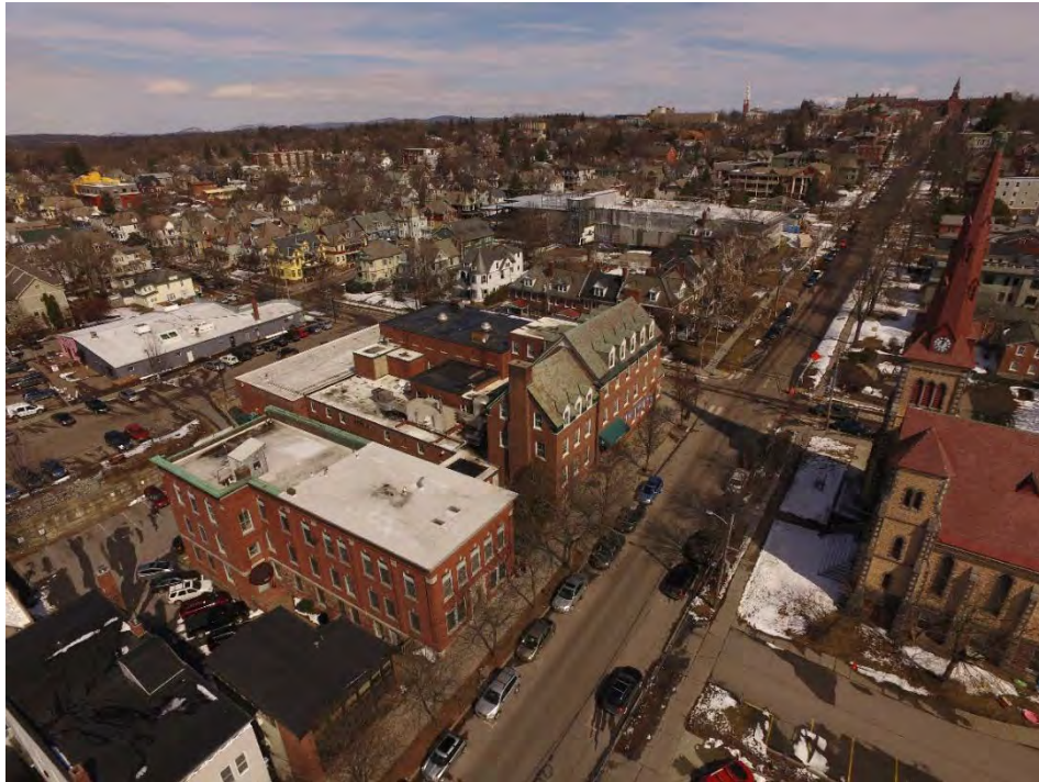
Photograph 43: Bird's eye view of the YMCA building, looking east-northeast. The multiple stories and additions on the north gymnasium and pool additions of the building are clearly visible from this location, as is the neighborhood context.
