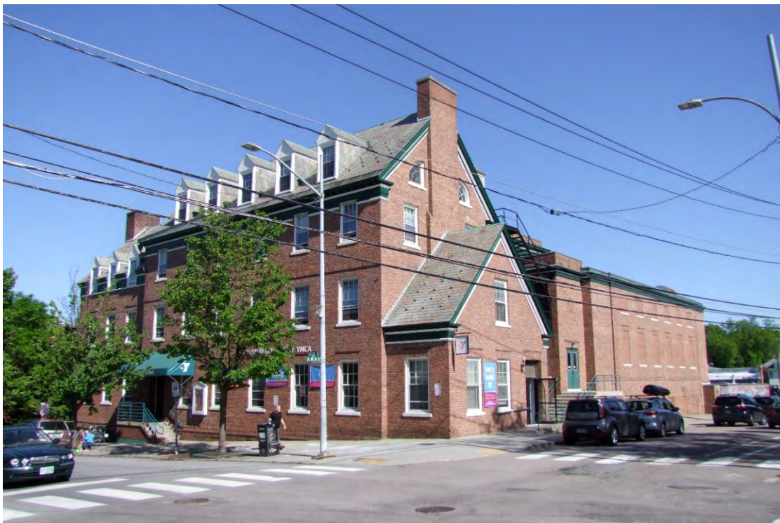
Photograph 8: South and east elevations of the YMCA building.
