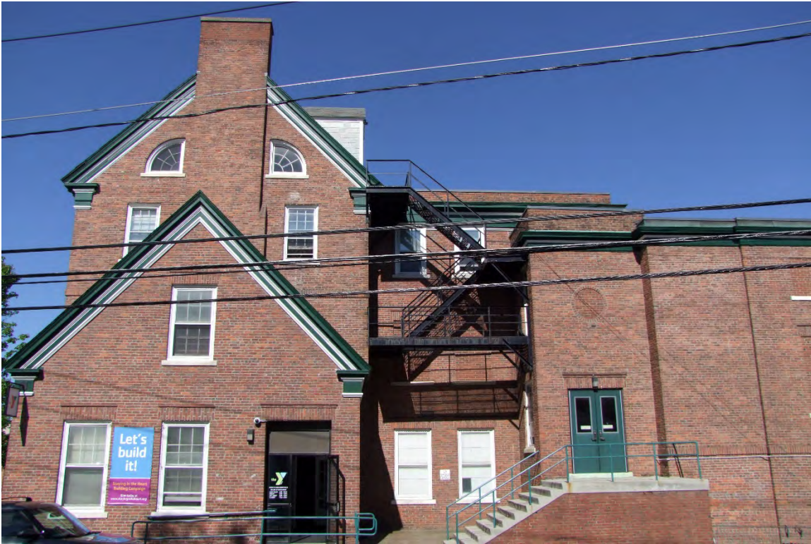
Photograph 9: East elevation of YMCA building. The gabled wing at left will be remodeled to serve as the primary entrance. The quarter fan lights will be preserved. One bay of the hyphen (at center) will be preserved to connect the historic building to the new hotel addition, which will replace the existing gymnasium at right. The fire escape will be removed.
