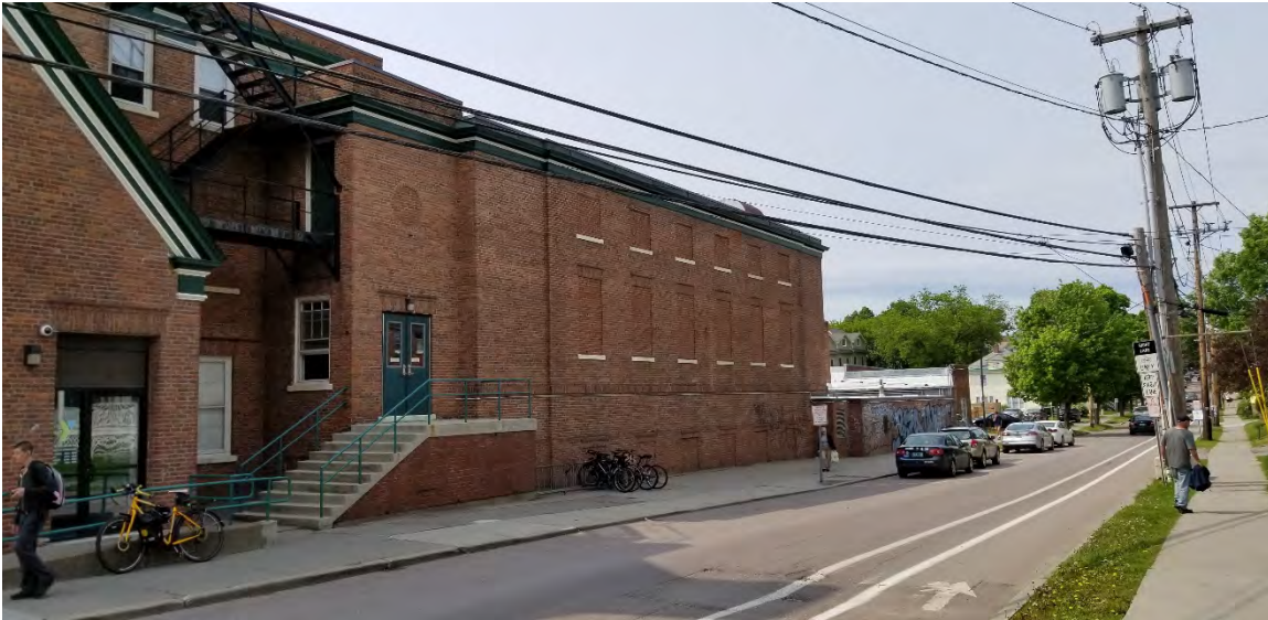
Photograph 11: East elevation of the 1934 gymnasium and pool wing along S. Union Street. The windows were infilled with brick sometime before the mid-1970s. This addition is proposed to be removed and replaced with the new hotel building.
