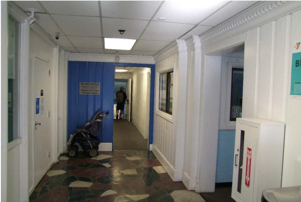
Photograph 25: Interior of the main hallway on the ground floor of the existing YMCA building's south block. The interior will be completely remodeled for the hotel.
