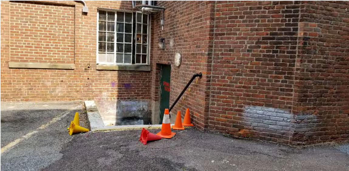
Photograph 19: Detail of existing boiler room entrance on the west elevation. Note the one remaining, historic, multi-light casement window; most of these were removed at some point and the openings infilled with brick.
