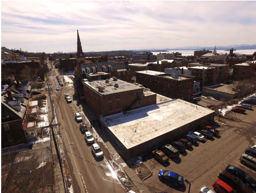
Photograph 41: Birds-eye view of the existing YMCA building, looking southwest. The two wings – the 1934 central wing and the 1984 north wing – are clearly visible. This photo displays the existing building within its neighborhood context.
