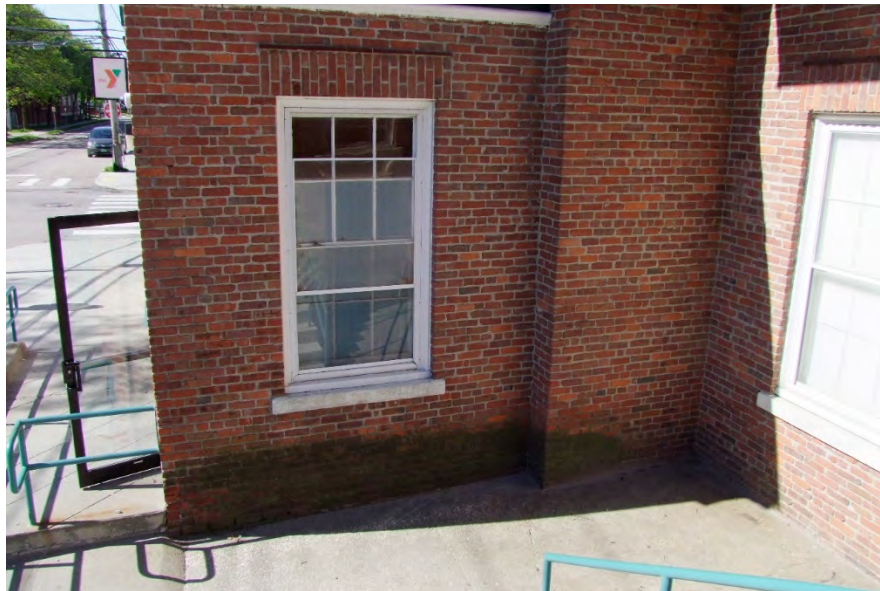
Photograph 10: North elevation of gabled east entrance wing. This wing will be retained, but it will be remodeled with new siding applied over the brick. The masonry will be repaired and repointed as needed following the Secretary of the Interior's Standards for the Treatment of Historic Properties.
