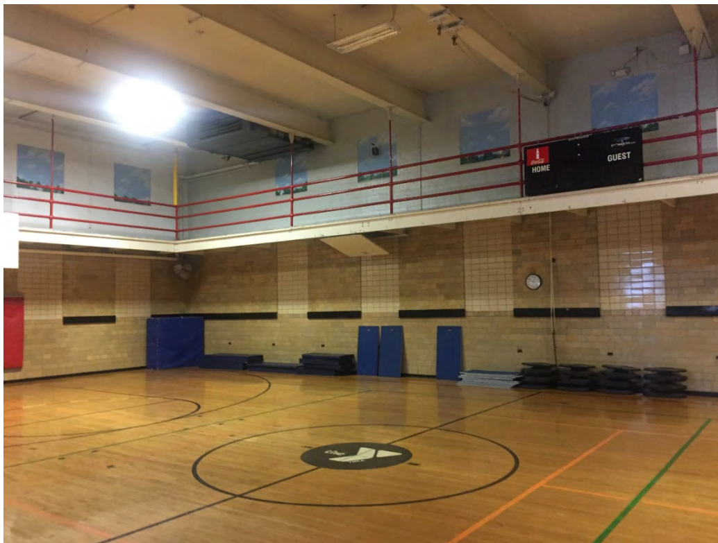
Photograph 32: Interior of existing, 1934 gymnasium wing proposed to be replaced by the new hotel building. Note the contrasting tiles and painted concrete located in the former window openings.
