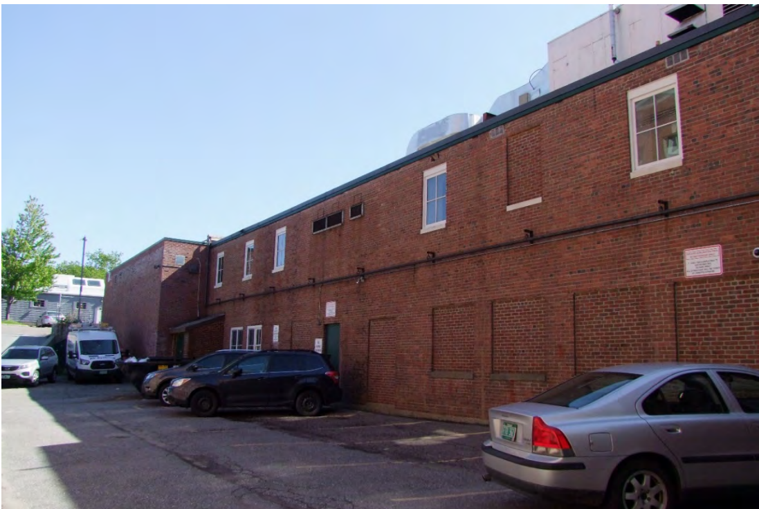
Photograph 18: Detail of altered west elevation of the gymnasium addition. Note the infilled windows and replacement windows. The new building will extend further west in the location of the existing parking spaces.
