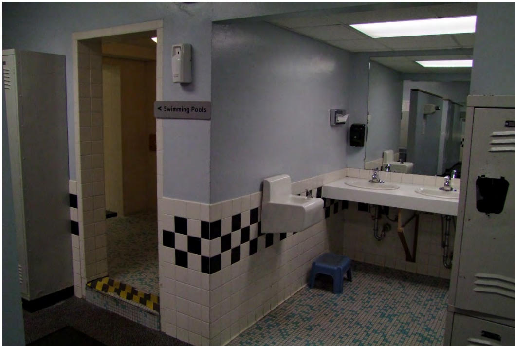
Photograph 35: Interior of the women's locker room of the 1934 pool/ gymnasium wing to be removed. The locker room appears to be in its historic location and features some historic finishes.
