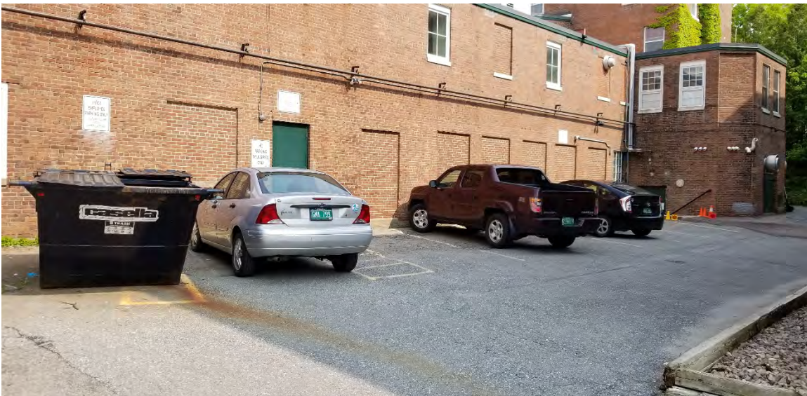
Photograph 20: Additional view of the west elevation of the gymnasium addition. The parking spaces mark the approximate edge of the proposed new building. The small wing at far right will also be removed and replaced with the new building.
