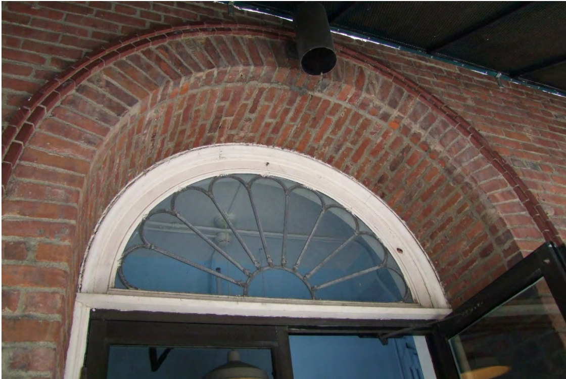
Photograph 5: Existing fanlight above main entrance of south elevation; this will be preserved and will be more visible once the awning is removed and replaced with a higher canopy.
