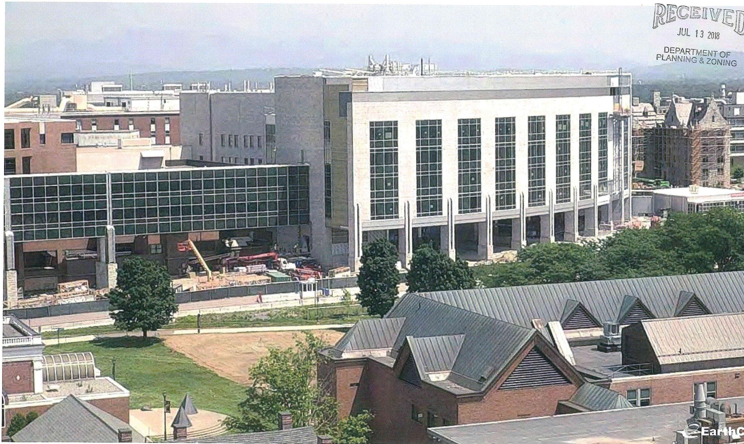
UVM Medical Center - RH Miller Building Under Construction with Temporary Emergency Department, July 2018
