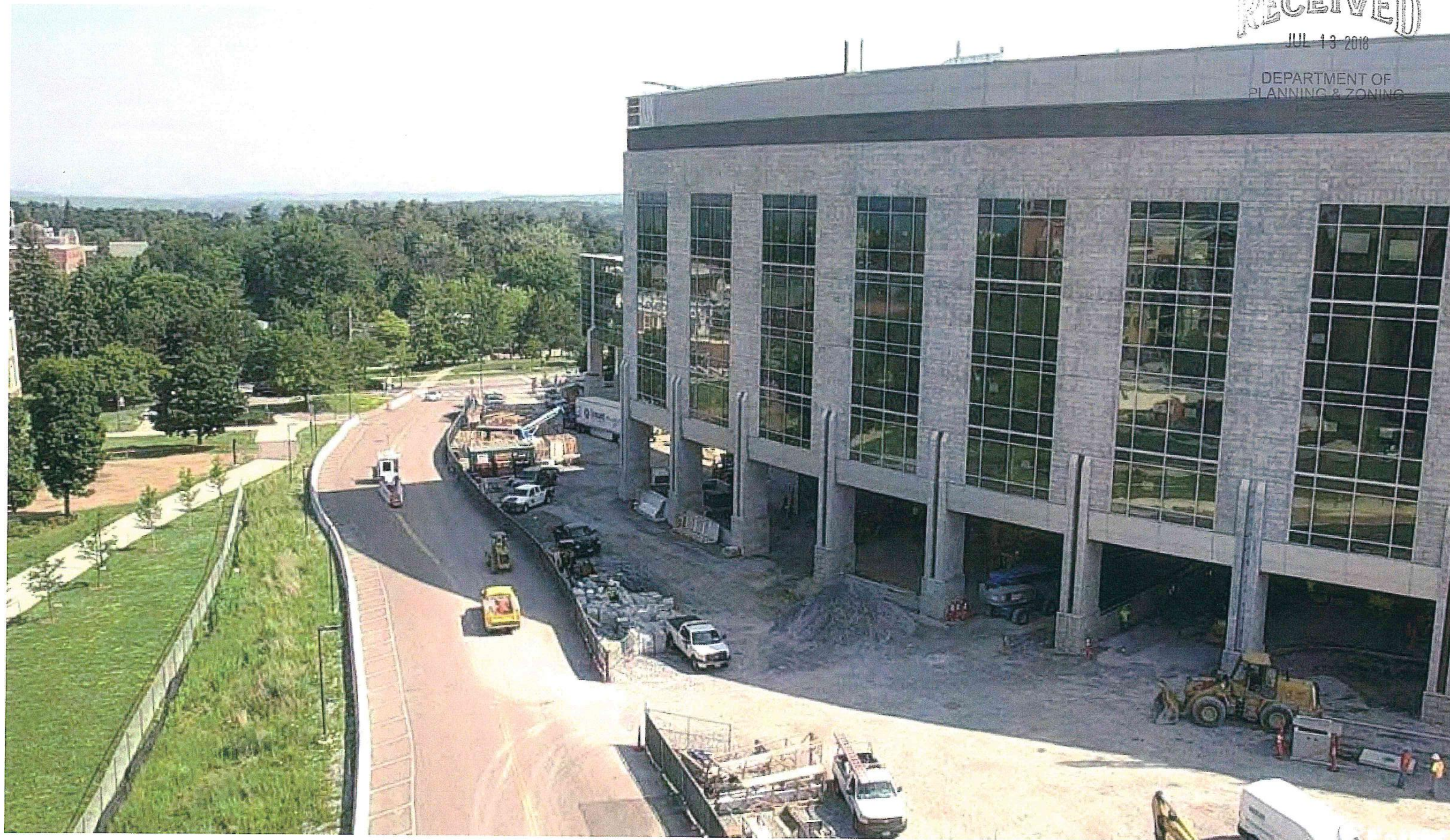
UVM Medical Center - RH Miller Building Under Construction, Hospital Drive Temporary Location, July 2018
