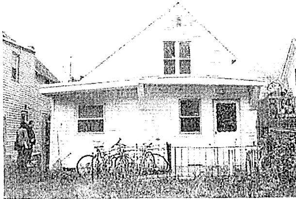
Rear elevation, showing non-historic rear addition.
