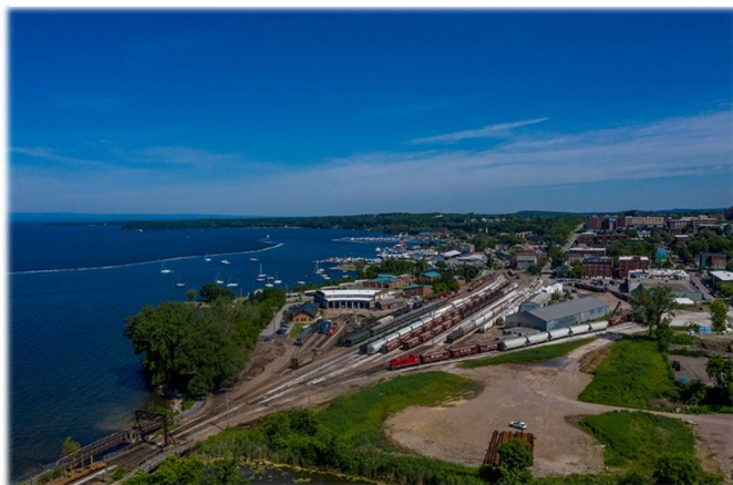
Figure 1: 2019 Aerial View of Existing Burlington, VT Railyard
