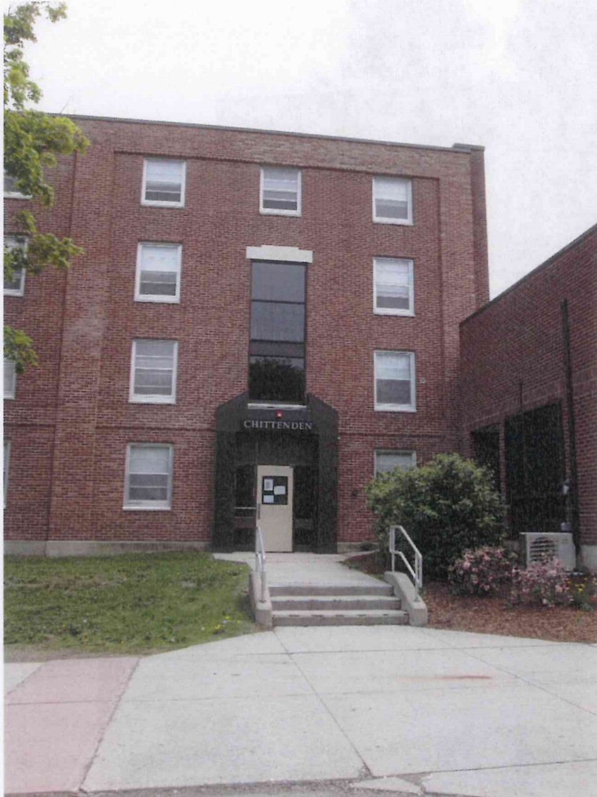
Chittenden, South Entry on West Façade
