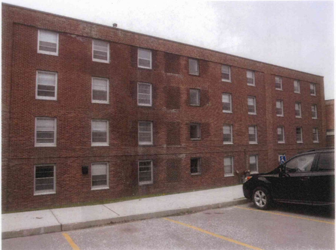
Buckham, East Façade
