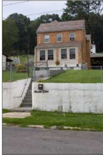
Examples of retaining walls used to provide flat areas for houses.
