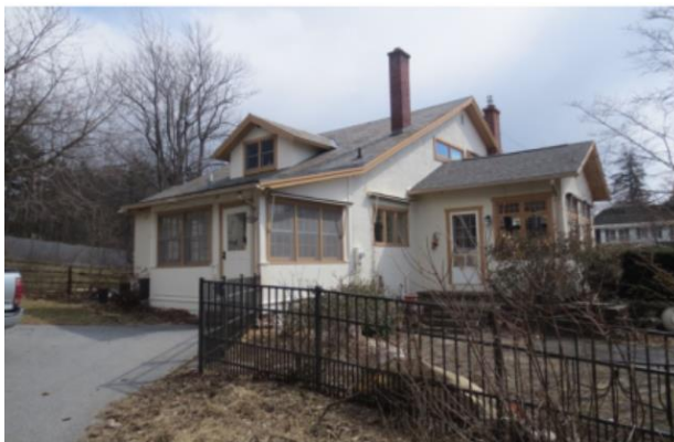
AREA OF RENOVATION
