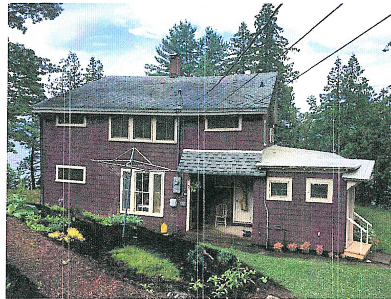
EXISTING HOUSE FROM EAST
