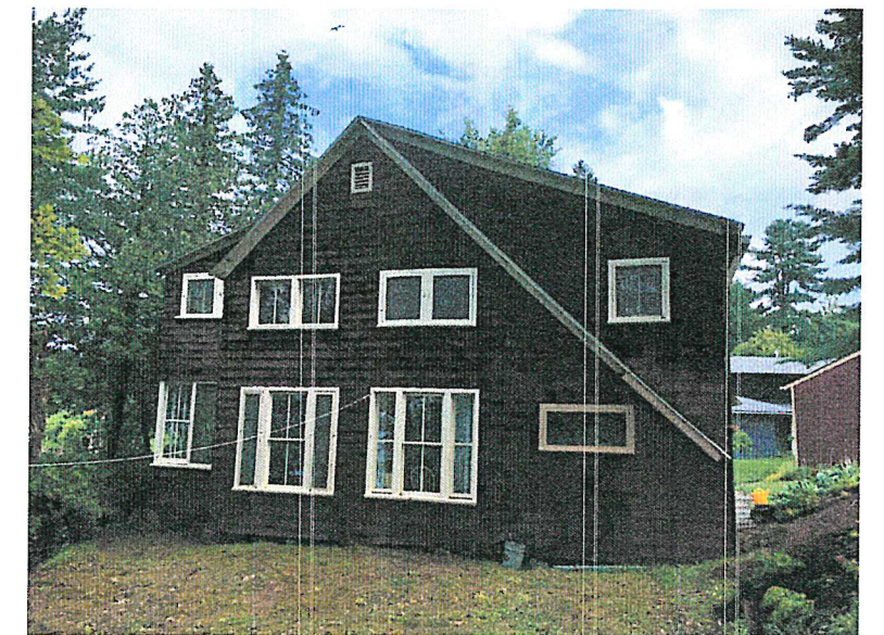
EXISTING HOUSE FROM SOUTH
