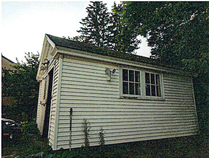
Figure 2: Current garage roof is asphalt shingle, siding is vinyl.
