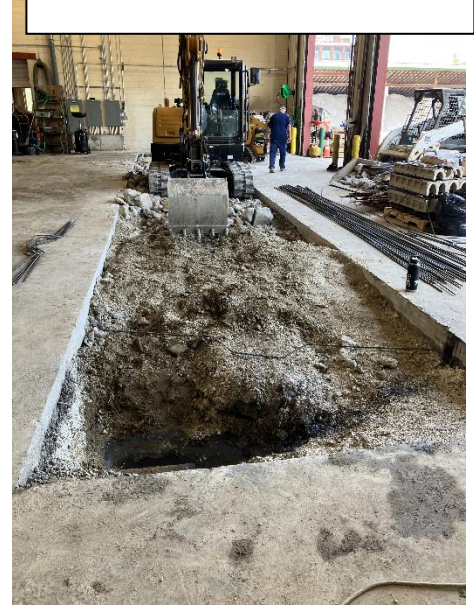
645 Pine drain installation
